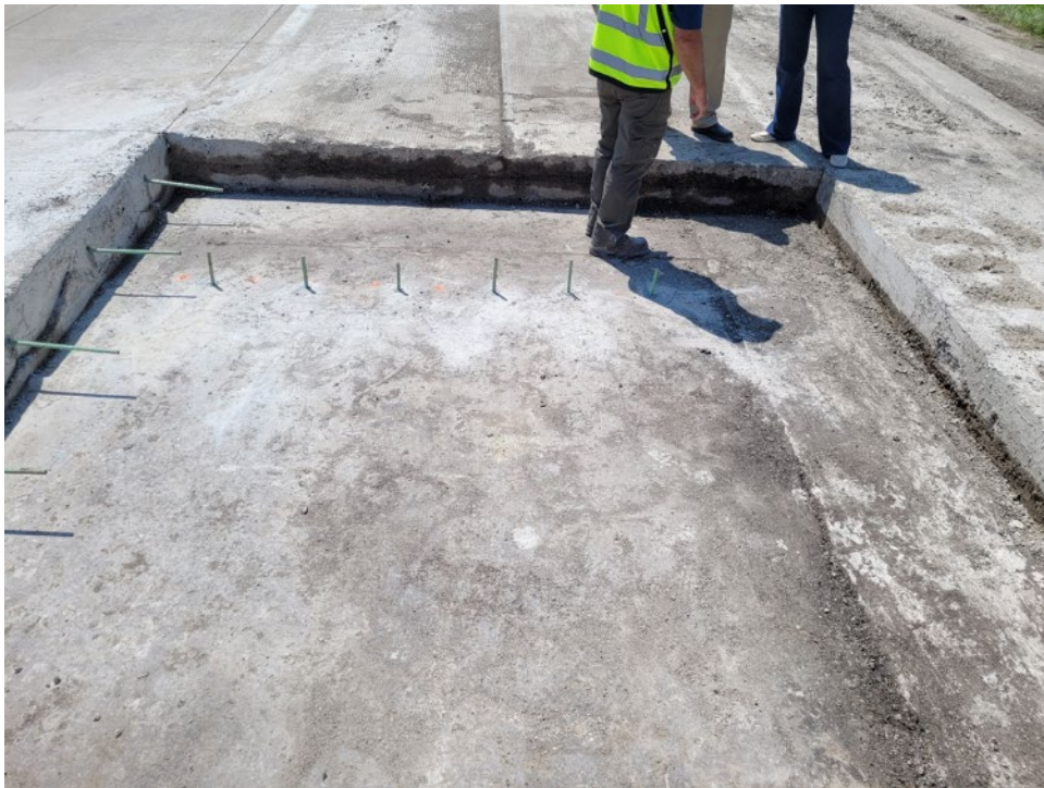
Figure 52 – Patch, existing original pavement left in place and pins.
