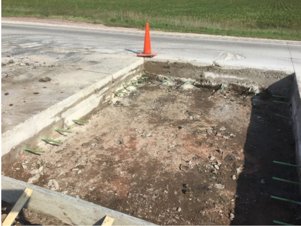
Figure 51 – Full depth PCC patch in overlay
