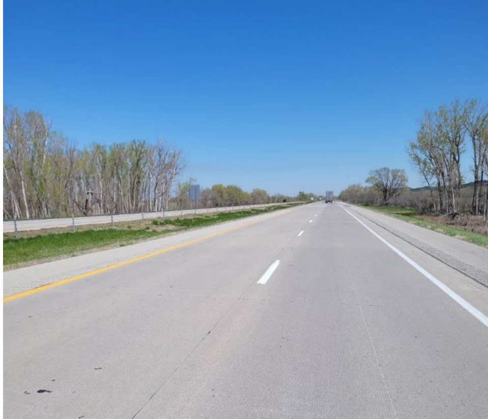
Figure 29 – Mills County I-29 NB Unbonded Overlay (2023)
