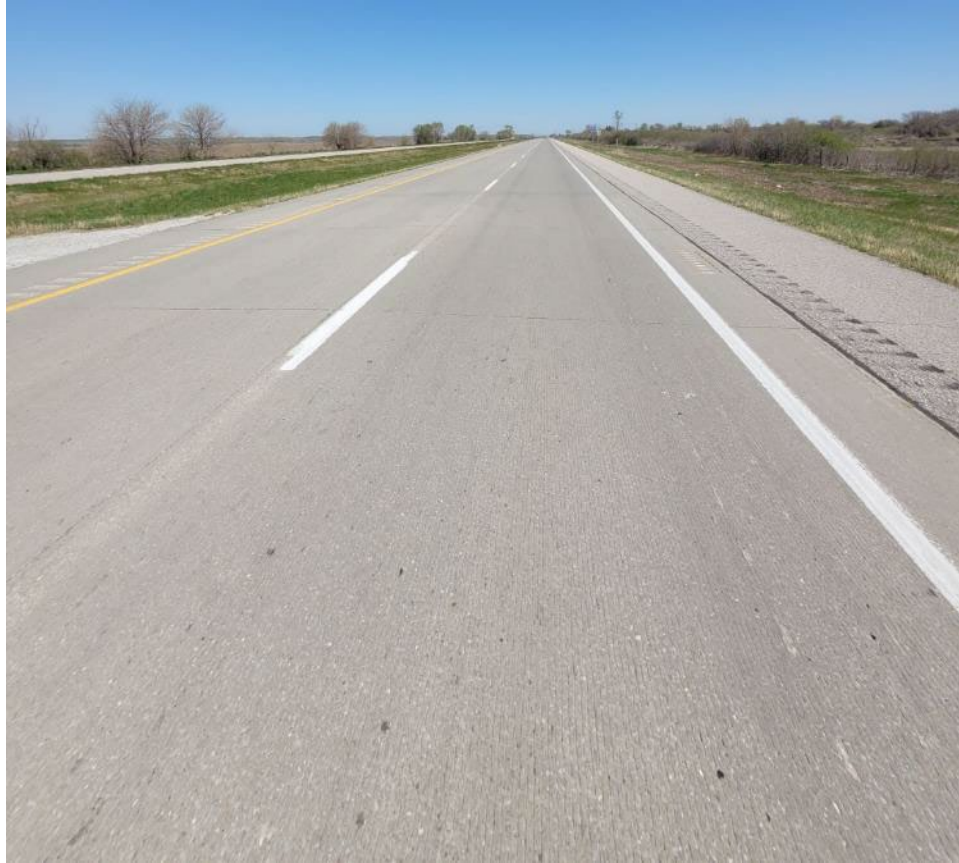
Figure 28 – Fremont County I-29 NB Unbonded Overlay (2023)
