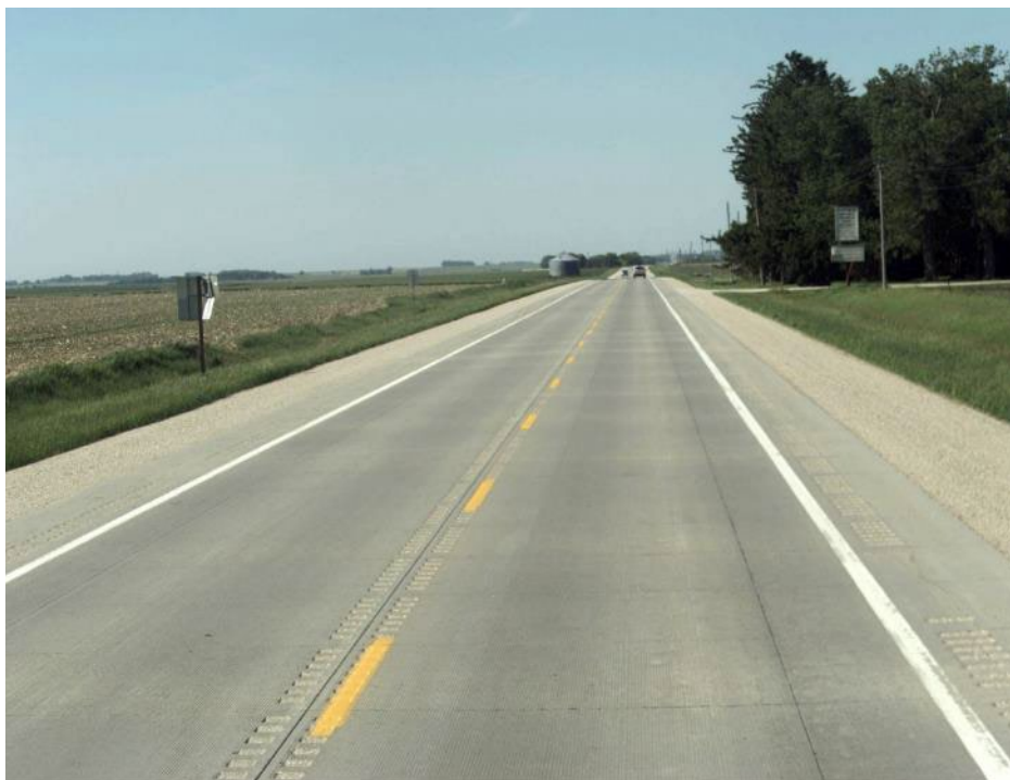
Unbonded overlay section
