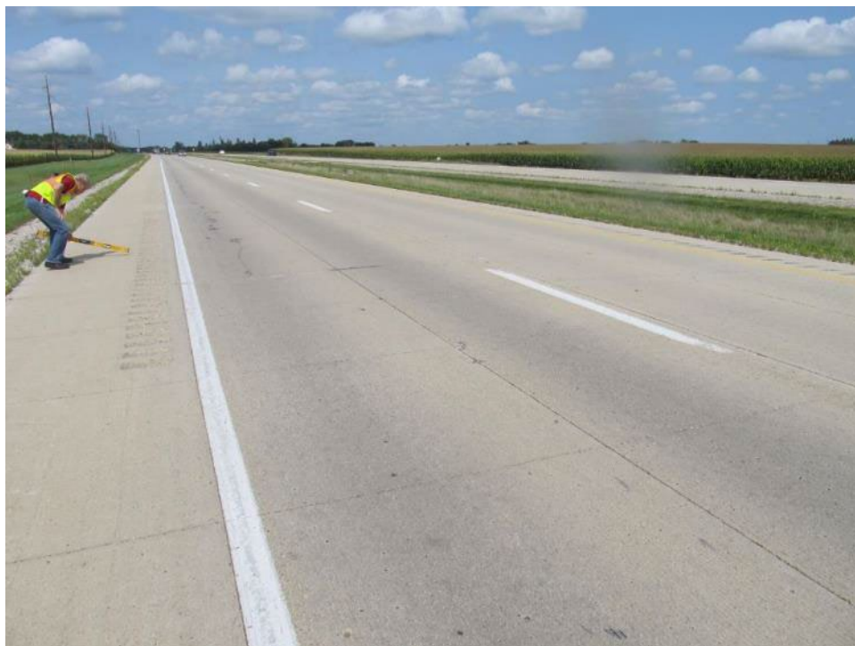
Shoulder cross slope 3.3%, Design 4%.
