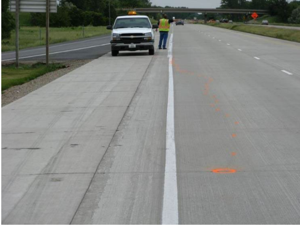
Section 2 Cross stitching 9242 feet right, 3763 feet left.
