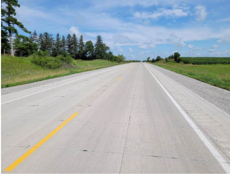
Figure 48 – Tama/Blackhawk US 63 Overlay with 5 lbs. macro fiber per cubic yard.
