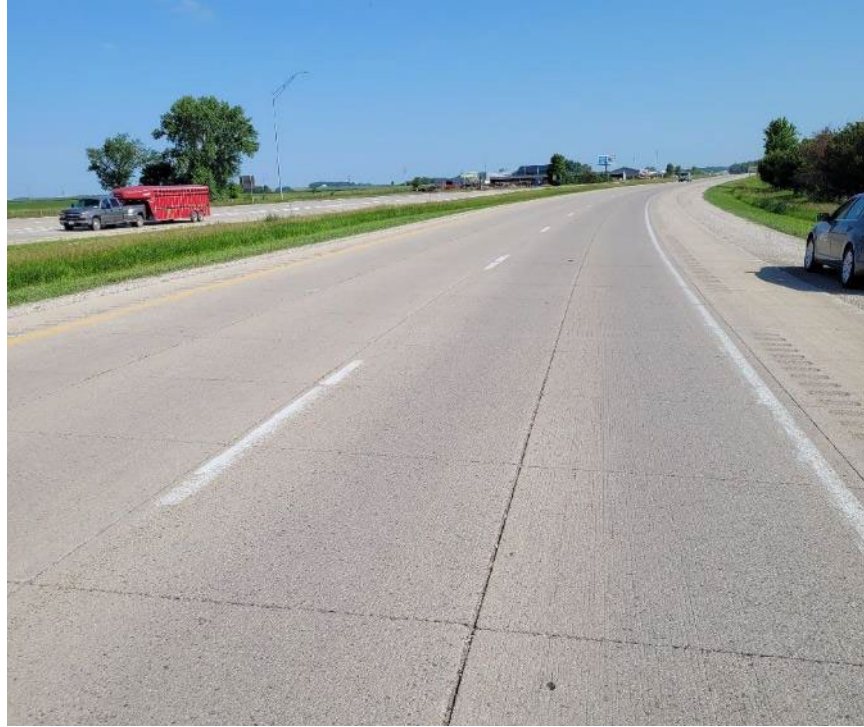
Figure 16 – Clay/Dickinson US 71 Whitetopping Overlay Built 2012 (Picture 2023)
