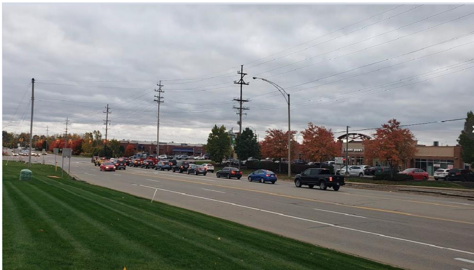
Figure 4-12. Section of E Beltline Ave SE lacking pedestrian crossings
