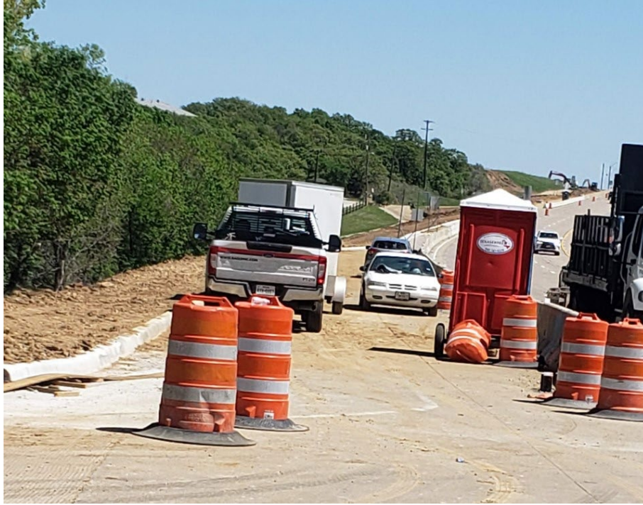
Figure 42. Photo. Site photo of the identified work zone sites on US-380.
