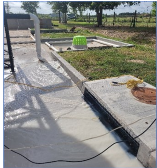
Figure 1. Drop Inlets and Curb/Gutter Application.
