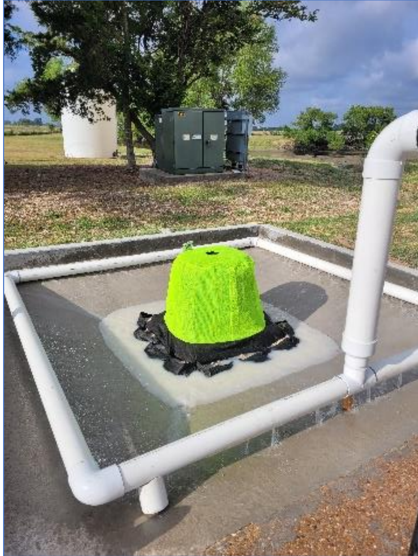
Figure 7. Concrete Drop Inlet Evaluation Test System.
