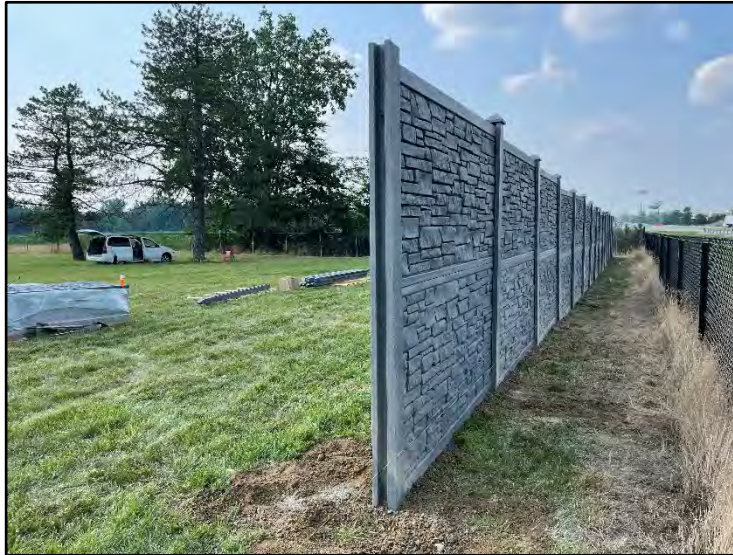
(21) First 14 panels looking North, east face of wall
