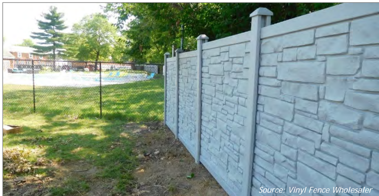
Figure 2.6: Photos of the Bexley, Ohio Vinyl Fence Noise Wall
