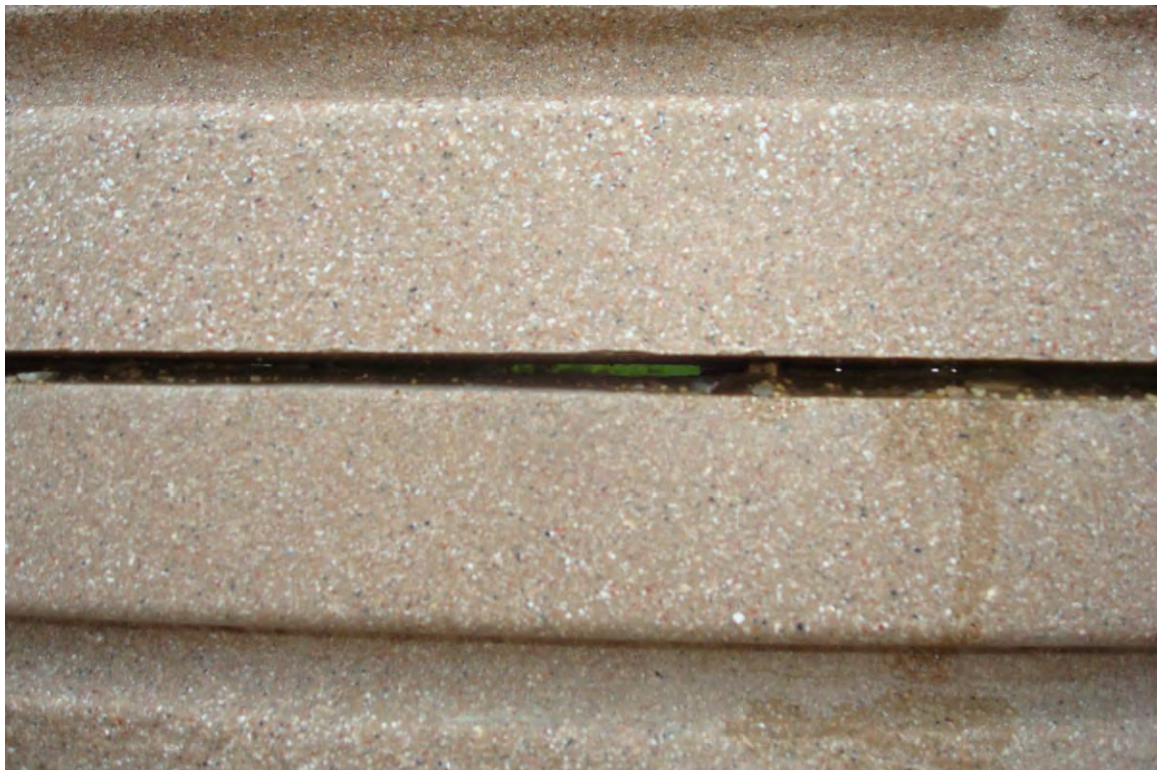
Bigger gap between two of the panels. Light very transparent thru panels.
