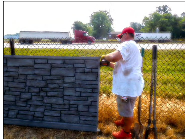
(10) Deburring of panel edges
