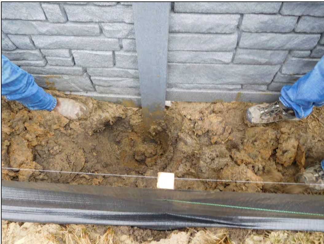
(24) Post 4 soil condition approx. 18" below surface
