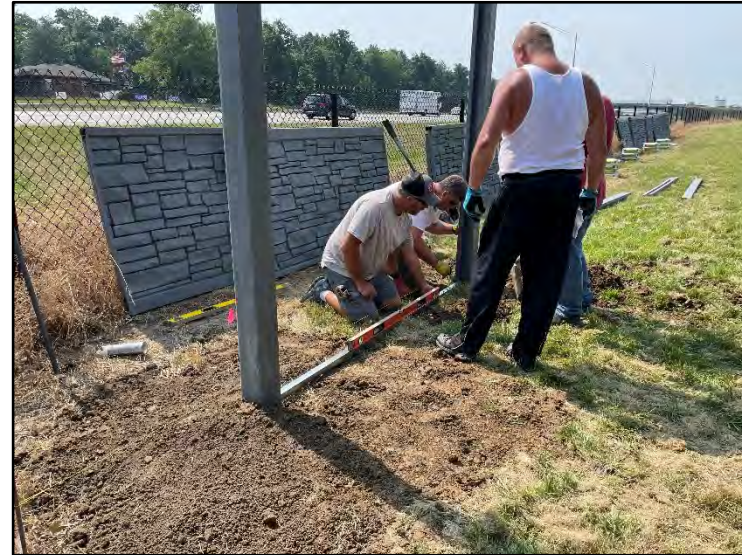
(14) Leveling panel bottom brace on brackets
