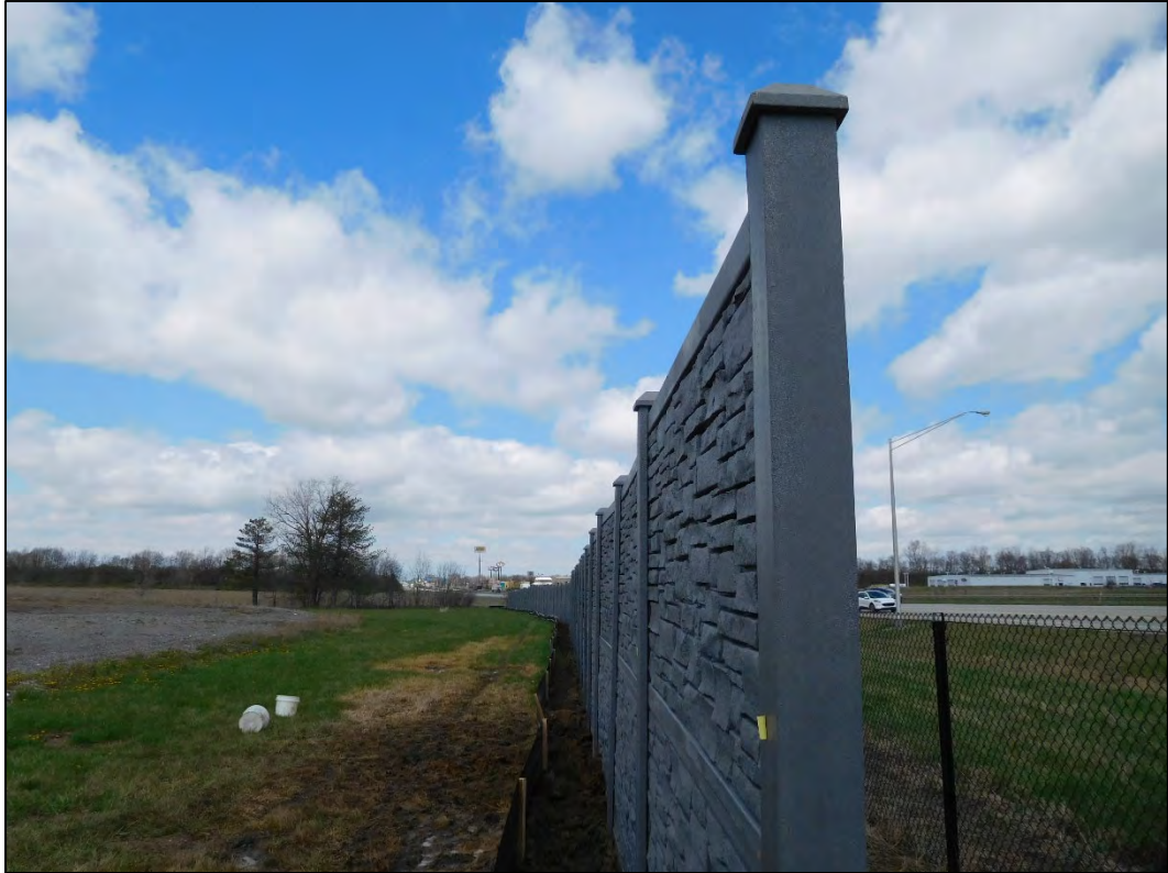
(33) West side of wall repair
