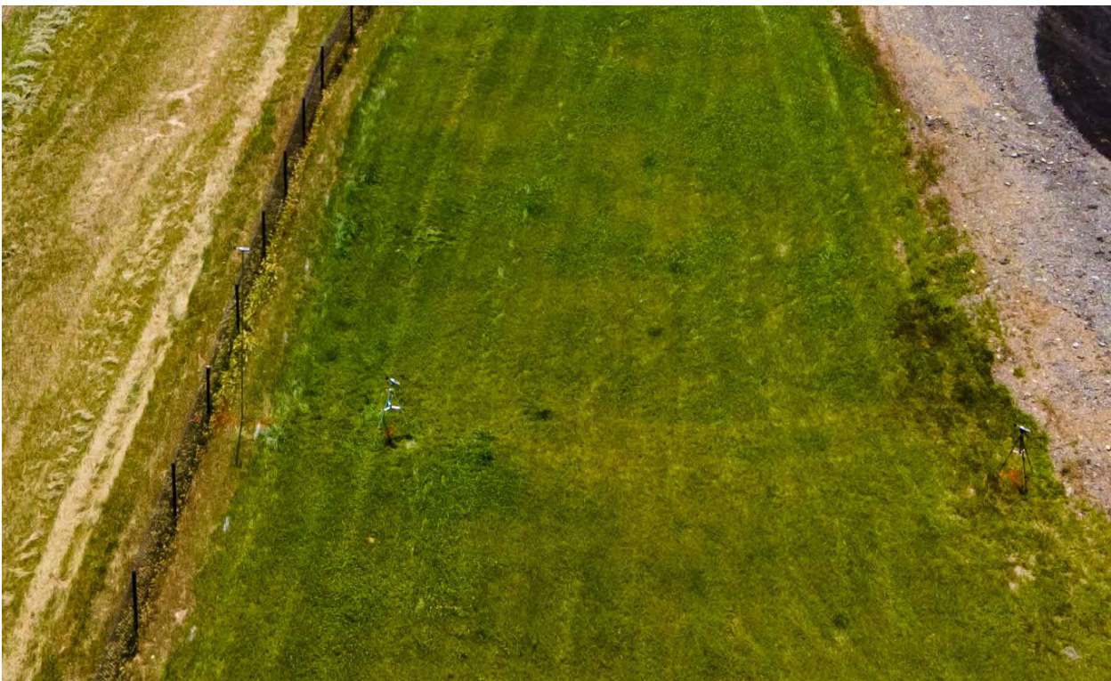
(06) Drone aerial image of Meters A, B, C, D, and E, at Lima, OH prior to vinyl wall construction
