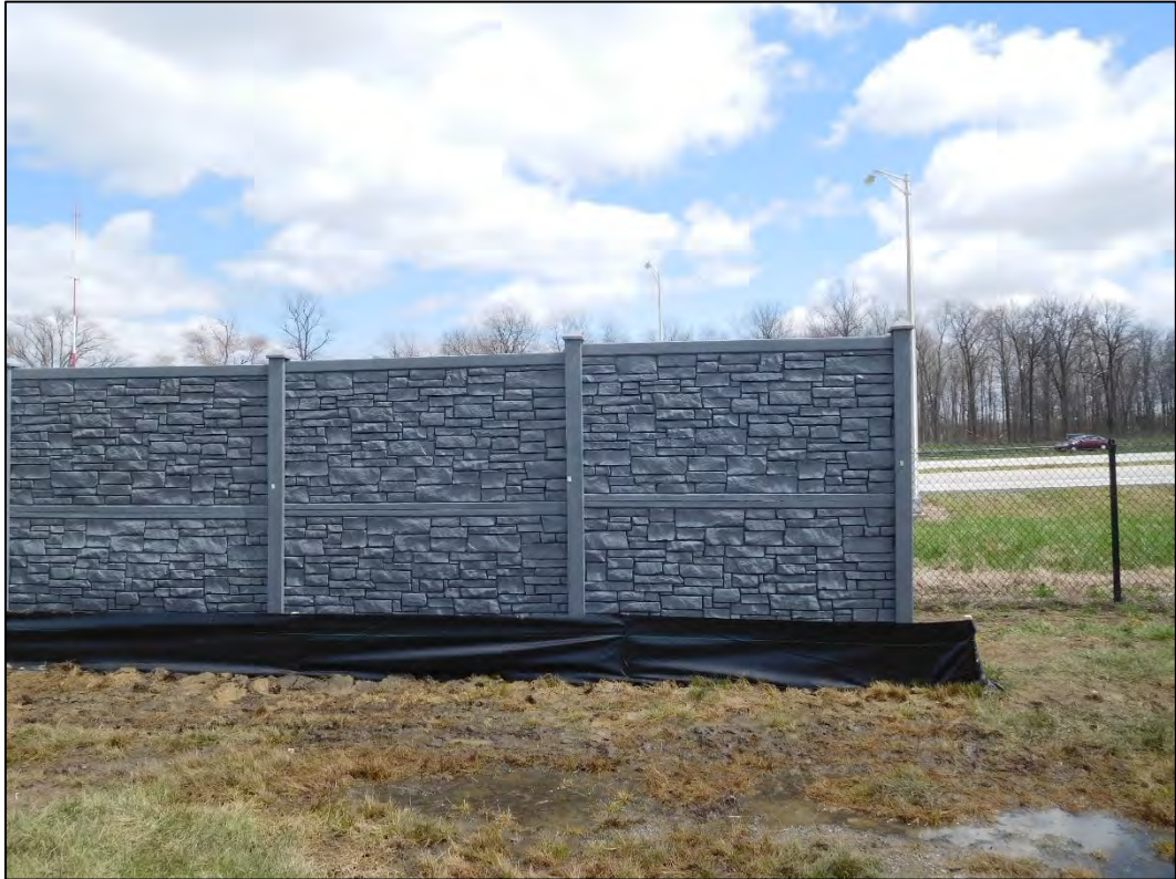
(34) View of repaired section west to east
