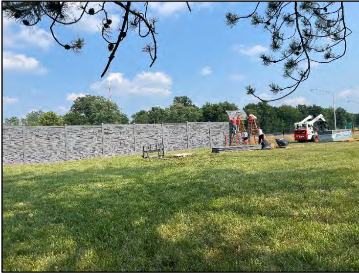
(17) Placing upper panel manually
