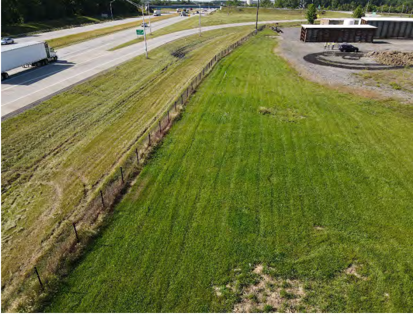
(01) Drone aerial image of Lima, OH prior to vinyl wall construction
