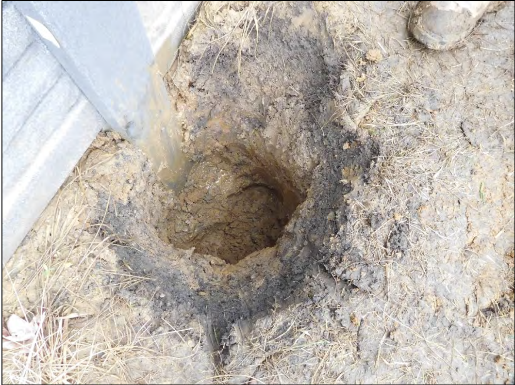
(25) Post 4 soil condition just above concrete footer
