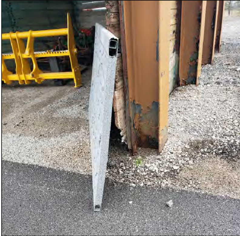
(05) New replacement panel
