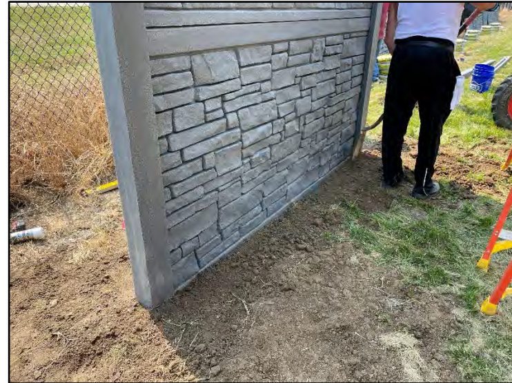
(16) Backfill to cover gap between lower panel and ground
