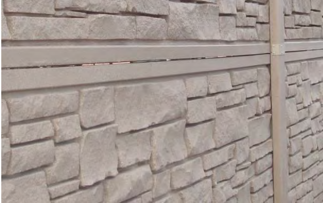
(2) Westside north wall
