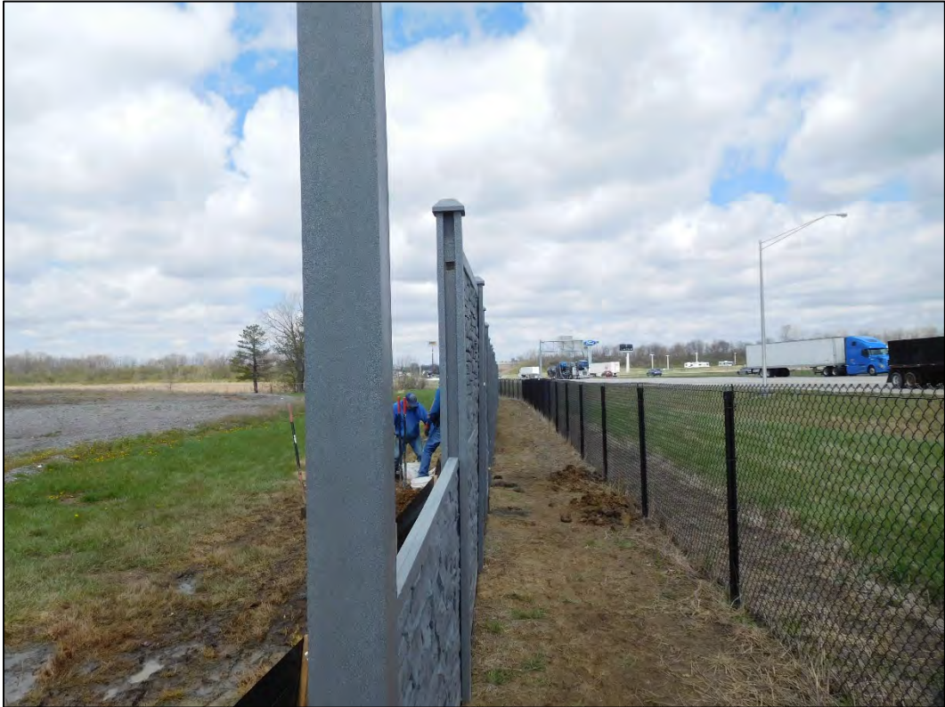
(30) Posts 3 & 4 after excavation and adjusting of posts
