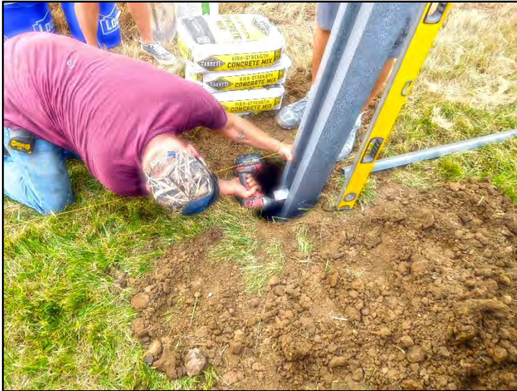
(13) Installation of lower panel support brackets
