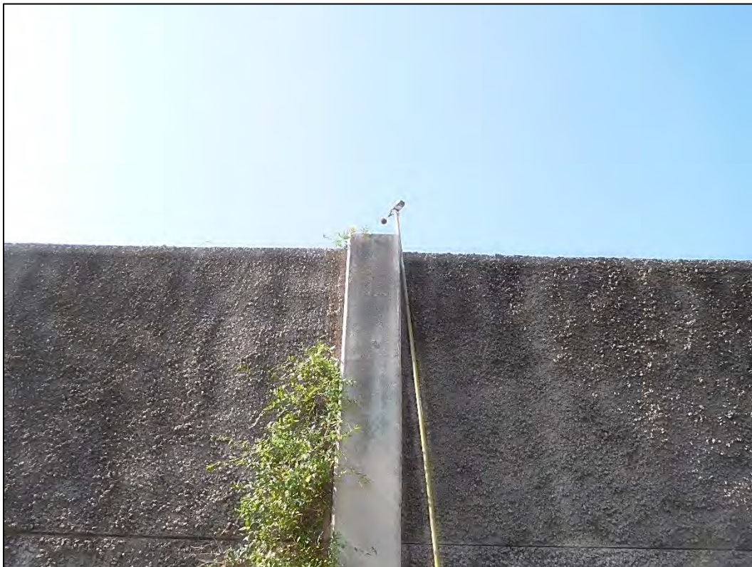
(34) Meter A in Richmond, VA at the concrete wall site
