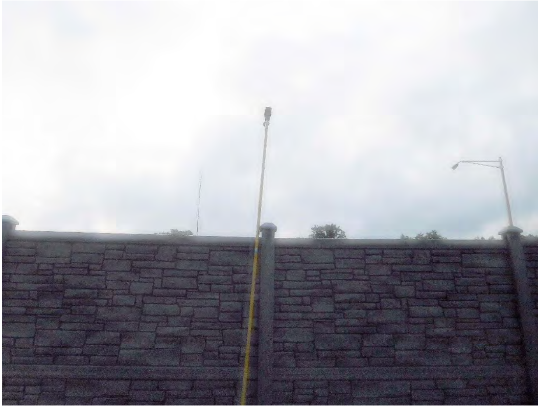
(07) Meter A (top of the wall) in Lima, OH after vinyl wall construction
