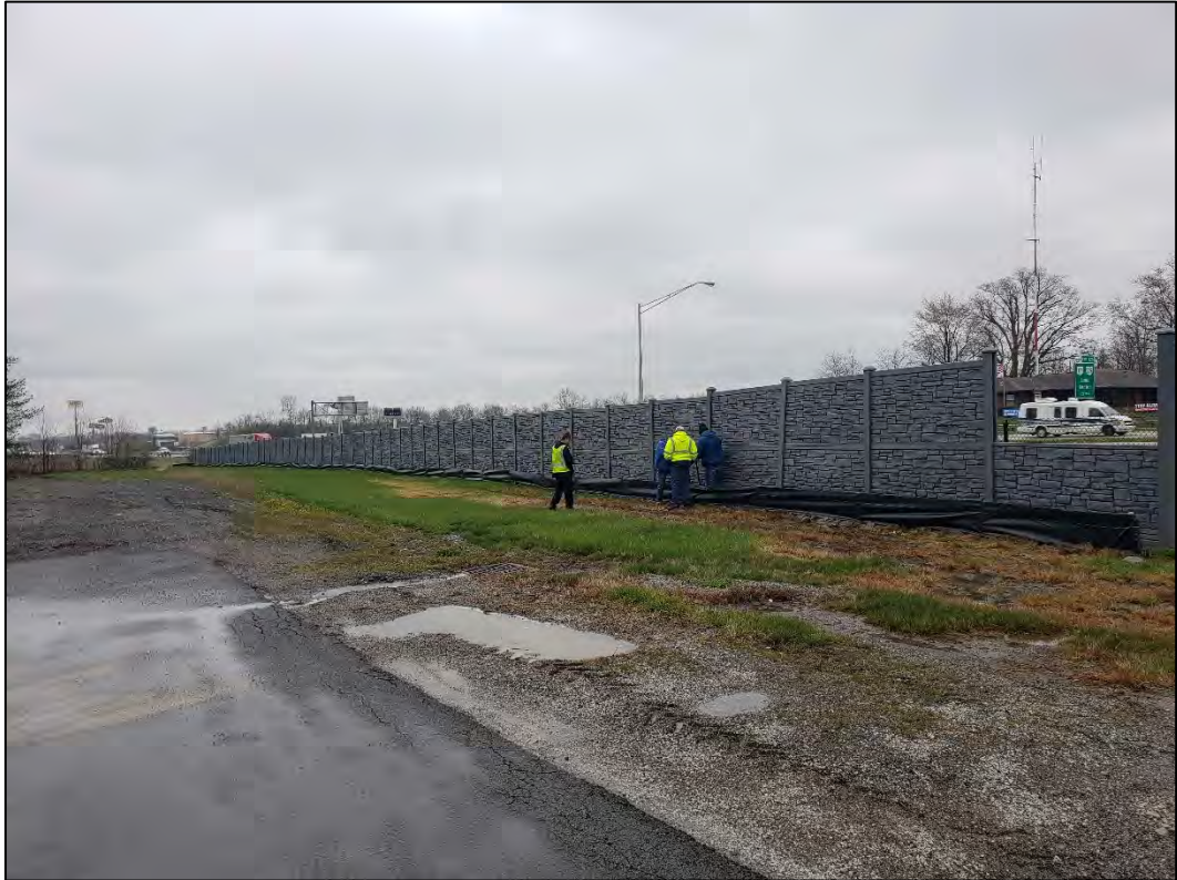
(22) General view of excavations and repairs
