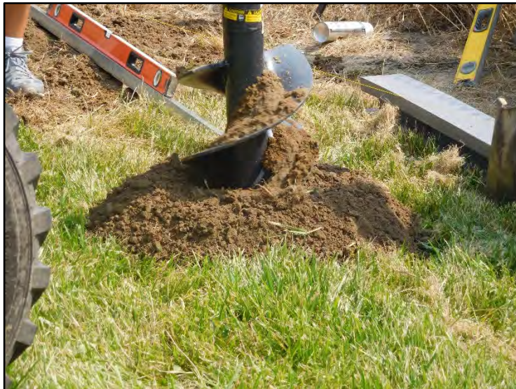
(11) Post hole drilling
