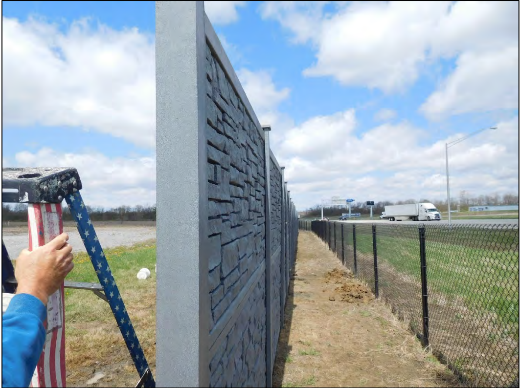
(31) after post adjustments and panel replacement
