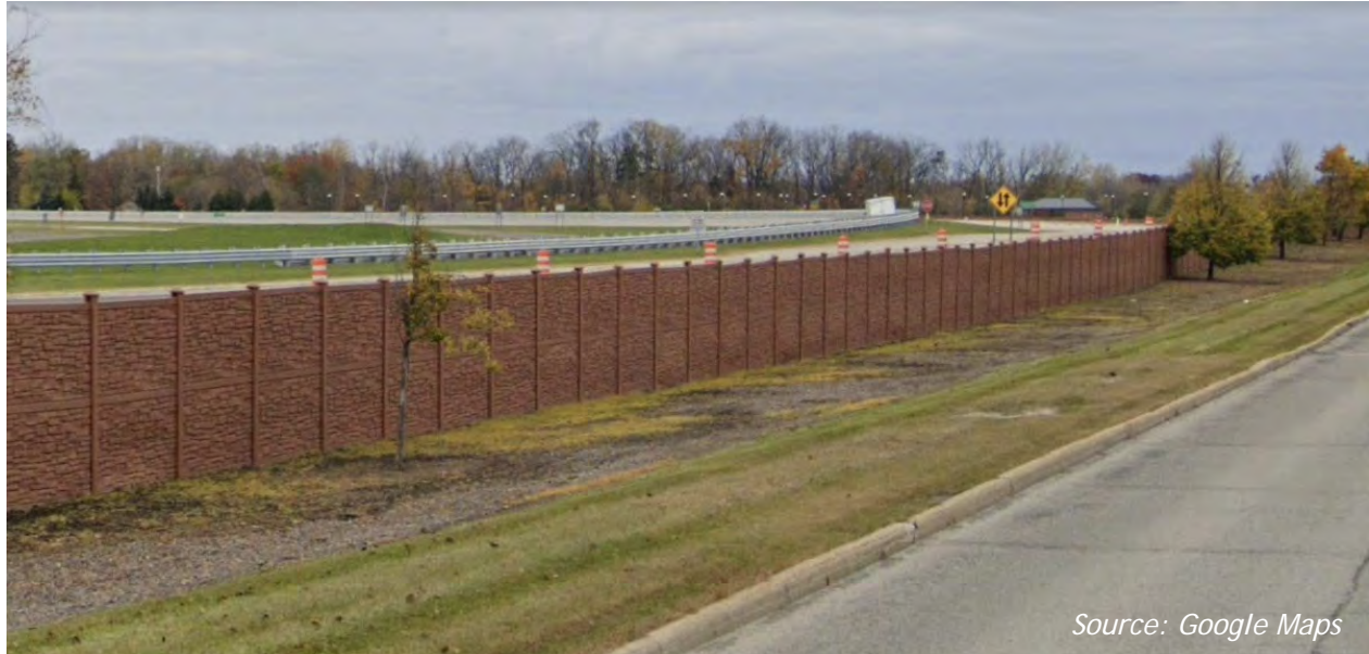
Figure 2.11: Michigan Vinyl Noise Walls, along Southfield Freeway
