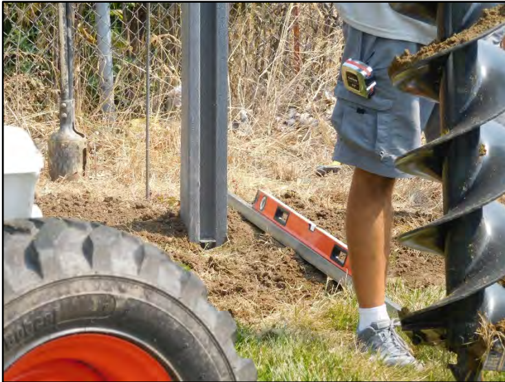
(15) First post installed showing panel support bracket
