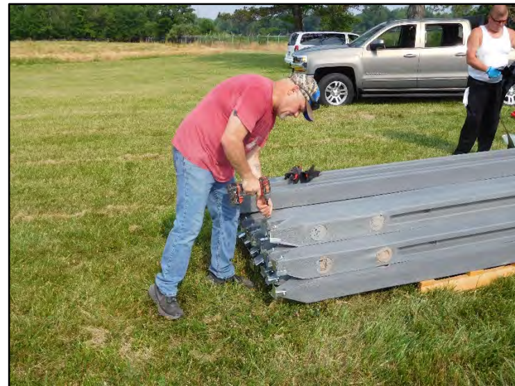
(08) Removal of panel support brackets
