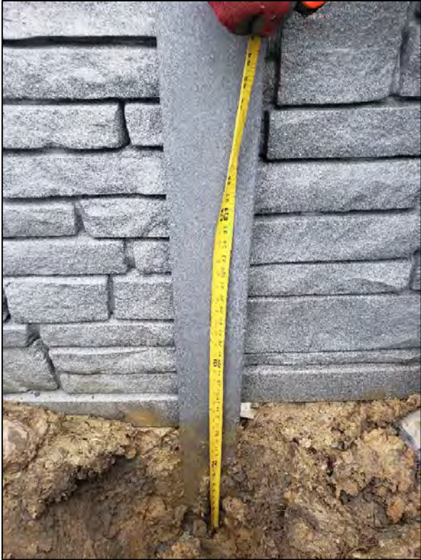
(27) Post 5 soil condition just above concrete footer
