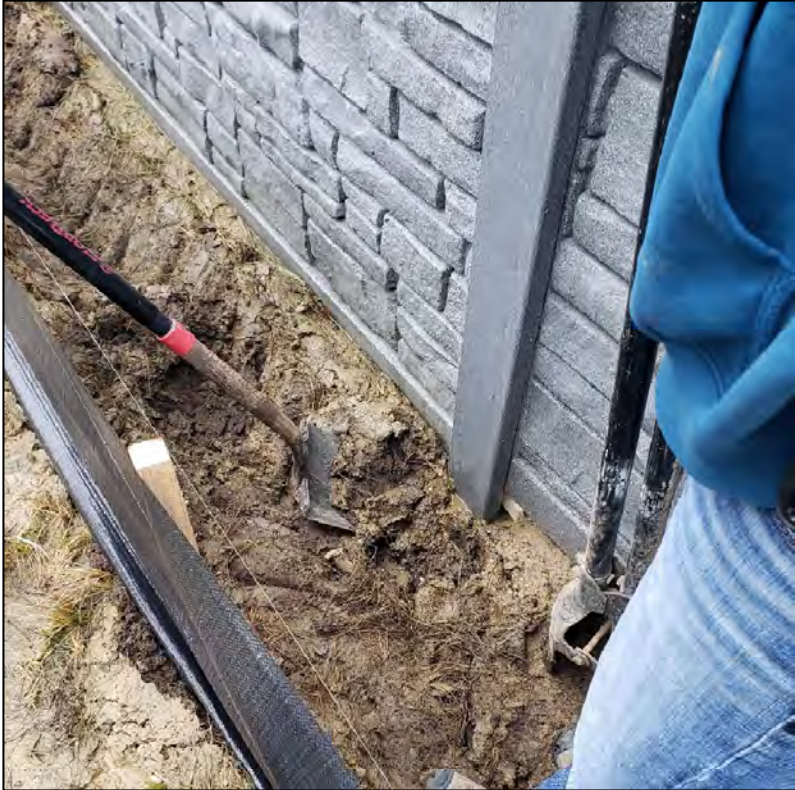
(21) Start of excavation at post 5
