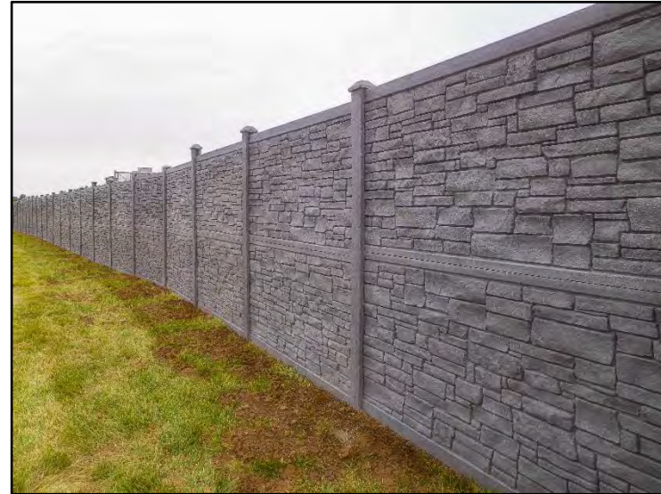
(22) Completed wall – west side looking North
