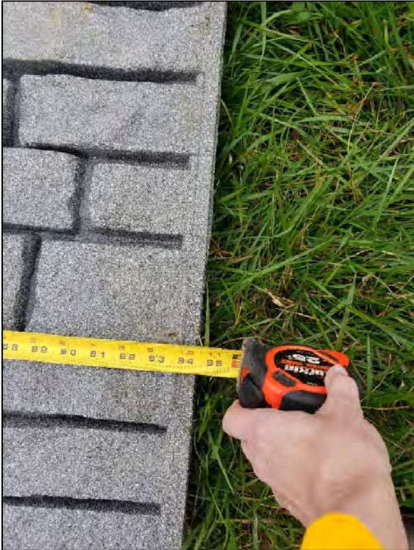
(08) Broken panel width
