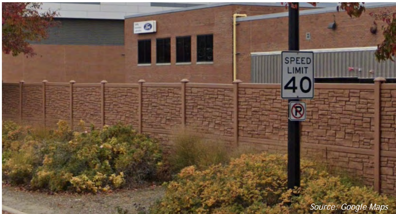
Figure 2.12: Michigan Vinyl Noise Walls, along Oakwood Boulevard
