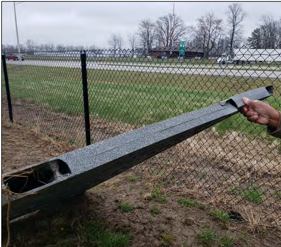
(02) Broken panel and damage to panel at bending point
