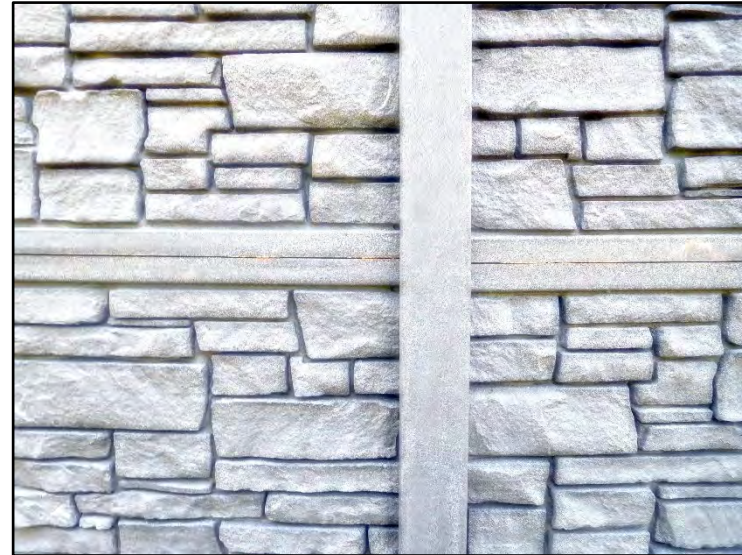
(20) Slight gaps. Some of these gaps closed after being in the heat of day
