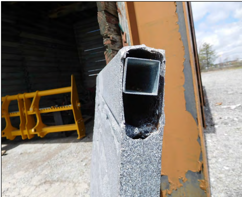
(06) Replacement panel with upper reinforcement beam in place
