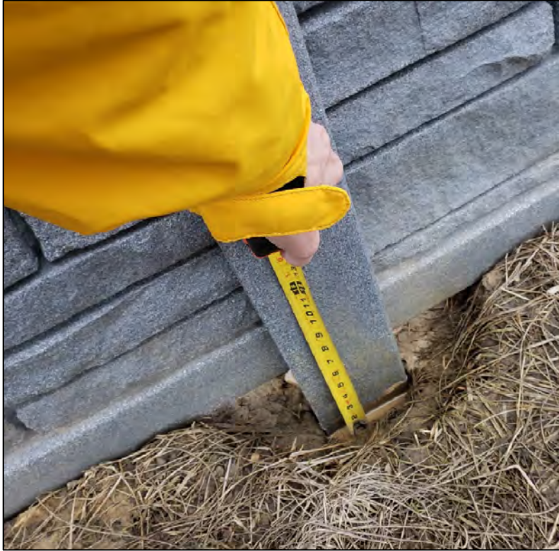
(23) Settlement at post with measurement
