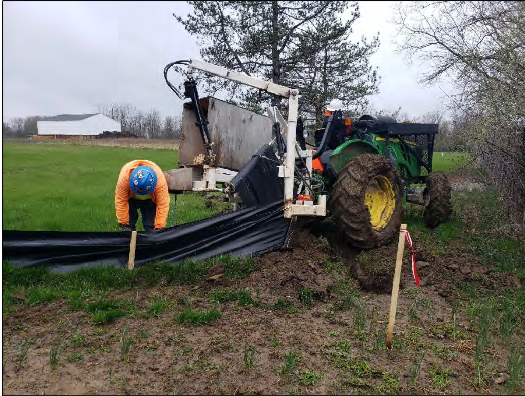
(19) Silt fencing being installed
