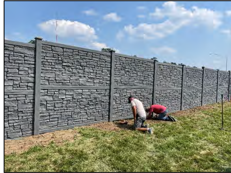
(18) Propped up panel and readjusting for post cap
