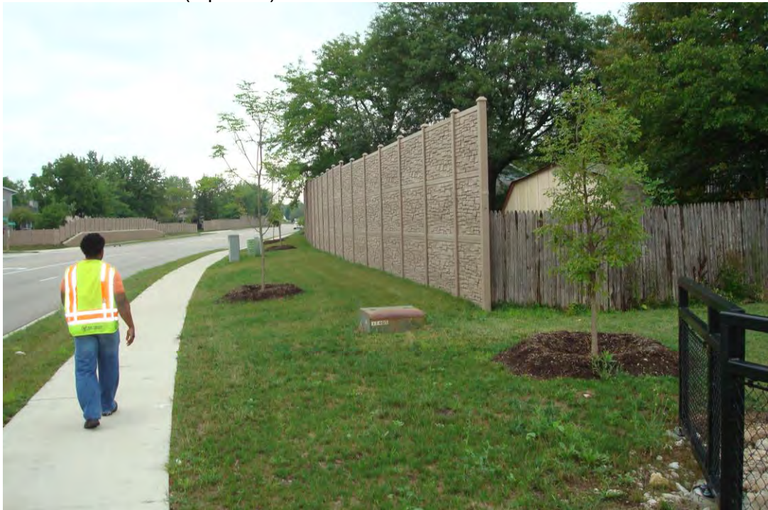
Eastside north wall (3 panels):
