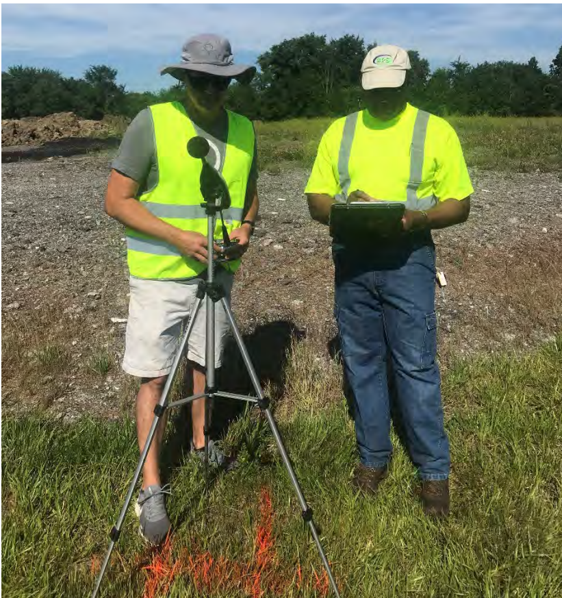
(02) BPS field work crew in Lima, OH prior to vinyl wall construction
