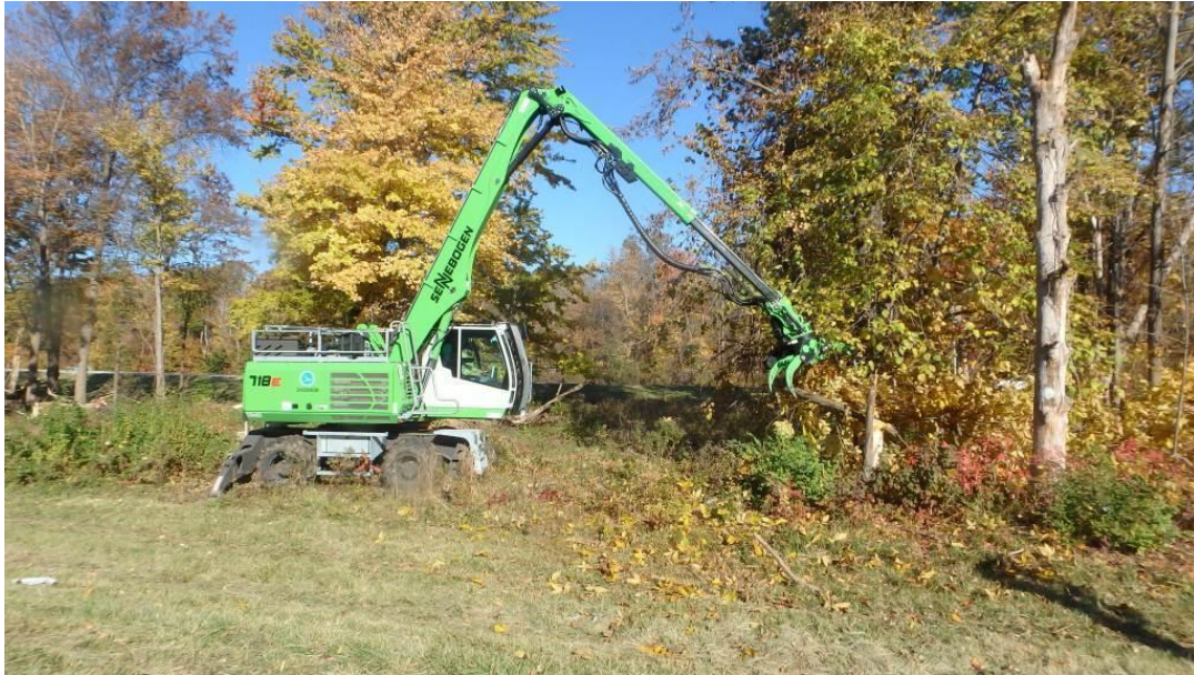
Photo 3: Sennebogen 718E being operated by ODOT in November 2021.
