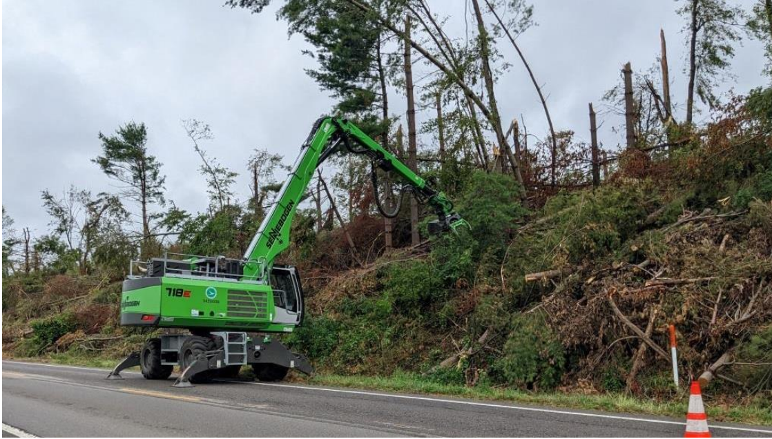
Photo 6: Sennebogen 718E moving piles of debris in July 2022 operations.
