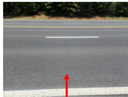
Example Current Condition Photo 2
