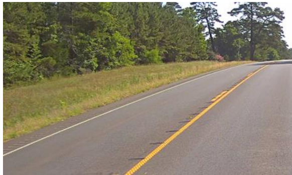
Example Current Condition Photo 1
