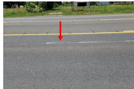
Example Current Condition Photo 2
