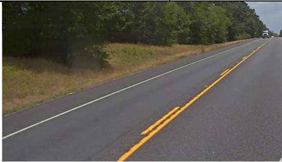
Example Current Condition Photo 1
