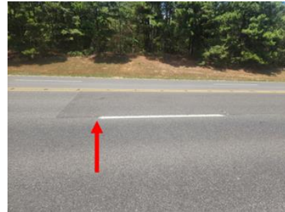
Example Current Condition Photo 2
