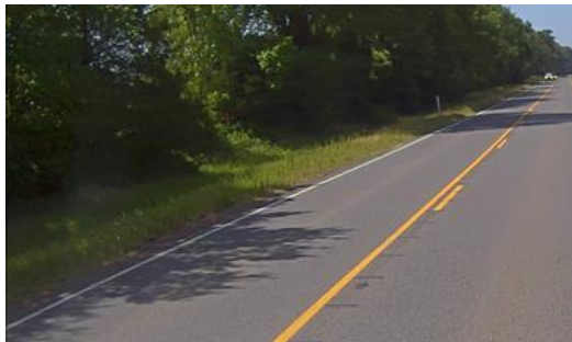
Example Current Condition Photo 1
