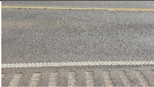
Example Current Condition Photo 1
