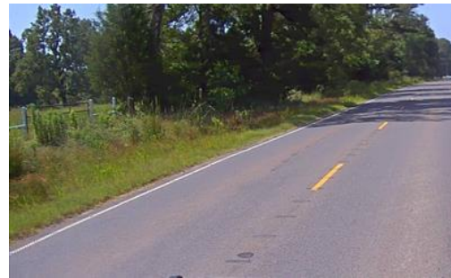
Example Current Condition Photo 2
