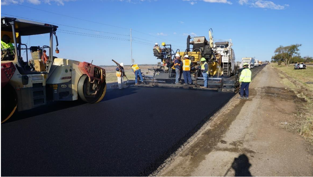
Figure 34. Paving Operation on US 287.
