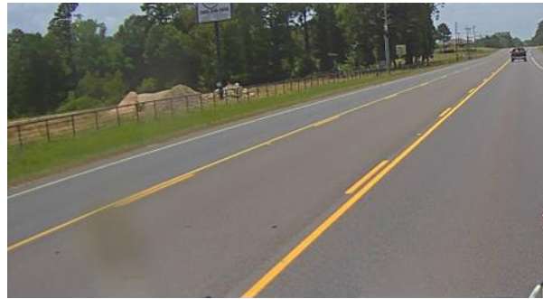
Example Current Condition Photo 2
