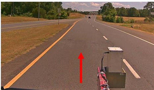
Example Current Condition Photo 1
