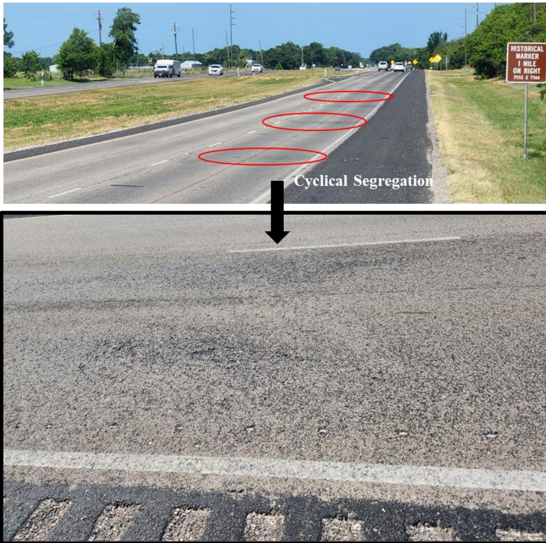
Figure 111. Cyclical Segregation on RMC Project.
