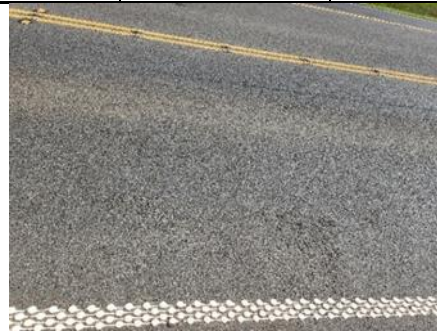
Example Current Condition Photo 2
