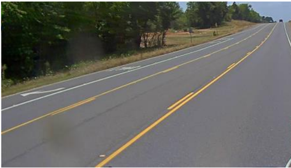
Example Current Condition Photo 1
