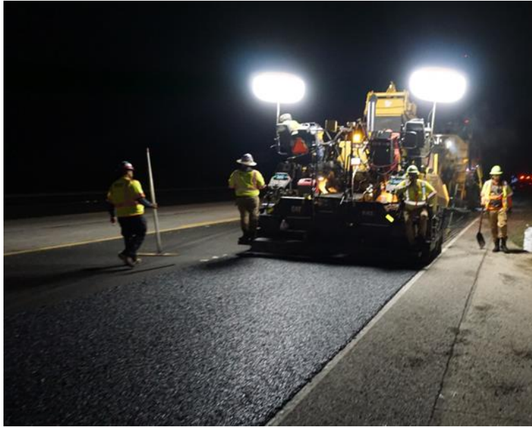
Figure 61. Paving Operation on SH 6.
