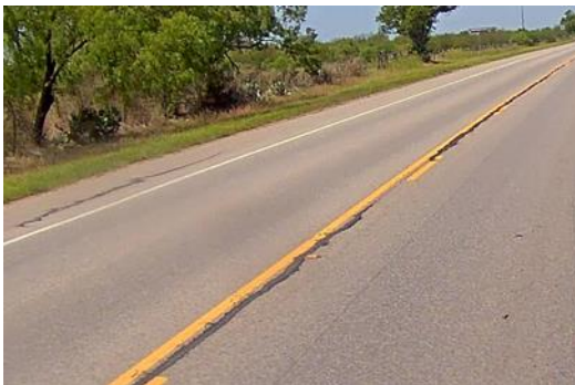
Example Current Condition Photo 1
