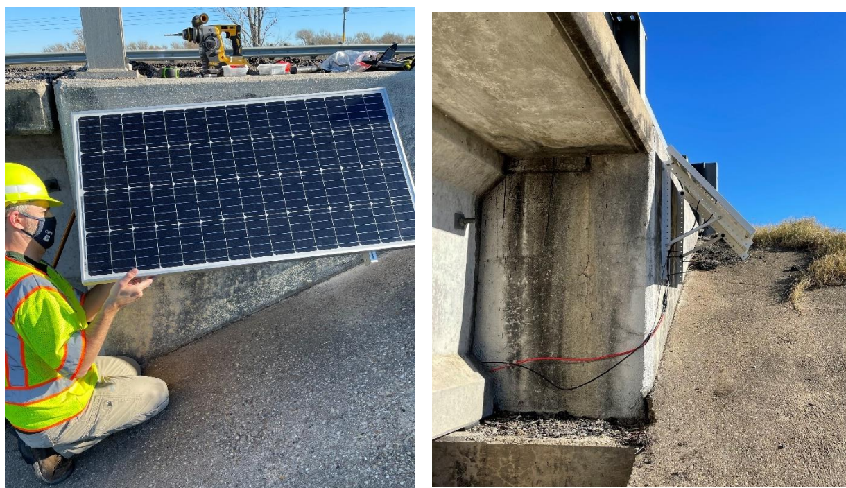
Figure 5.7. Installation of the Solar Panel.
