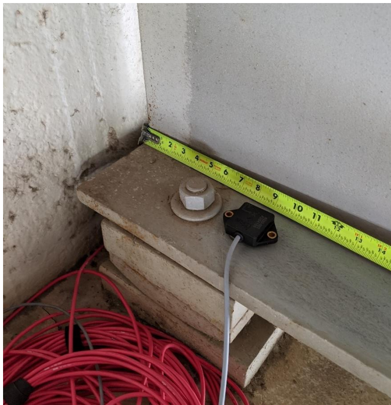
Figure 5.31. Accelerometer at North End (Bridge #3).
