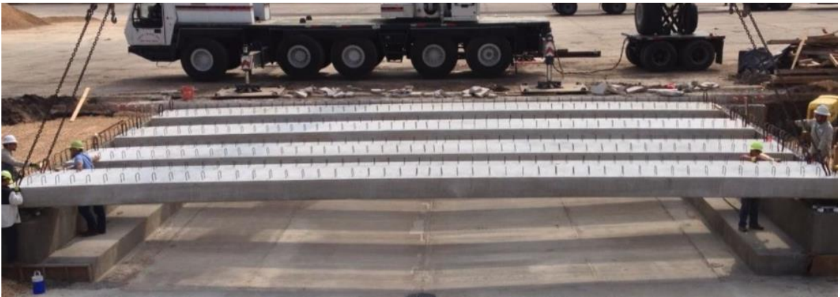
(b) Slab Beam Placement
