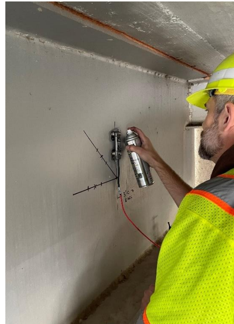
(b) Apply Paint to Protect the Steel
