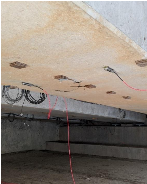
(c) Strain Gauges Installed at Midspan
