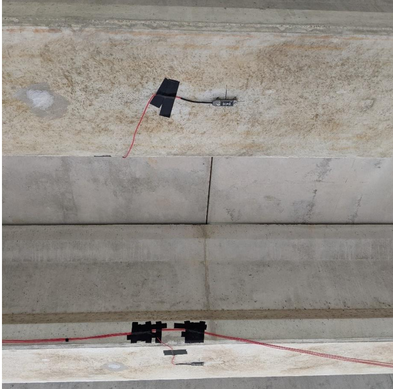
Figure 5.20. Midspan Strain Gauges (Bridge #2).
