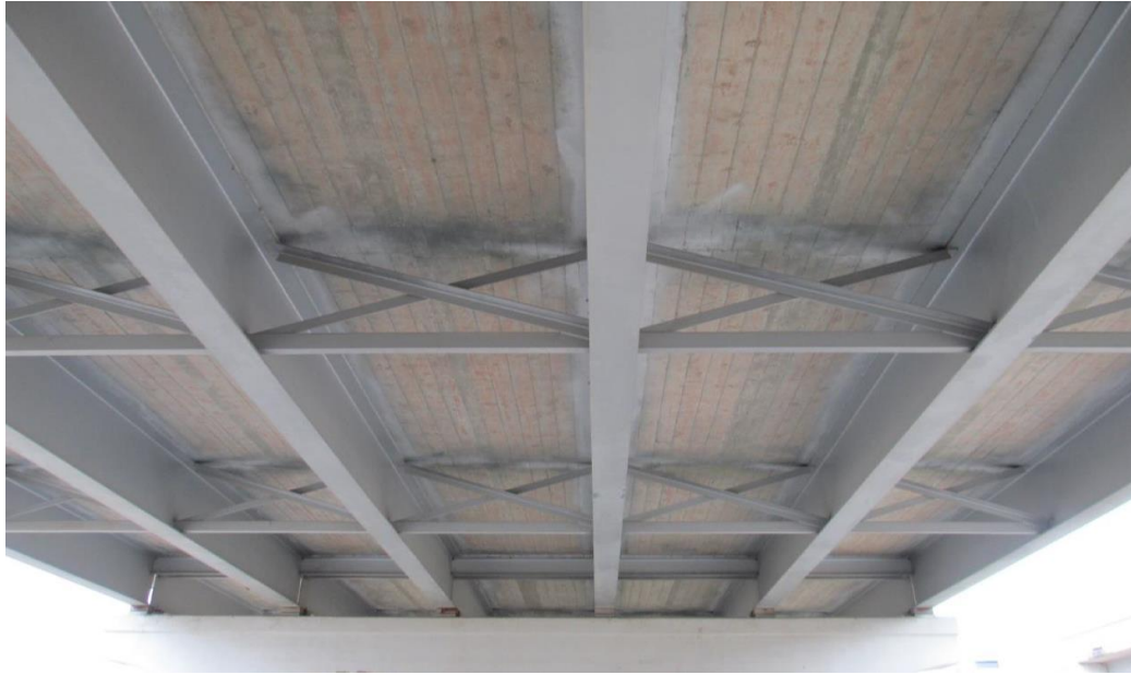
Figure 4.9: Bridge #3 Underside View.
