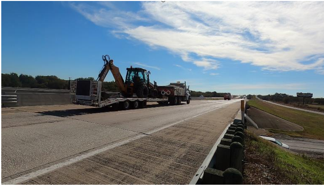
Figure 5.41. Truck B Passing the Inside Lane (Bridge #3).
