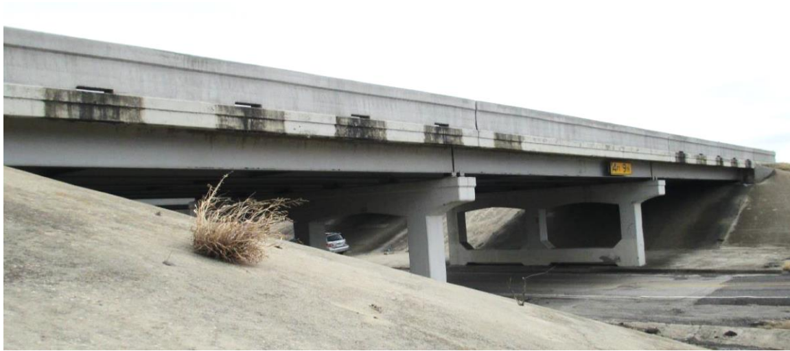
Figure 4.8: Bridge #3 Elevation View.
