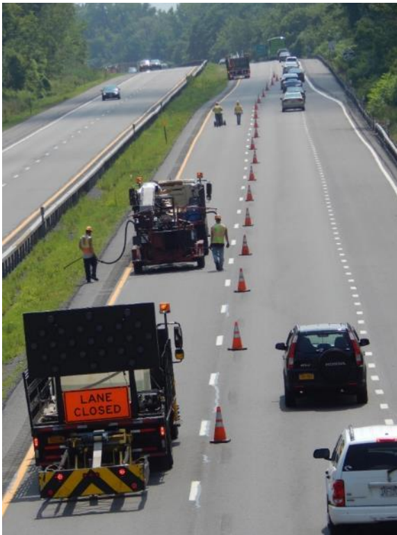
A.5 Traffic is kept off the crack sealant after installation
