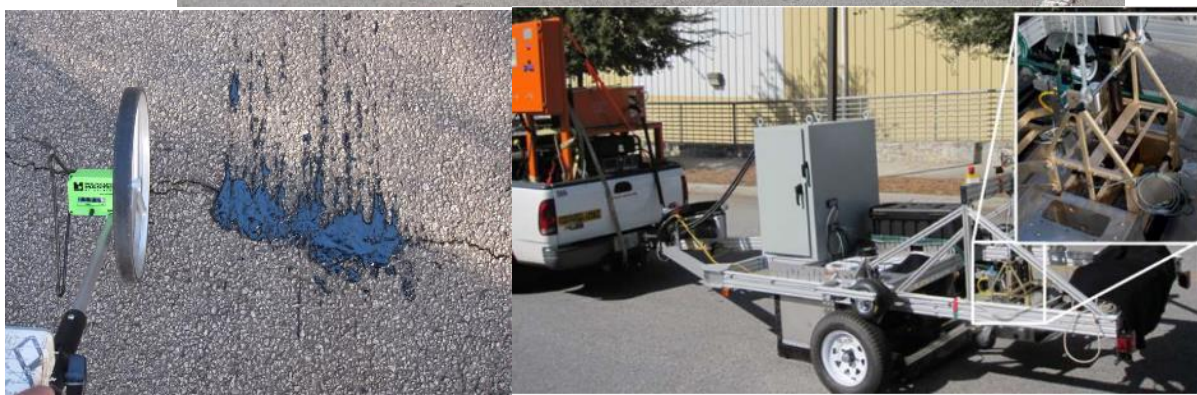
A.6 Simi-autonomous crack sealing technology (21).
