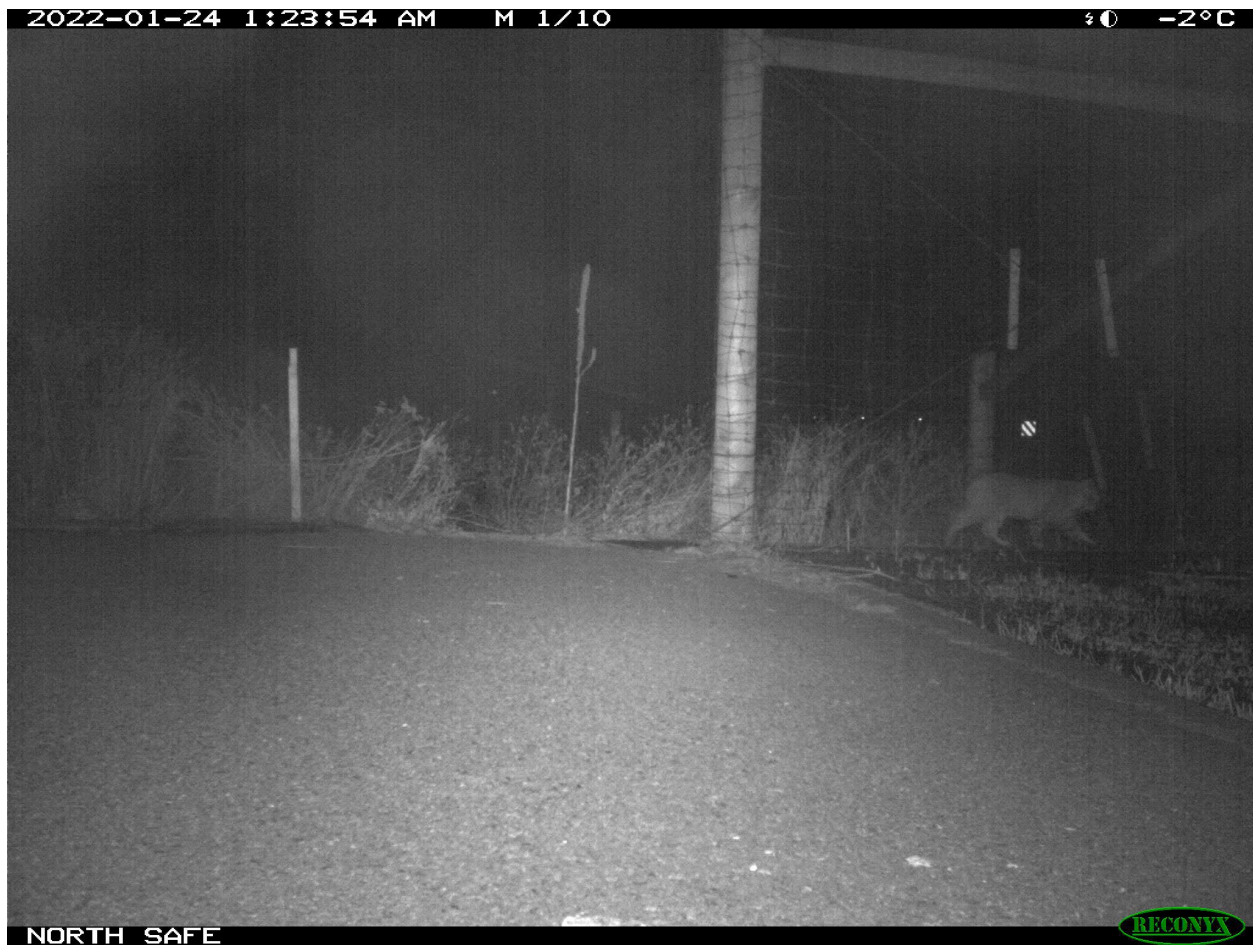
Figure 11: A bobcat enters the fenced road corridor by walking on the accessible concrete edge of the pit under the grate of the wildlife guard. There is no electrified barrier installed yet at the time of the event.
