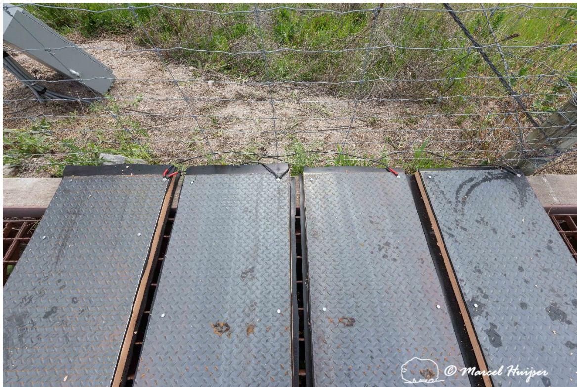
Figure 3: The electrified mat by Crosstek covers the concrete edge around the pit, at the north wildlife guard, US Hwy 93, south of Ravalli, Montana.
