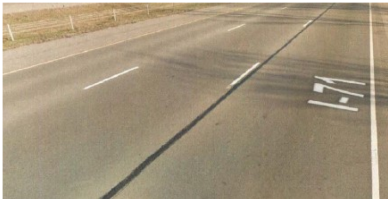
Figure 2.17 Crack sealing in Ohio (63)
