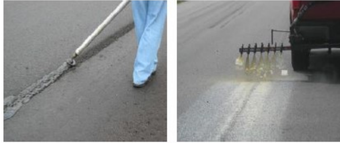
Figure 2.9 Application of joint adhesive and sealants (16)
