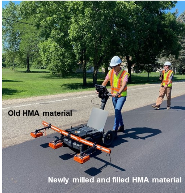
Figure 3.5 DPS data collection on confined butt joint - M-89 project, MI
