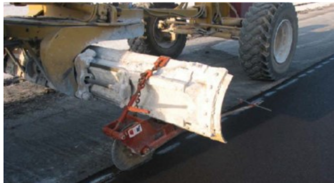
Figure 2.8 Cutting wheel attached to grader (2)
