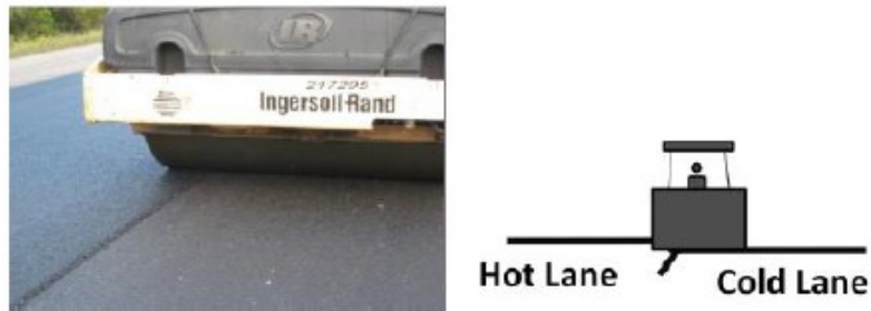
Figure 2.3 Cold roll method (16)
