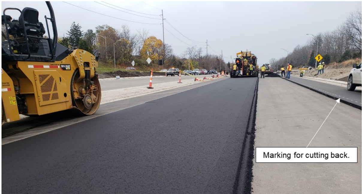
Figure 3.7 Paving operation on I-496, East Lansing, MI
