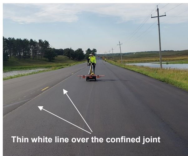
Figure 5.5 Appearance of a thin white line over the confined joint using the Maryland method at the Manning Trail project, MN
