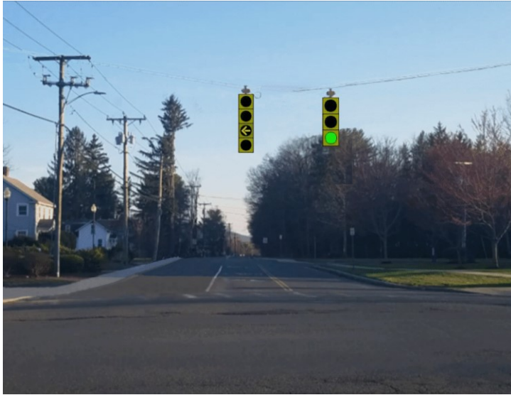
Figure 2.17 Question 12 - Four-Head Flashing Yellow Arrow without Sign. The image was animated to show flashing.
