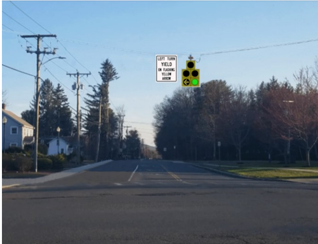
Figure 2.18 Doghouse signal head used in Questions 48 and 50. The yellow arrow was flashing, and the sign was not present for Question 48.
