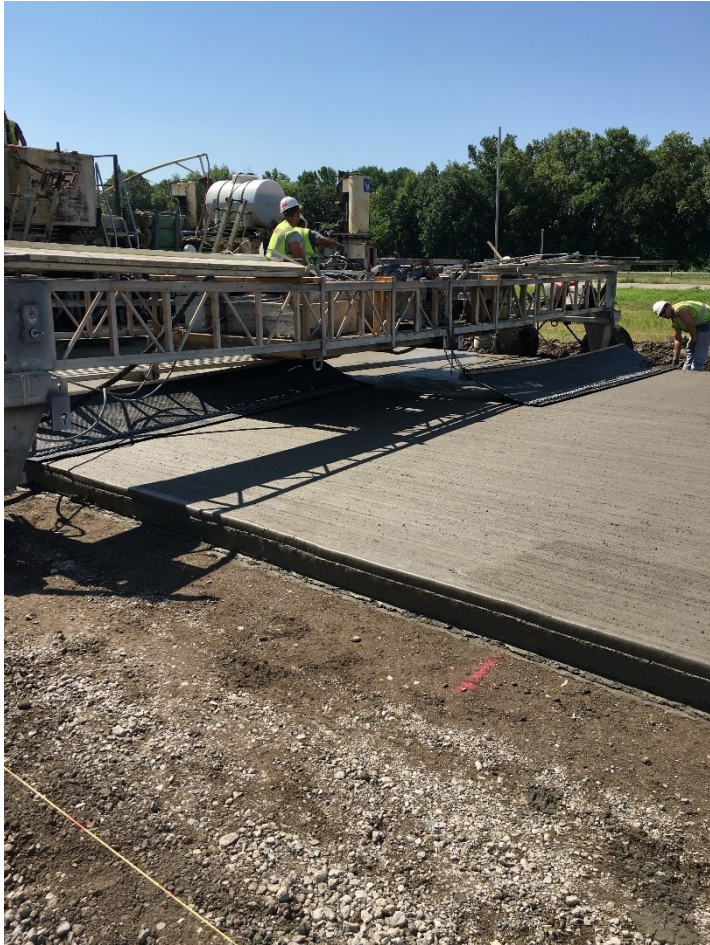
Figure 7-2 Concrete Finishing for CarbonCure RGC1 Test Section 2210
