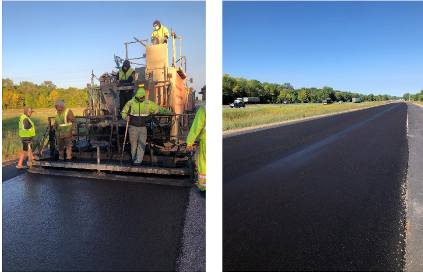
Figure 4-5 Application of Microsurfacing on Test Sections 2204 and 2205
