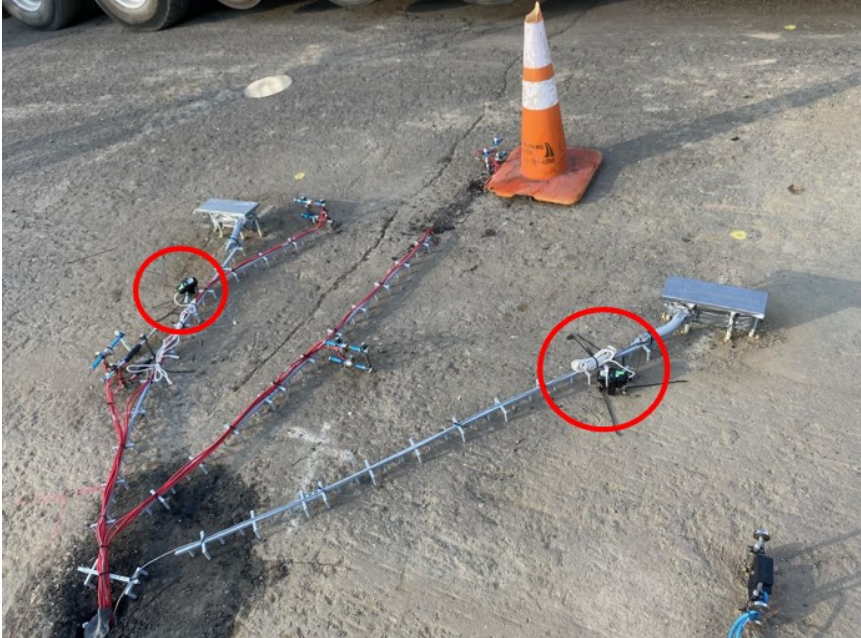
Figure 10-9 Maturity Sensors Installation Alternative Cementitious Materials Test Sections
