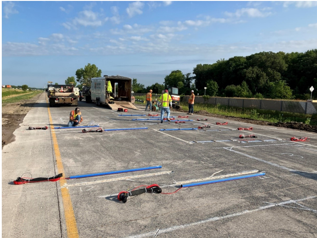
Figure 9-7 Installation of WIM System Sensors in Test Section 2225 during July 2023
