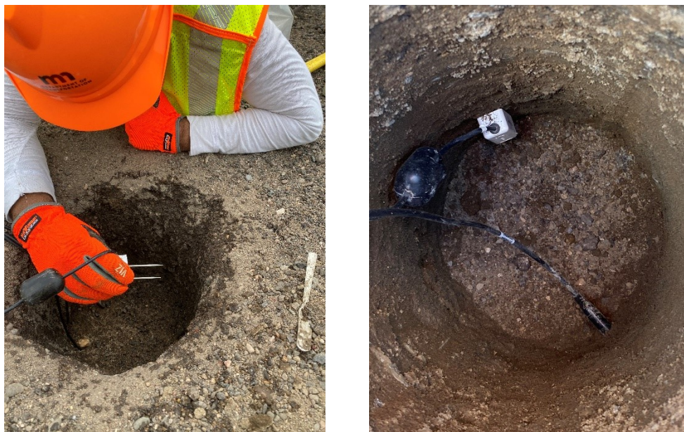
Figure 3-3 TEROS 10 and TEROS 21 Moisture Sensors Installation
