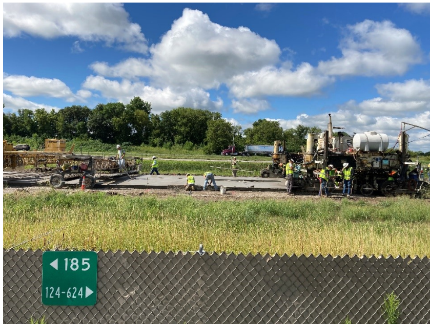
Figure 7-6 Concrete Finishing for CarbonCure Control Test Section 2217
