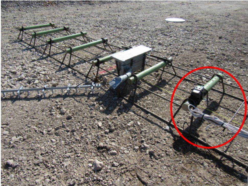
Figure 7-10 Maturity Sensors Installation for Carbon Dioxide Test Sections
