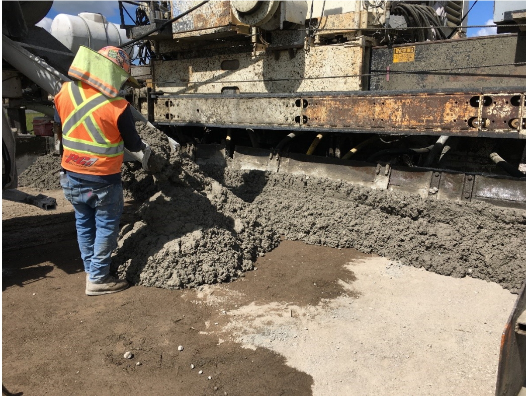
Figure 8-3 Concrete Placement for Ash Grove ACM Test Section 2214
