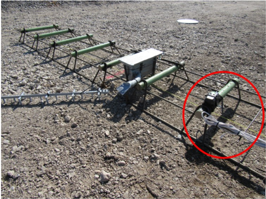
Figure 8-10 Maturity Sensors Installation Alternative Cementitious Materials Test Sections
