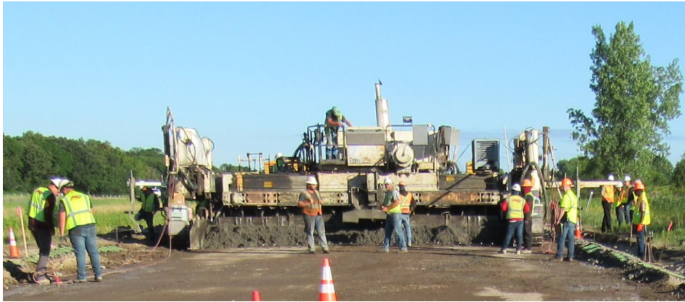
Figure 7-5 Concrete Placement for Carbon Upcycling Processed Fly Ash Test Section 2213
