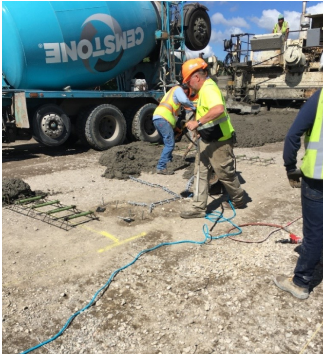
Figure 7-4 Concrete Placement for CarbonCure RGC3 Test Section 2212
