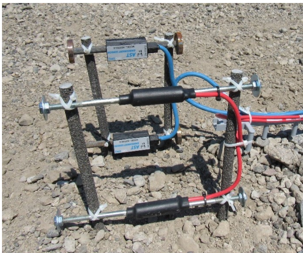
Figure 14-13 Concrete Embedded Strain Gauges used in MnROAD 2022 Construction
