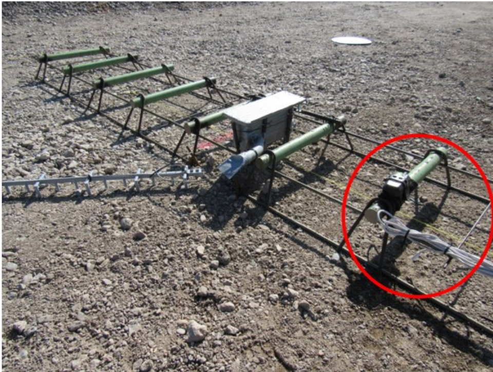
Figure 6-11 Maturity Sensors Installation for Alternative Pozzolanic Materials Test Sections
