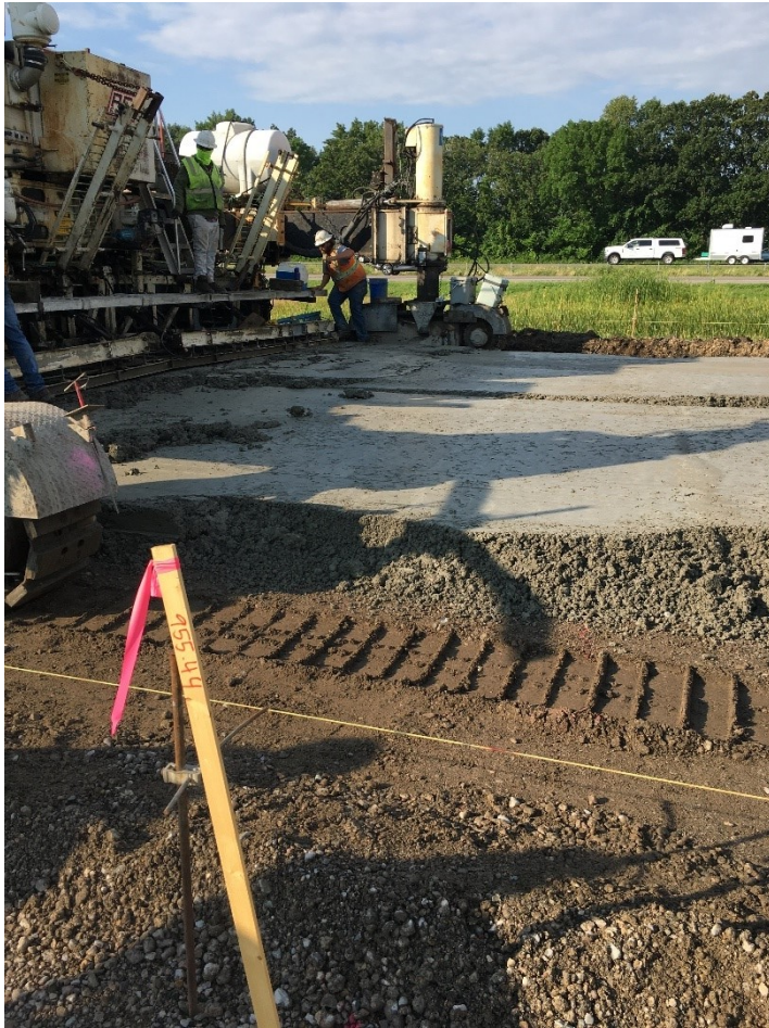
Figure 8-2 Concrete Placement for Ultra High Material ACM Test Section 2209
