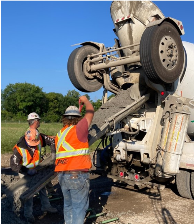
Figure 6-6 Concrete Placement for Burgess Pigments Natural Pozzolan Test Section 2220
