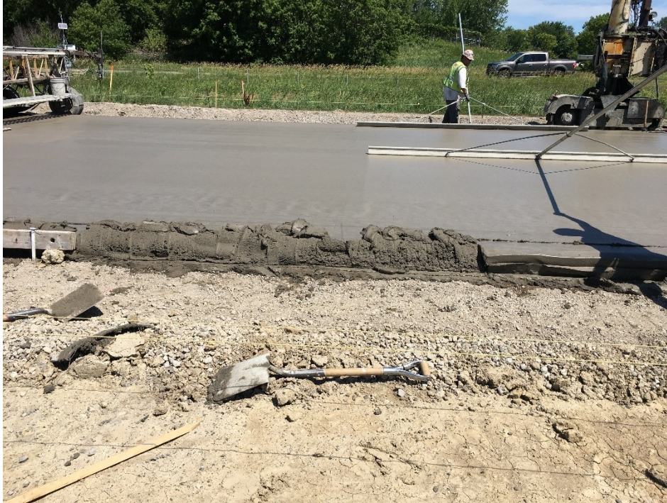
Figure 8-4 Concrete Finishing for Terra CO2 Manufactured Fly Ash Test Section 2216
