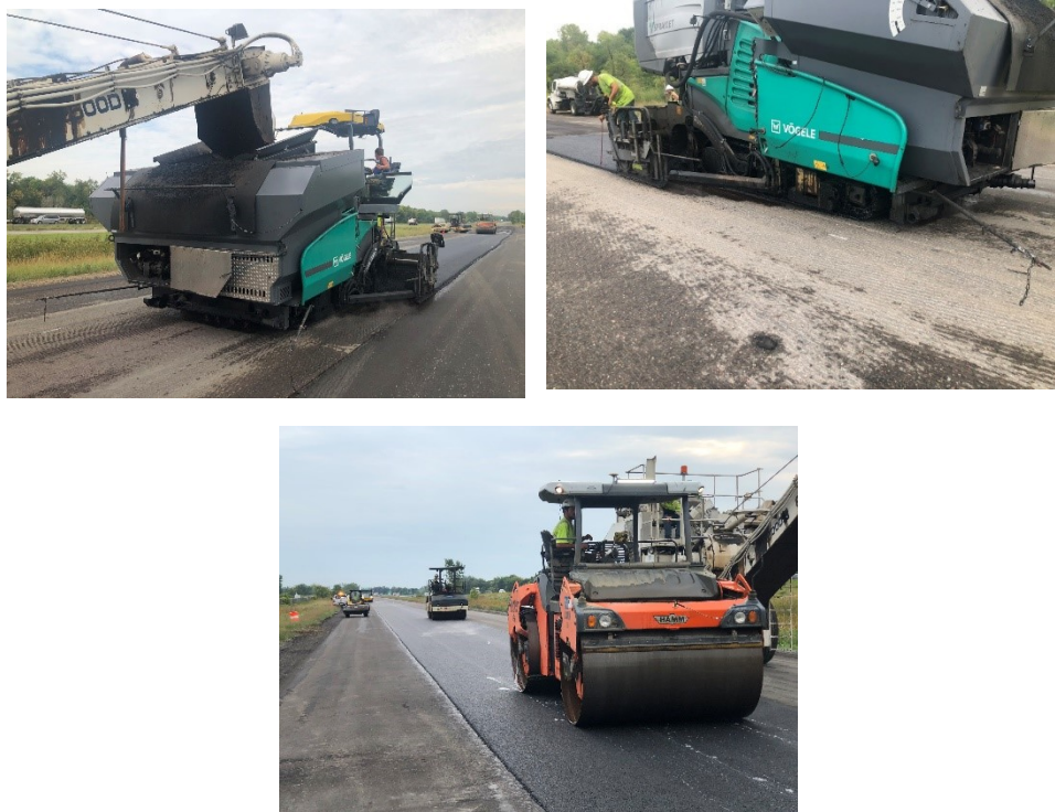
Figure 4-4 UTBWC Placement on Test Sections 2201, 2202, 2203, 2206, 2207 and 2208
