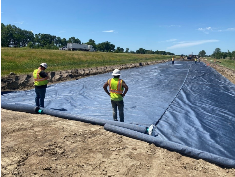
Figure 3-7 Wicking Geotextile Installation
