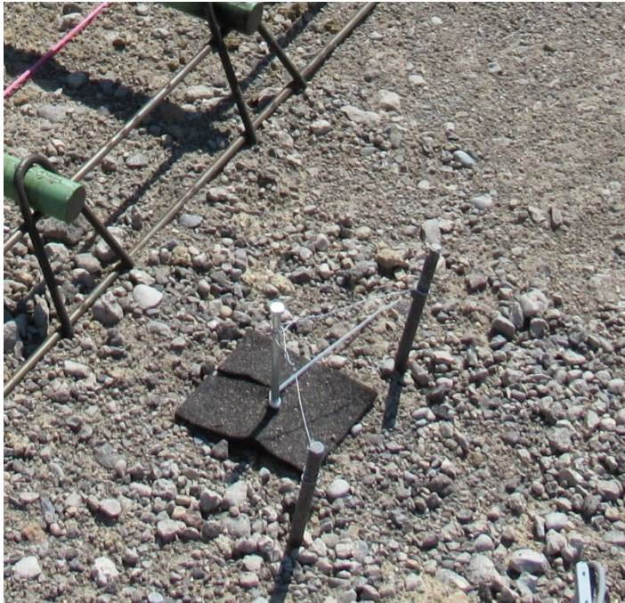
Figure 14-9 Magnetic Induction Sensor Installed in Base Material
