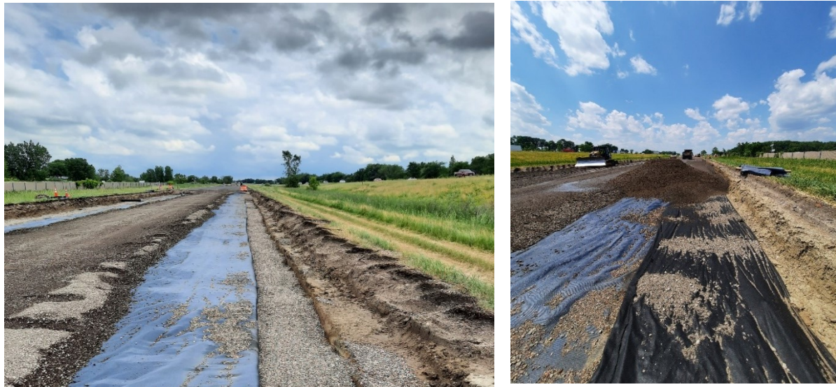
Figure 12-9 Trench with Gap Graded Aggregate and Non-woven Geotextile.
