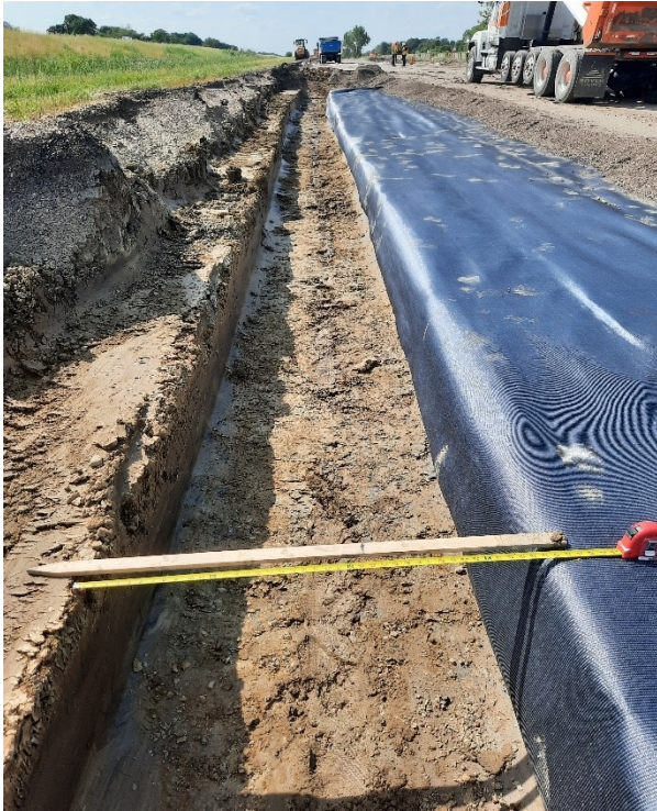
Figure 12-8 Figure 12.8 Width and Depth of the Trench
