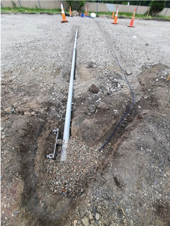
Figure 12-12 Installation of Shape Array Sensors
