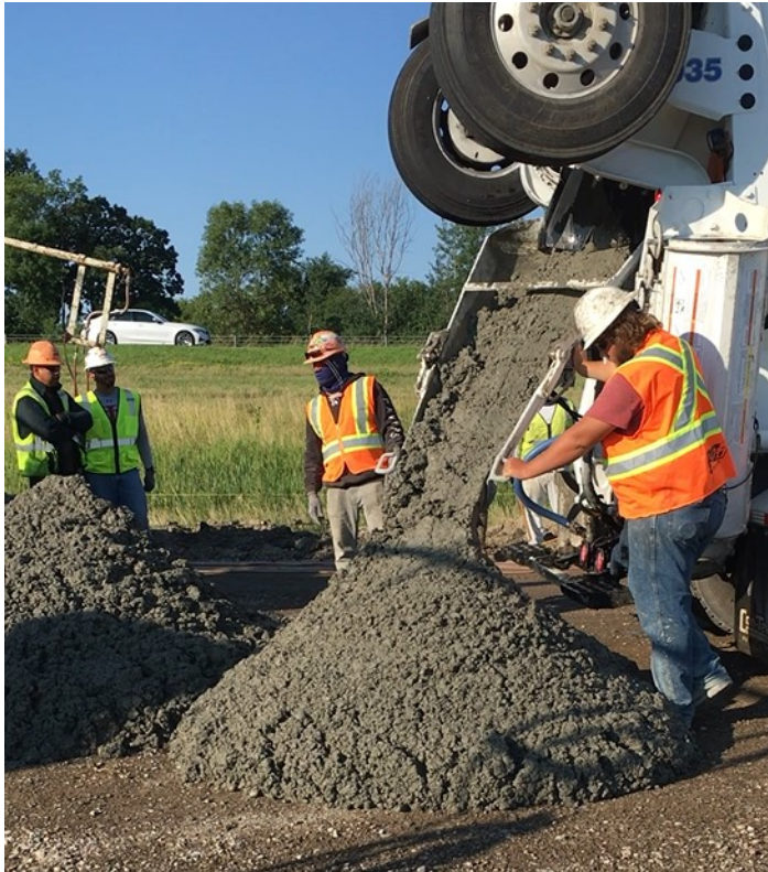
Figure 6-4 Concrete Placement for Hess Pumice Natural Pozzolan Test Section 2222
