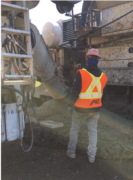
Figure 6-5 Concrete Placement for 3M Natural Pozzolan Test Section 2221
