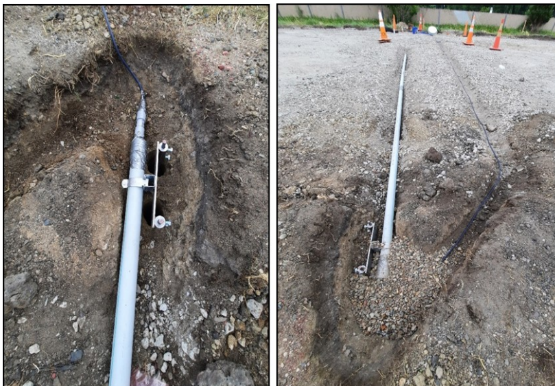
Figure 3-9 Fixing the Reference Point of SAA
