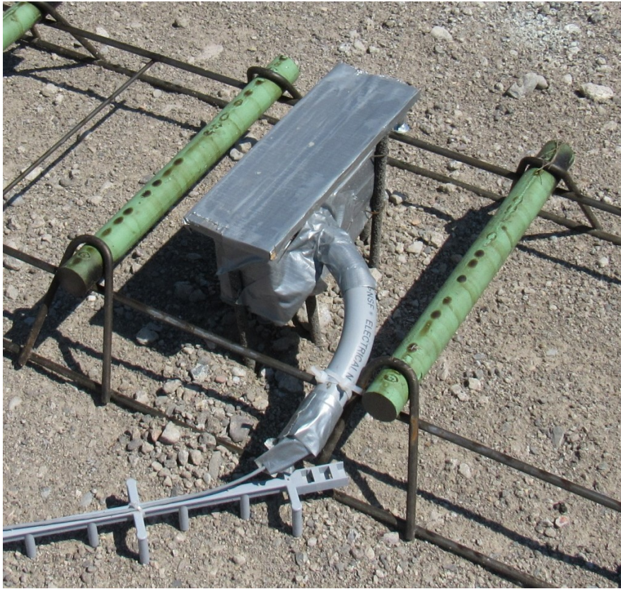
Figure 14-7 Joint Gauge (JG) Block Out
