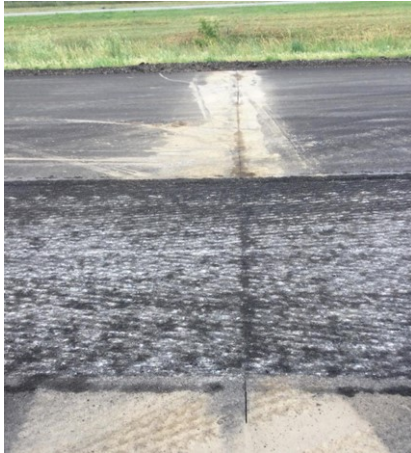
Figure 13-5 Pavement Surface Appearance after Saw-cut and Partial mill
