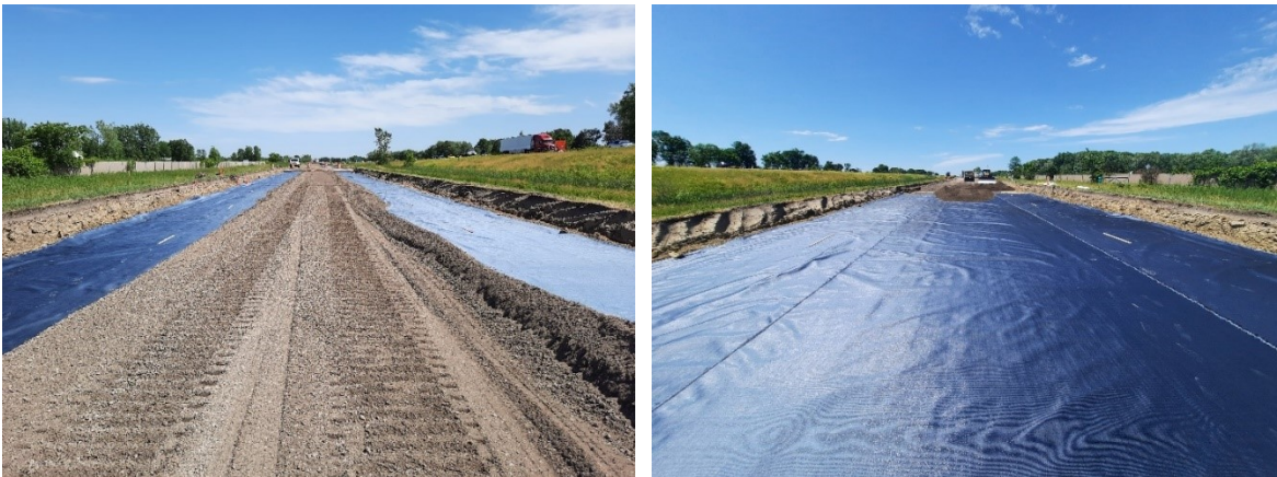
Figure 12-6 Installation of Wicking Geotextile at the Interface of Subgrade and Subbase
