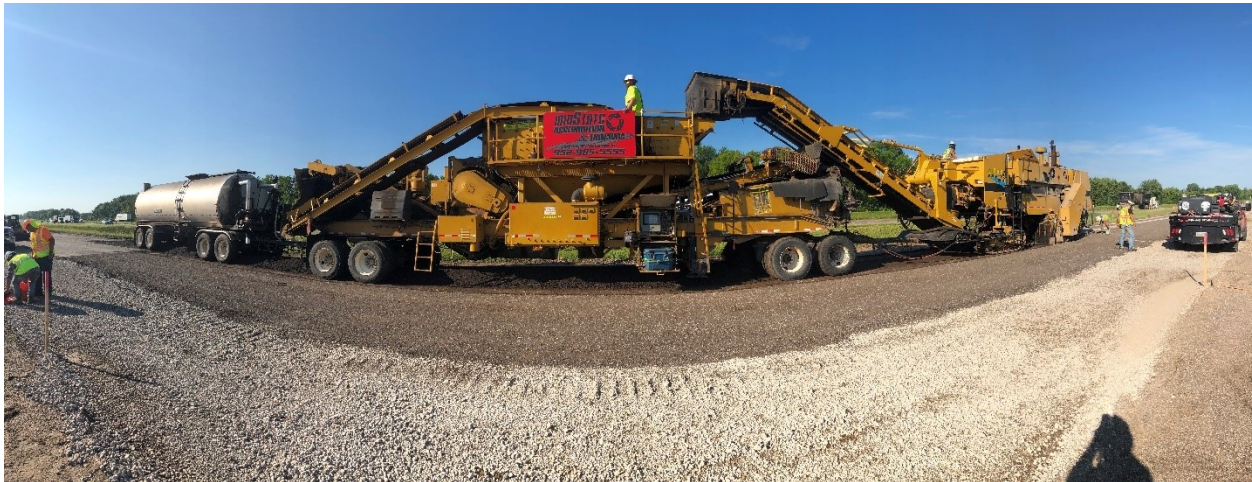
Figure 4-3 Cold in Place Recycling Train
