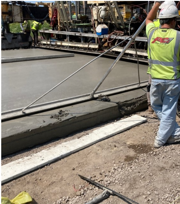
Figure 9-3 Concrete Finishing for WIM Test Section 2225
