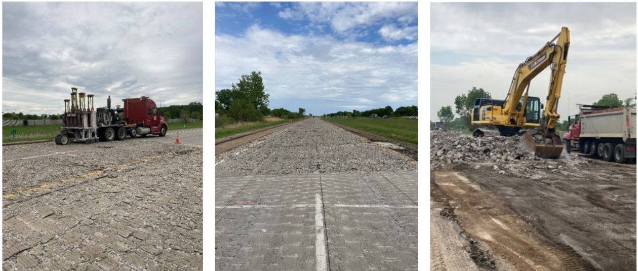
Figure 2-3 Existing Test Sections Concrete Removal
