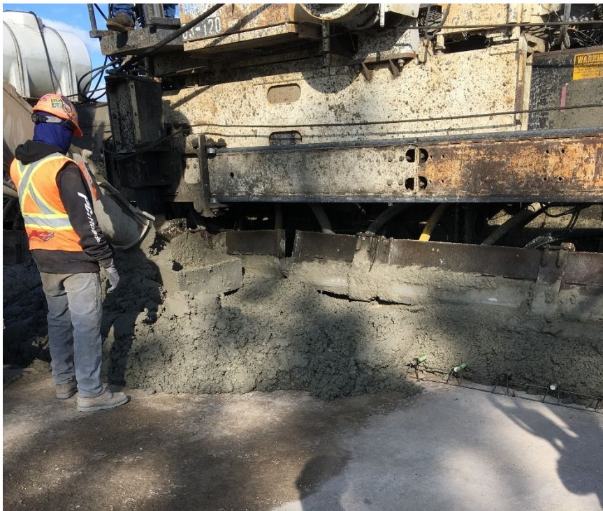
Figure 6-2 Concrete Placement for Urban Mining Ground Glass Test Section 2215
