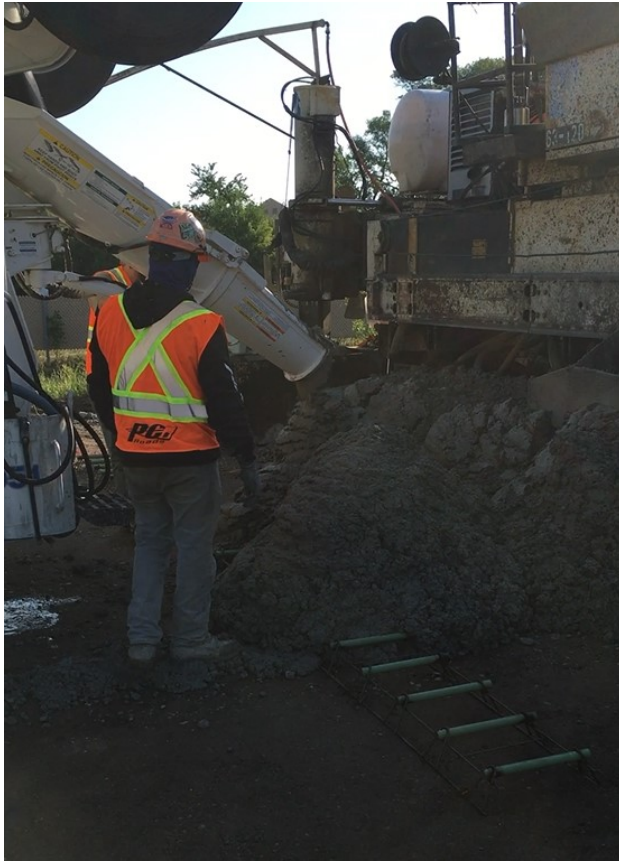
Figure 6-3 Concrete Placement for Carbon Limit Blended ASCM Test Section 2224
