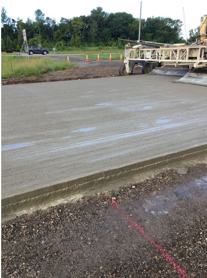
Figure 8-6 Concrete Finishing for Control Test Section 2218
