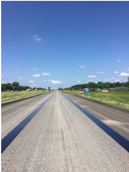
Figure 13-6 VRAM Application on the Centerline of Test Sections 2230 to 2239
