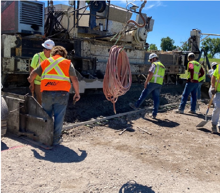
Figure 8-5 Concrete Placement for Continental Cement High Limestone Test Section 2223
