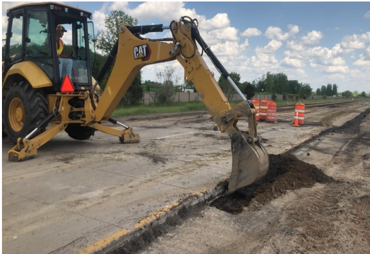
Figure 2-4 Concrete Removals Over HMA Layer in Former Test Sections 614 to 914
