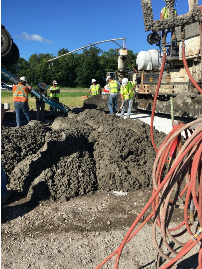
Figure 7-3 Concrete Placement for CarbonCure RGC2 Test Section 2211
