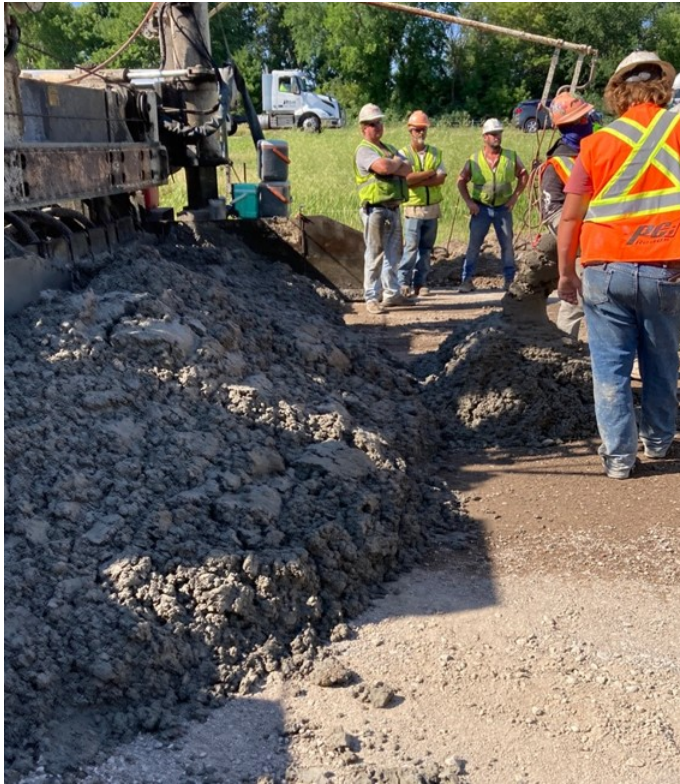
Figure 6-7 Concrete Placement for CPTECH Center Optimized Mix Test Section 2219
