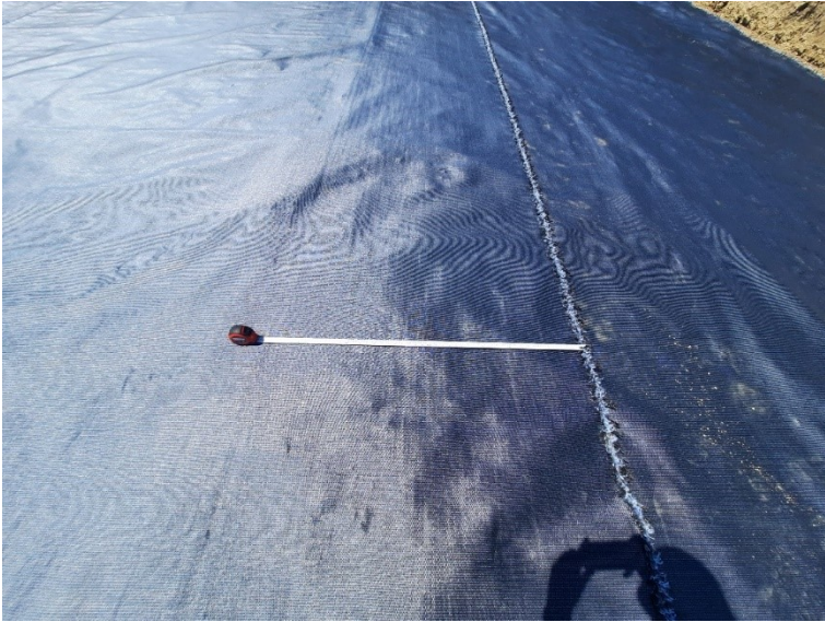
Figure 12-7 Overlapping of Geotextile
