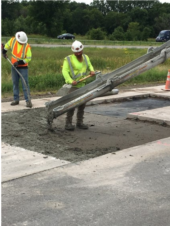
Figure 5-4 Placement of Concrete in Repair Panels in Test Section 160
