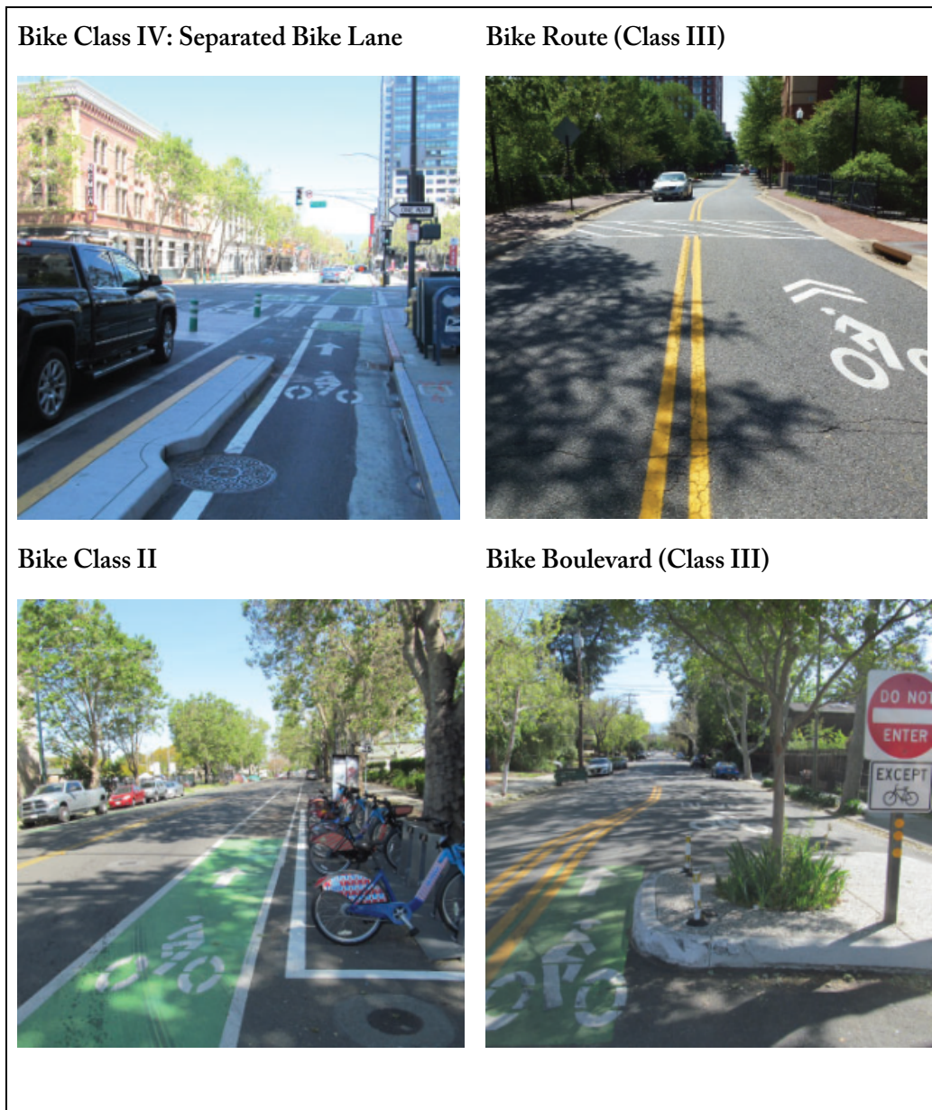
Figure 4. Examples of Different Bike Lane Classes from San José, CA (City of San José Department of Transportation, 2020)
