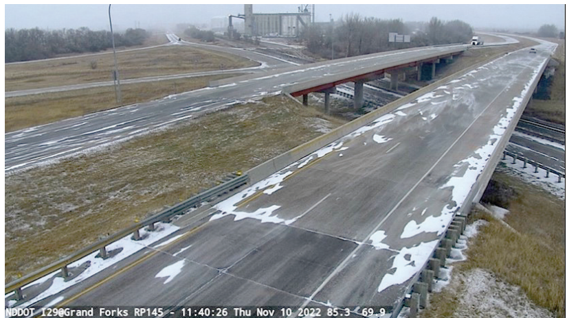
RWIS camera image showing snow on the shoulders and traces of snow in the lanes
