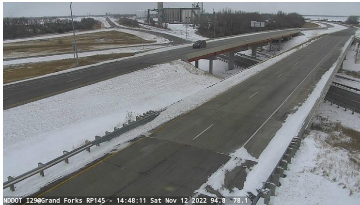
Figure 7. I-29 at Grand Forks Exhibiting Some Snow on the Shoulders but No Snow in the Traffic Lanes
