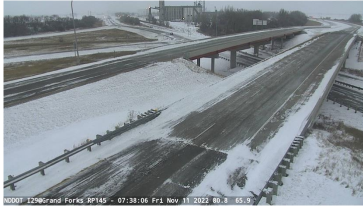
Figure 6. I-29 at Grand Forks exhibiting snow primarily on the shoulders but traces on the traffic lanes
