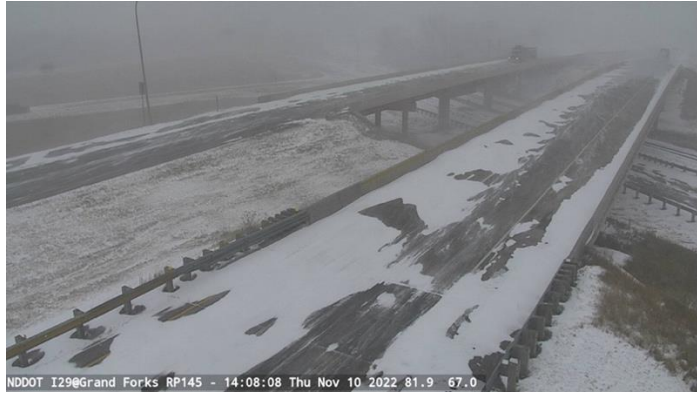
Figure 4. I-29 at Grand Forks exhibiting low visibility and problematic snow on both the shoulders and traffic lanes
