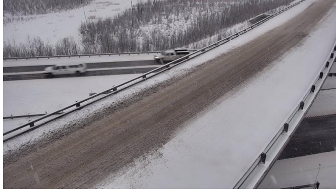
Figure 13. Camera image of bridge in Alaska belonging to “slush” and “snow covered” categories simultaneously
