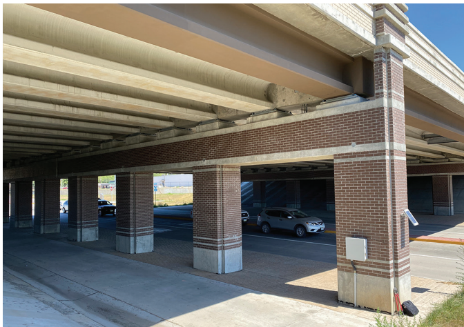
Instrumented frame pier of the 418 Woodbury bridge
