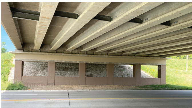
Instrumented frame pier of the 318 Scott bridge
