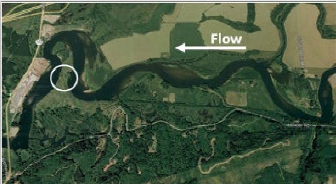
B. 2006 photo of SR 107 crossing of Chehalis River.
