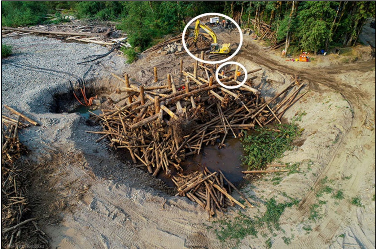
Figure 8.8. Engineered logjam (ELJ) built in 2018 to deflect flow into a side channel of the Sandy River, Oregon. Note excavator and people circled for scale. Image used by permission of Wolf Water Resources Inc.
