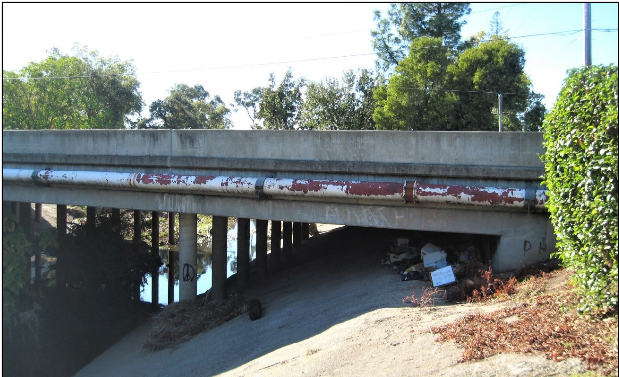
Figure 8.11. Debris (under the bridge) that may soon be in the waterway.
