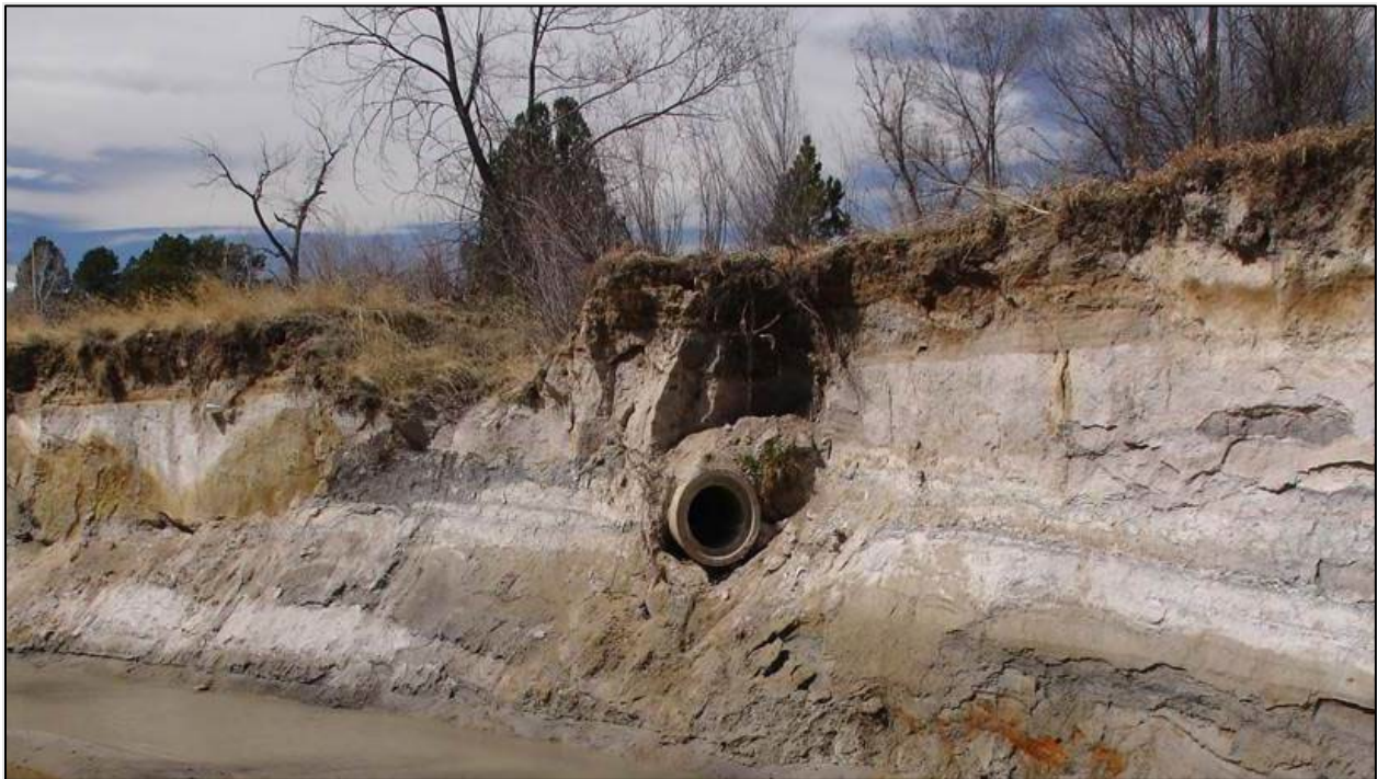
Figure 6.12. Channel bank with multiple sediment layers. Image used by permission of Tetra Tech, Inc.
