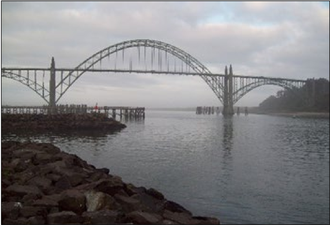
Figure 8.21. Tidally influenced Yaquina River at the Highway 101 bridge crossing near Newport, Oregon. Image used by permission of WEST Consultants, Inc.
