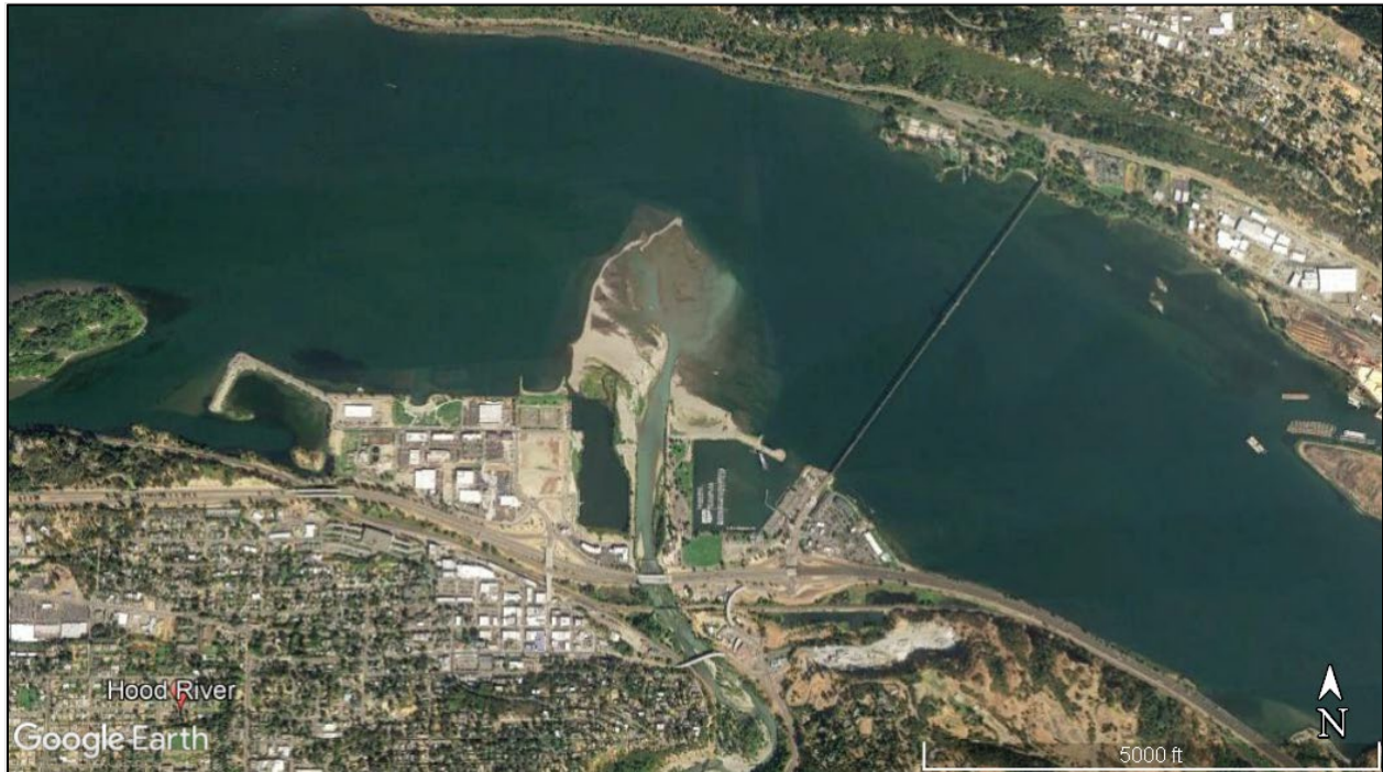
Figure 8.2. Delta formed in 2018 by flooding at the Columbia River/Hood River confluence in Oregon.
