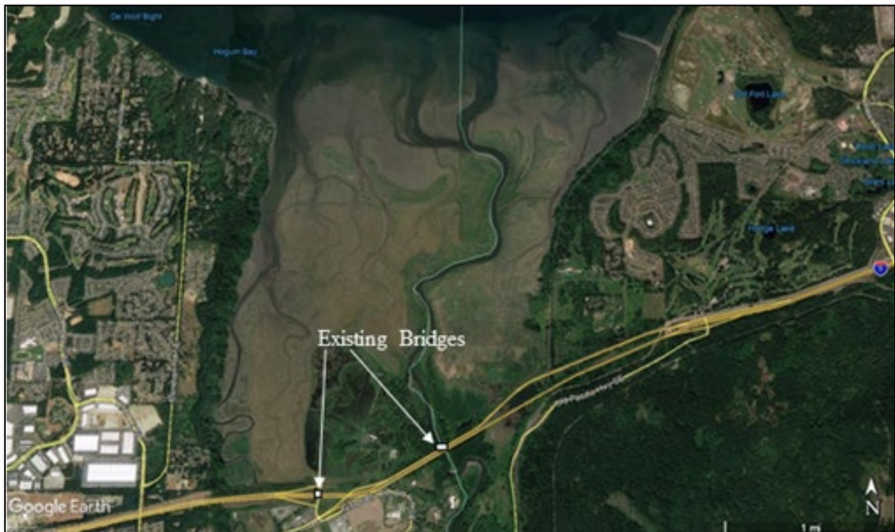
Figure 8.26. Interstate 5 crossing of the Nisqually River delta, Washington State.
