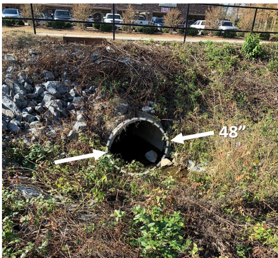
Figure 3: The outlet at monitoring Site 591 Site 573
