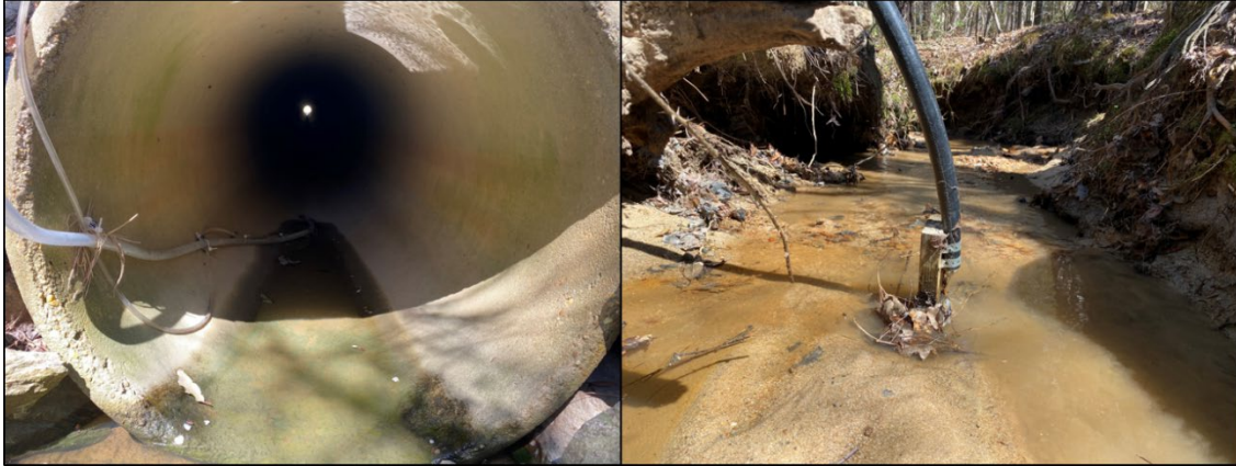
Figure 4. Monitoring setup of bubbler and sampler tubing in pipe (left) and channel (right)
