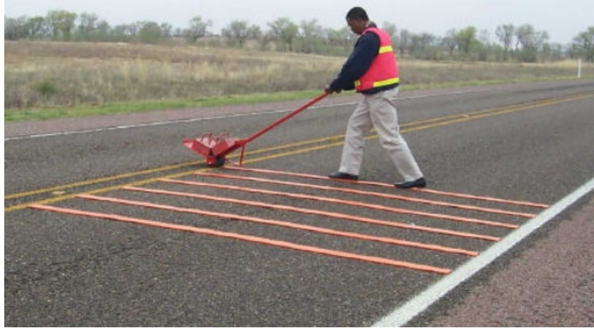
Figure 5. Photo. Rumble strips in work zone.
