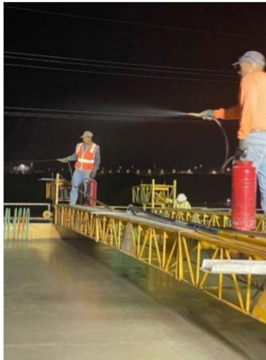
Figure 2.66: Applying Finishing Aid to the Concrete Surface
