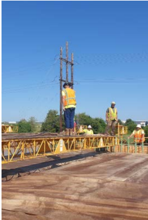
Figure 2.68: Rewetting the Burlap on the Deck
