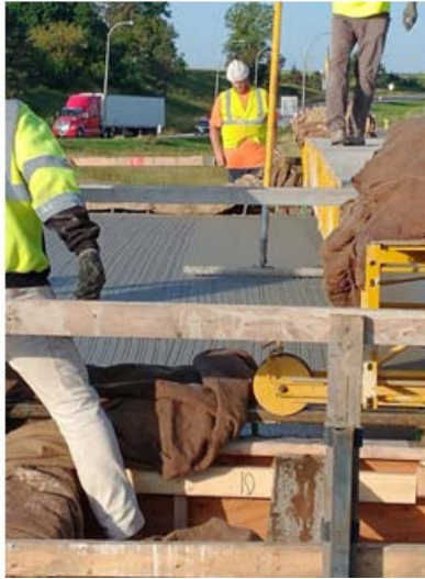
Figure 2.31: Tining the Deck Before Application of Curing Compound
