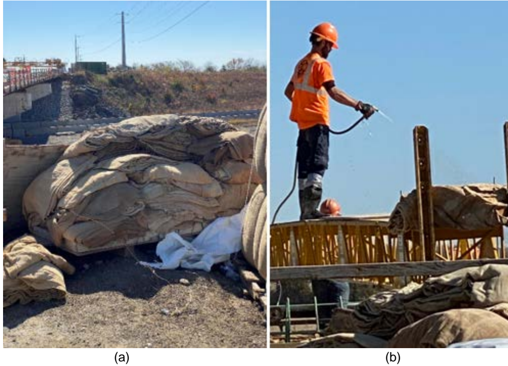
Figure 2.54: Burlap Placement of KS-IC-LC-HPC-2 (a) Dry Burlap; (b) Wetting the Burlap on the Deck
