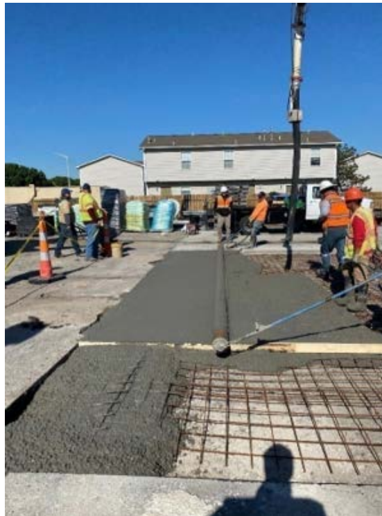
Figure 2.63: The Qualification Slab Placement Equipment
