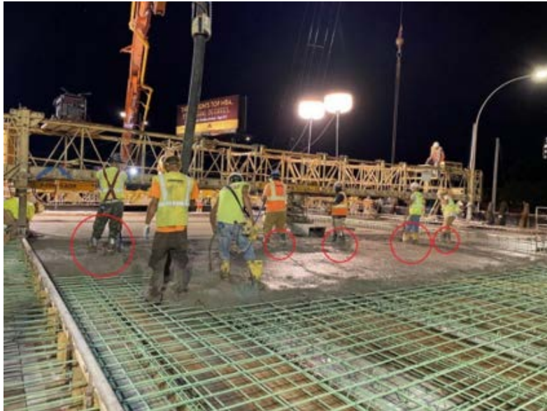
Figure 2.23: Walking Observed on Freshly Consolidated Concrete
