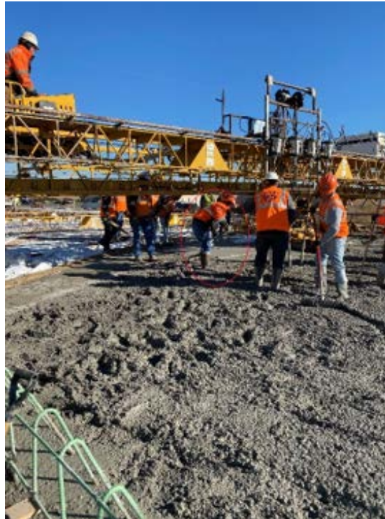
Figure 2.56: Walking Observed on Freshly Consolidated Concrete
