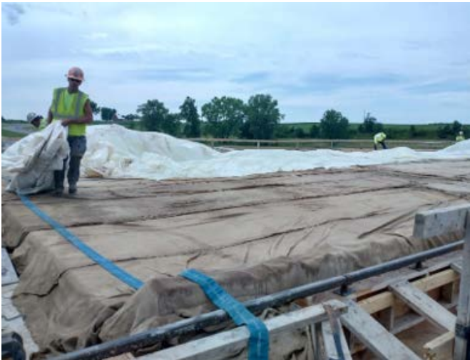
Figure 2.34: Covering the Deck with Wet Burlap and Plastic Sheeting
