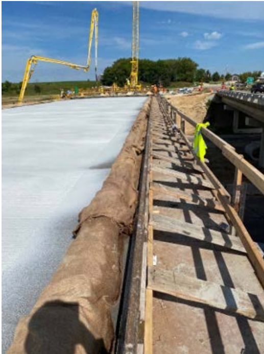
Figure 2.33: Burlap Placement on the Barrier Reinforcement
