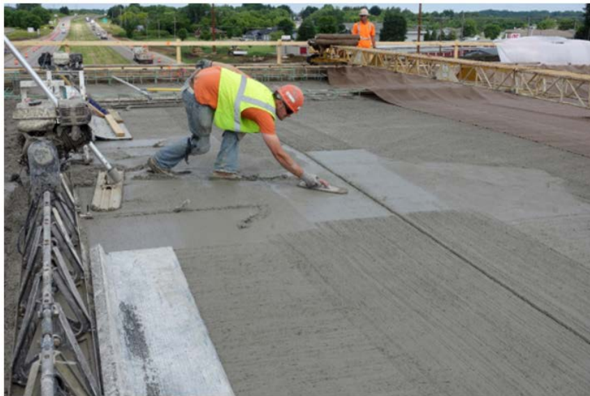
Figure 2.5: Walking through Freshly Consolidated Concrete
