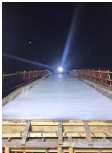
Figure 2.14: The Application of the Curing Compound on the Bridge Deck
