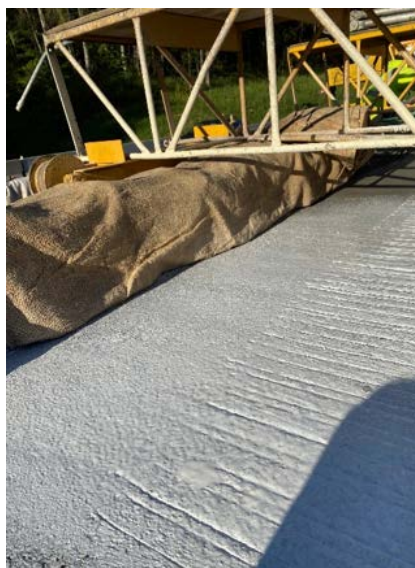
Figure 2.38: Burlap Placement on the Barrier Reinforcement
