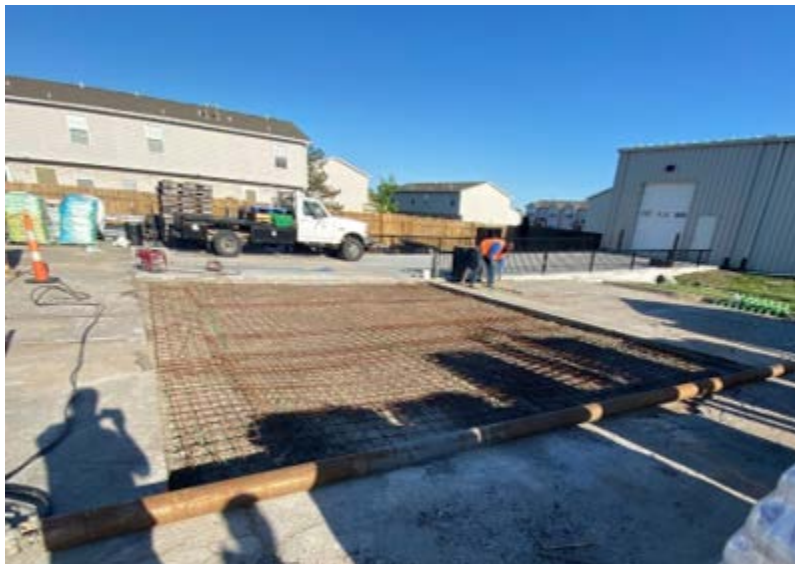
Figure 2.62: The Qualification Slab for KS-IC-LC-HPC-3
