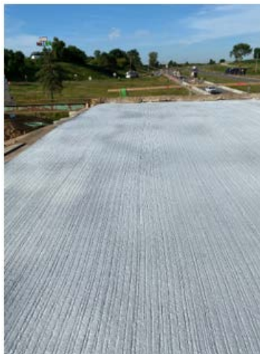
Figure 2.32: Non-Uniform Distribution of Curing Compound on the Deck
