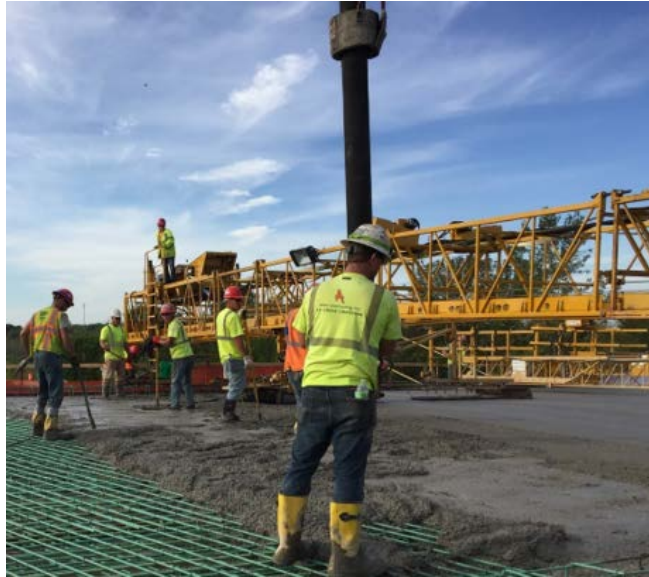
Figure 2.17: Placing, Consolidation, and Finishing Equipment
