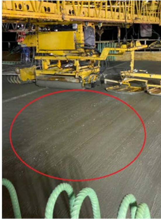
Figure 2.65: A Leaking Pipe Leaving Water Droplets on the Deck Surface
