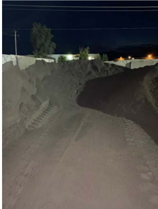
Figure 2.35: Disturbance of the Bottom of the Stockpile
