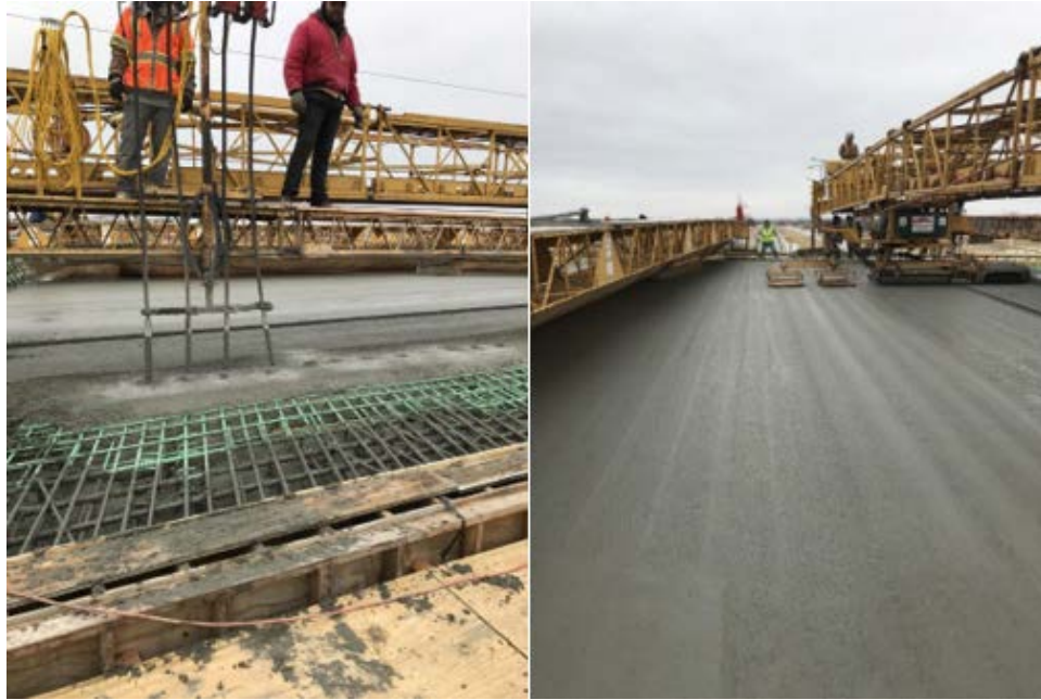
(a) (b) Figure 2.42: Placement Equipment (a) Manually Operated Gang Vibration System; (b) Double-Drum Roller Screed Followed by Two Metal Pans
