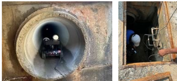
Figure 41 Husarion ROSbot positioned at pipe entrance with tether being connected
