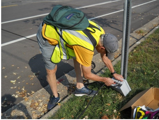
Figure 3.2: Setting up a traffic recorder
