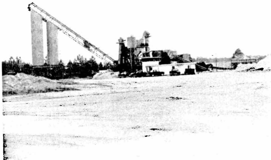
FIGURE 4 Batch Plant Used to Process Recycled Mixture
