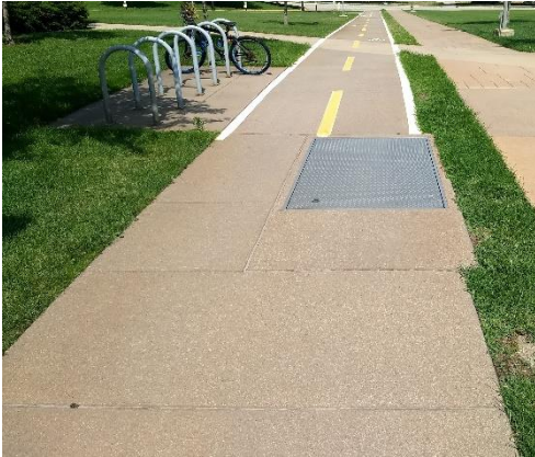
a) Tunnel Access on Purdue University Campus
