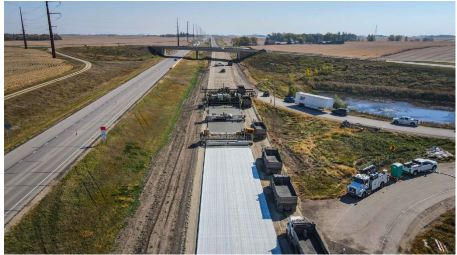
Concrete paving on TH 52 Cannon Falls to Zumbrota design-build
