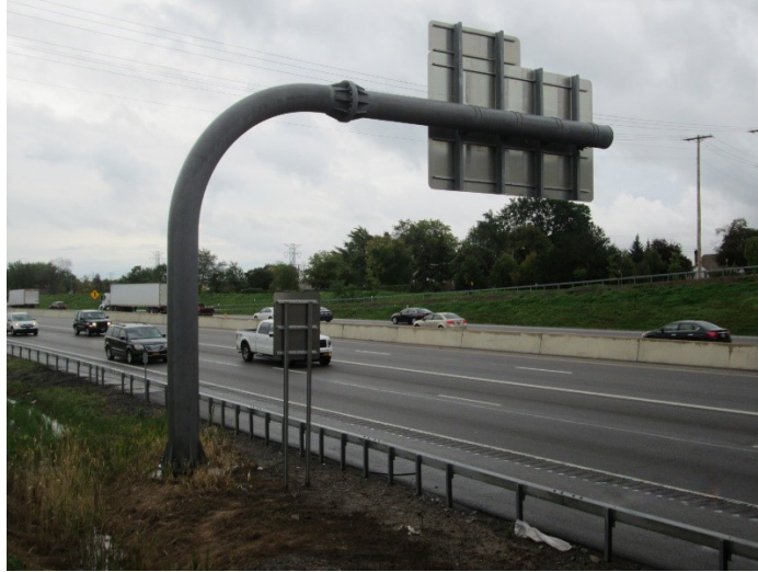
Figure 14. Photo. Monotube cantilever.
