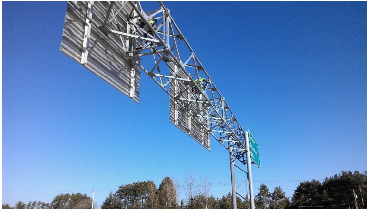
Figure 82. Photo. Inspectors climbing a four-chord full span structure.
