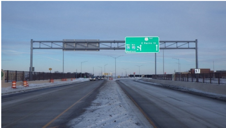
Figure 26. Photo. Bridge-mounted full span structure.
