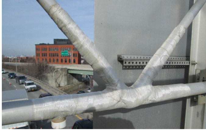
Figure 114. Photo. FRP wrap repair on an aluminum span.
