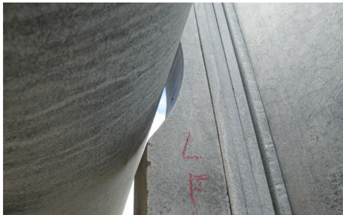
Figure 102. Photo. Gap between vertical saddle and chord.
