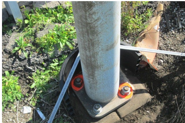
Figure 90. Photo. Pipe half section retaining structure repair.
