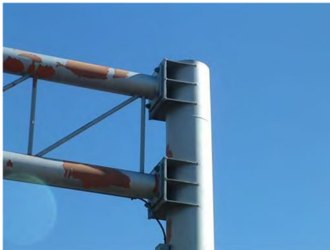
Figure 43. Photo. Bolted span-to-post connection.
