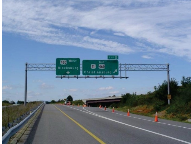
Figure 3. Photo. Three-chord full span.
