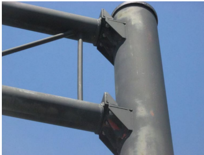
Figure 39. Photo. Bolted corbel span-to-post connection.
