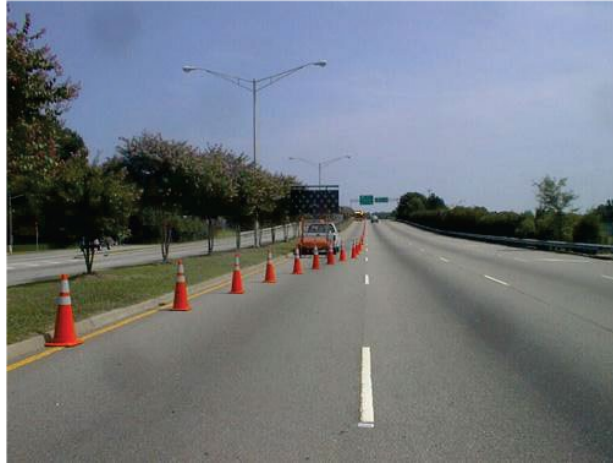
Figure 52. Photo. Stationary left lane closure.
