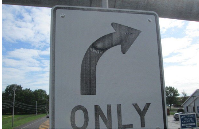
Figure 113. Photo. Faded sign panel.
