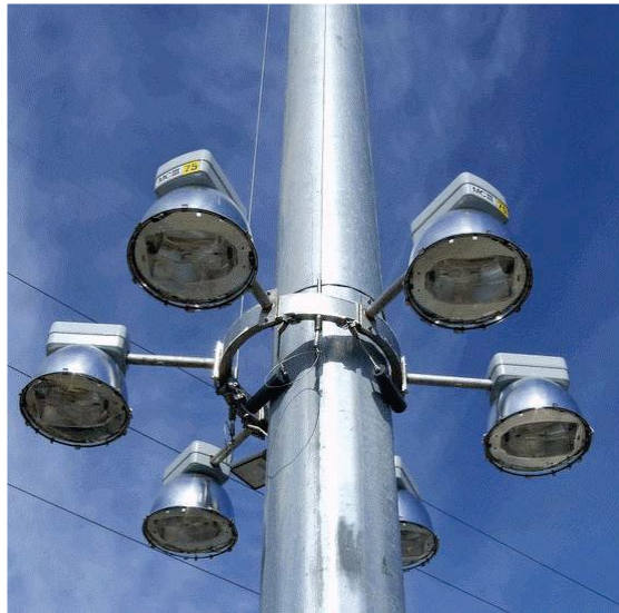
Figure 21. Photo. High mast light ring.
