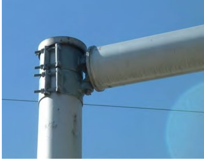
Figure 38. Photo. Pinned span-to-post clamp connection.
