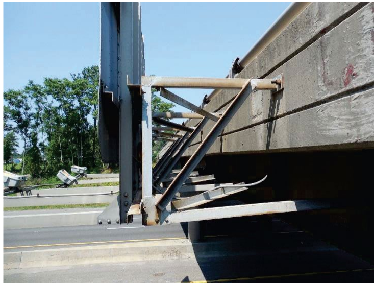
Figure 22. Photo. Bridge-mounted structure.
