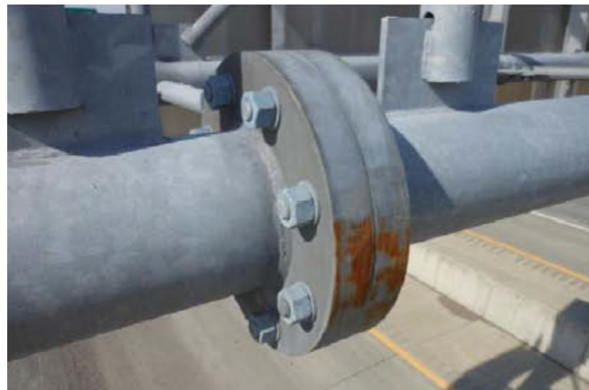
Figure 46. Photo. Steel span splice connection.
