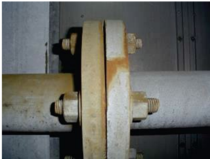
Figure 76. Photo. Gap in splice connection.
