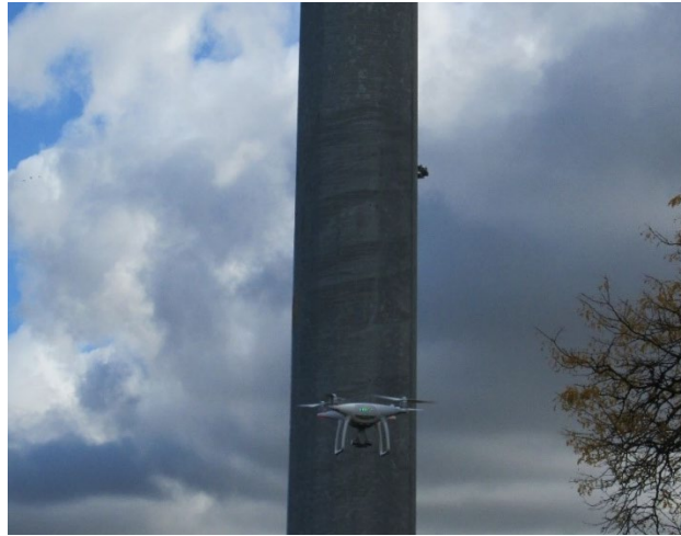
Figure 58. Photo. UAS mobilized on a high mast light pole.
