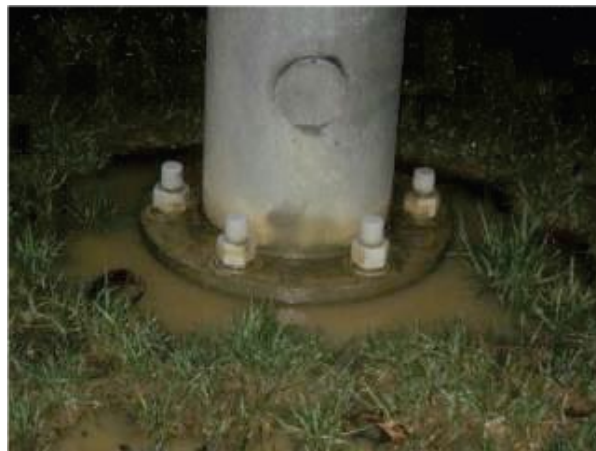
Figure 69. Photo. Foundation with grading sloped towards foundation.
