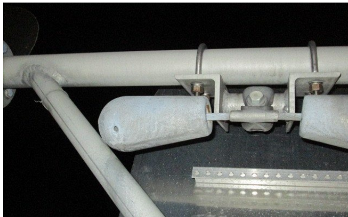
Figure 106. Photo. Damper on aluminum span. Left weight is in contact with the diagonal member.
