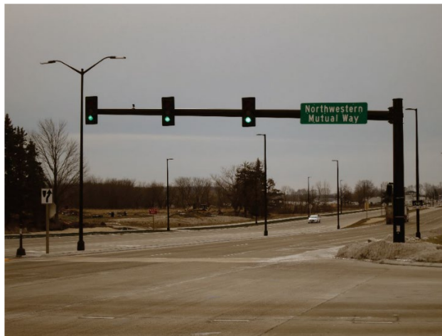
Figure 11. Photo. Single mast arm.
