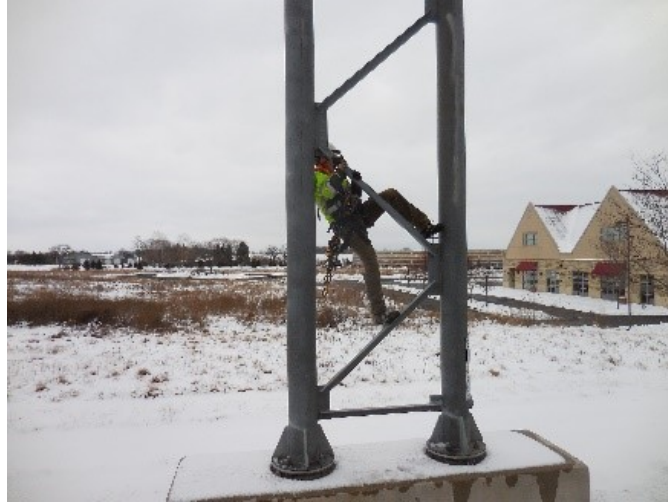
Figure 36. Photo. Dual post with framing members.
