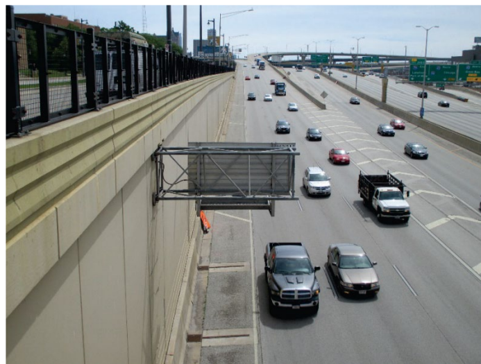
Figure 23. Photo. Retaining wall mounted structure.
