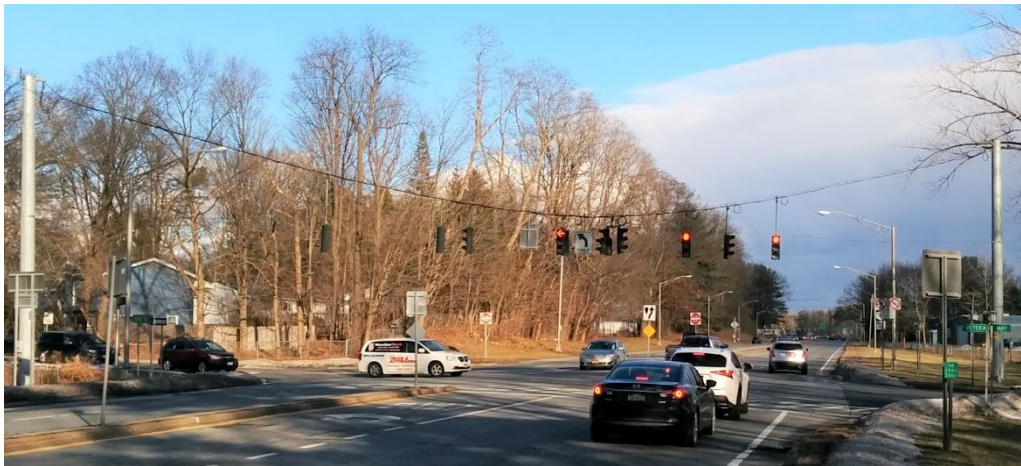
Figure 17. Photo. Span wire structure.
