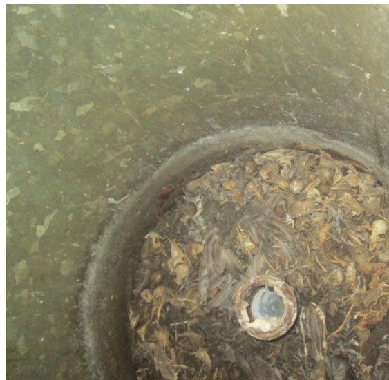
Figure 95. Photo. Accumulated bird remains inside an end support post.
