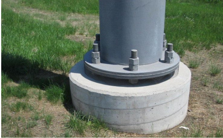
Figure 25. Photo. Drilled shaft footing.
