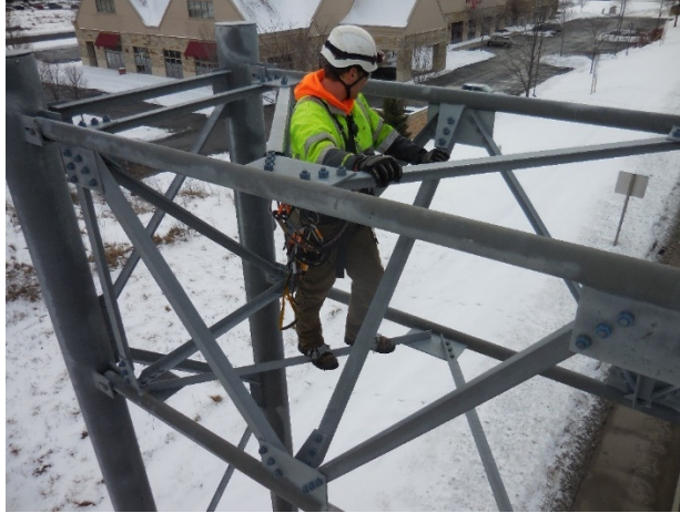
Figure 49. Photo. Common inspector safety equipment.
