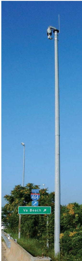
Figure 18. Photo. Camera pole structure.
