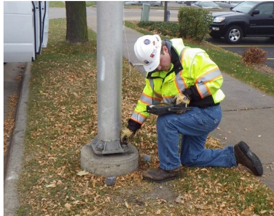
Figure 86. Photo. Inspector utilizing ultrasonic testing equipment.
