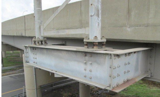
Figure 27. Photo. Structure attached to bridge fascia girder.
