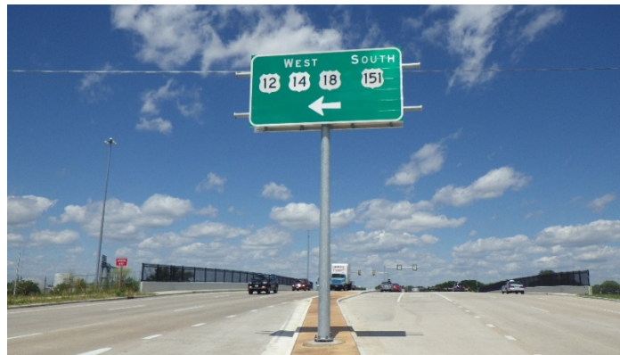
Figure 15. Photo. Untrussed, two-chord butterfly.
