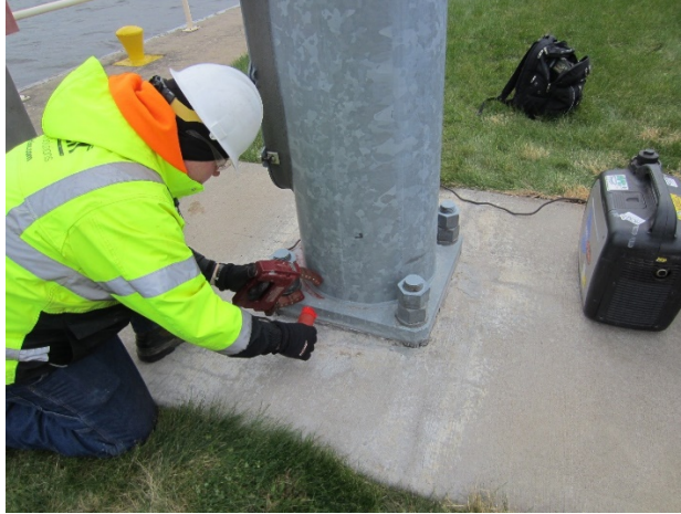
Figure 84. Photo. Inspector using Magnetic Particle Testing equipment.
