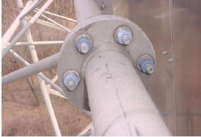
Figure 45. Photo. Aluminum span splice connection.
