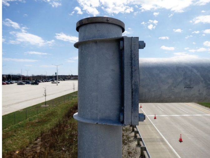
Figure 44. Photo. Mast arm bolted connection.
