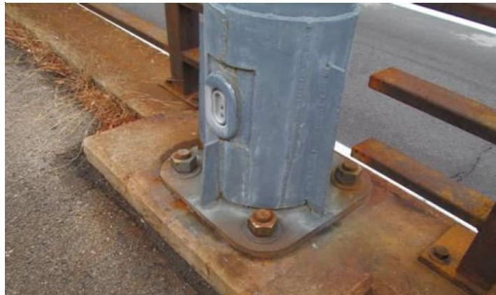
Figure 98. Photo. Plating repair of a vertical end support column.
