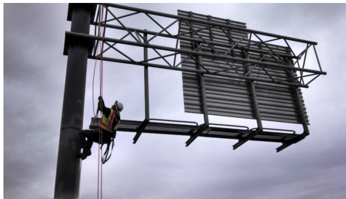
Figure 50. Photo. Inspector climbing using rope access equipment.
