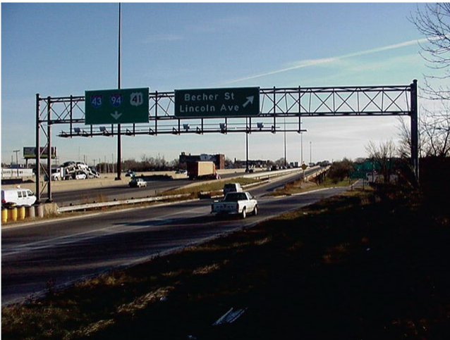
Figure 2. Photo. Four-chord full span.
