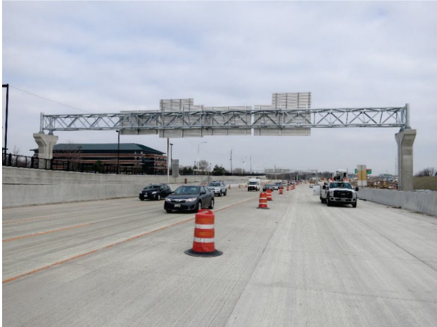
Figure 1. Photo. Four-chord full span.
