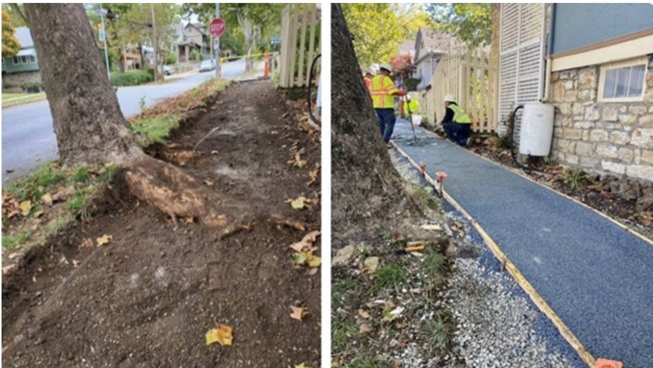
Figure 1: Before and after rubberized sidewalk implementation. (Source: City of Kansas City)
