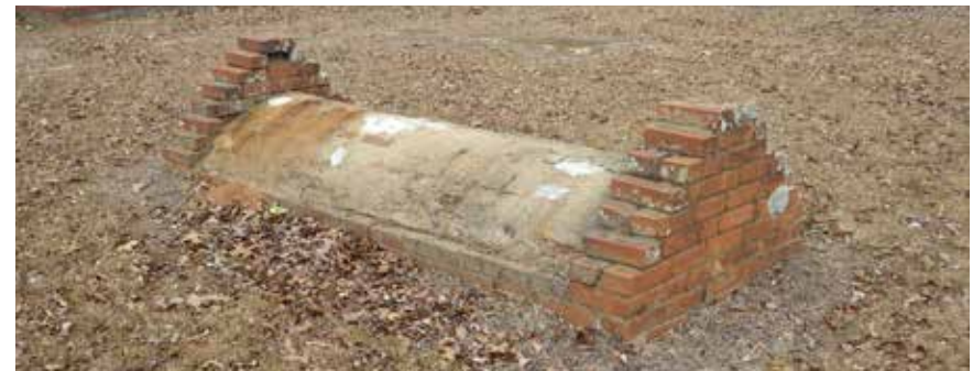
Brick Barrel Vault. The brick work is contiguous with, or a separate brickwork component from the underlying vault. Tabernacle Methodist Church Cemetery, Washington County.
