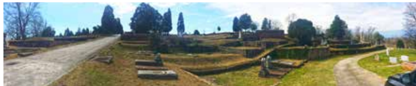
To make the most of interesting terrain, retaining walls and terraces were used to provide flat locations for burials, Rose Hill Cemetery, Bibb County.
