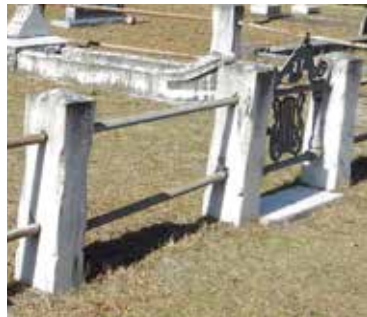
Gas Pipe with Lyre, Oak Grove Cemetery, Camden County.
