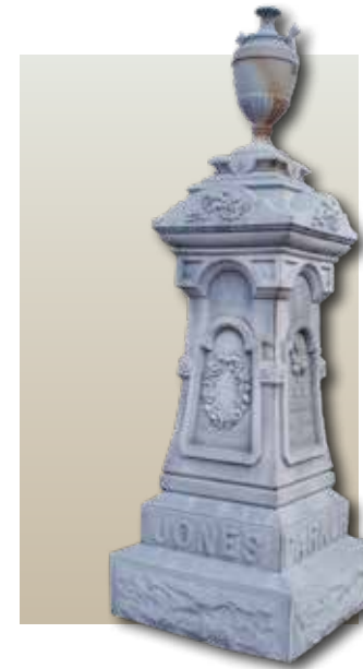
Complex decorative designs can be cast into zinc, making it an ideal medium for monument production. Cedar Hill, Terrell County.
