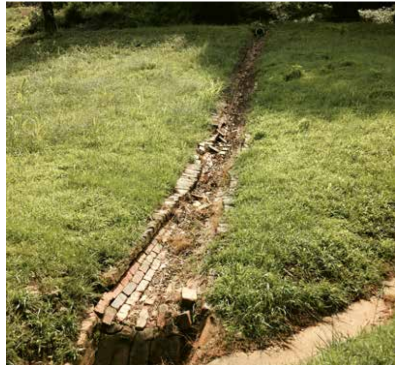
Original Brick Stormwater Gutter, Myrtle Hill Cemetery, Floyd County.
