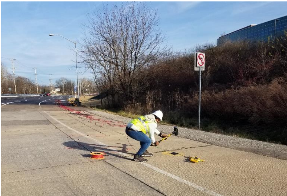
Figure 4.11. Seismic shots for post-grouting seismic data acquisition efforts.
