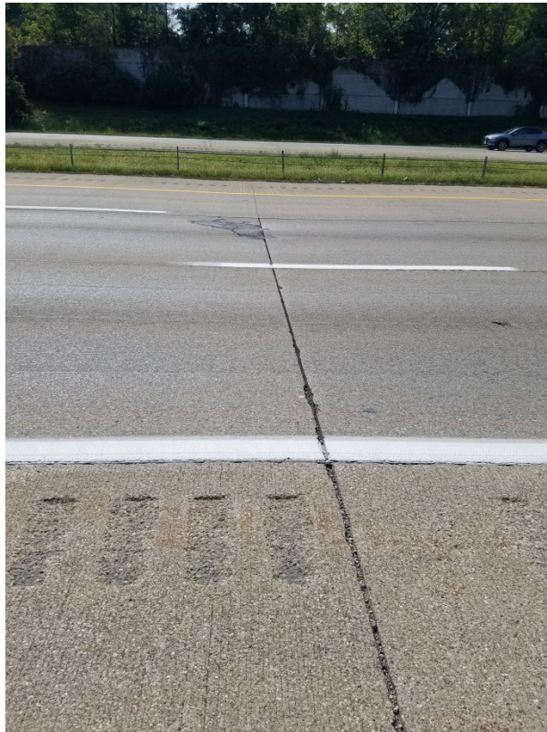
Figure 3.6 Corner Break on HAM-275-36.58
