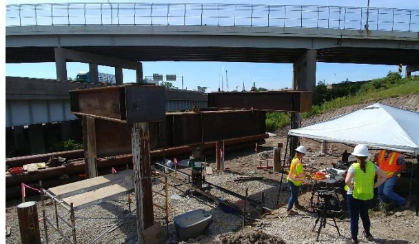
Static load test at LUC-75 Site
