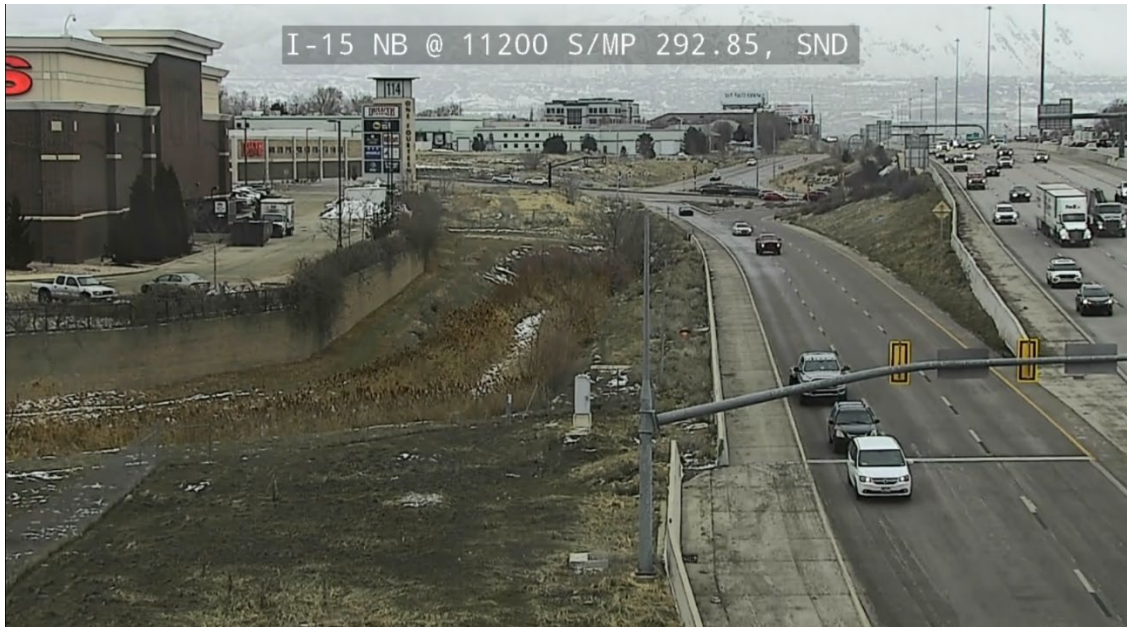
Figure 3.3 Sample Frame at 11400 South Bound Ramp at I-15 Highway
