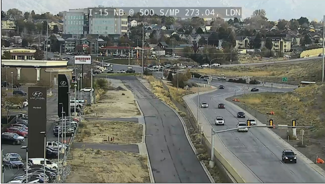
Figure 3.2 Sample Frame at 500 South Bound Ramp at I-15 Highway
