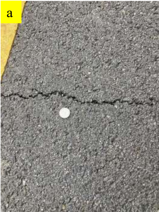
Figure D.14 Pictures taken of cracks on Bussey Road a) Reflection crack, b) longitudinal crack
