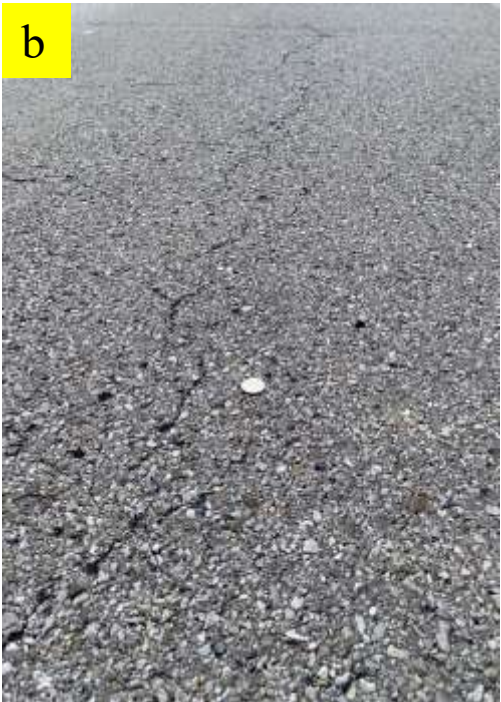
Figure D.14 Pictures taken of cracks on Bussey Road a) Reflection crack, b) longitudinal crack
