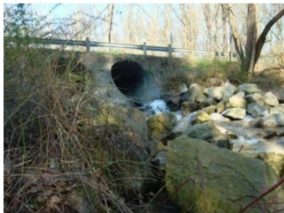
Figure 36: Unnamed tributary to East Branch at RM 15.35 is impaired by a perched culvert that acts as a fish barrier.
