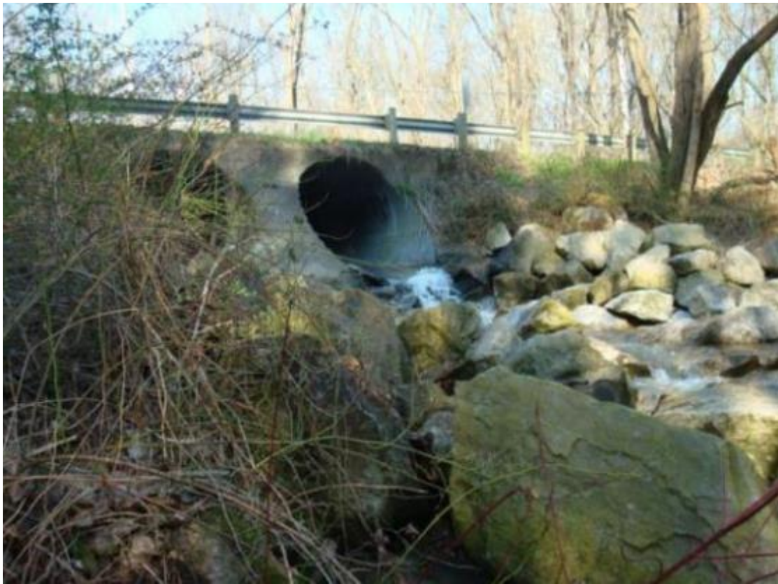
Figure 4 Perched culvert at Sperry Road Bridge. Photo Source: Chagrin River Watershed Partners – East Branch Chagrin.
