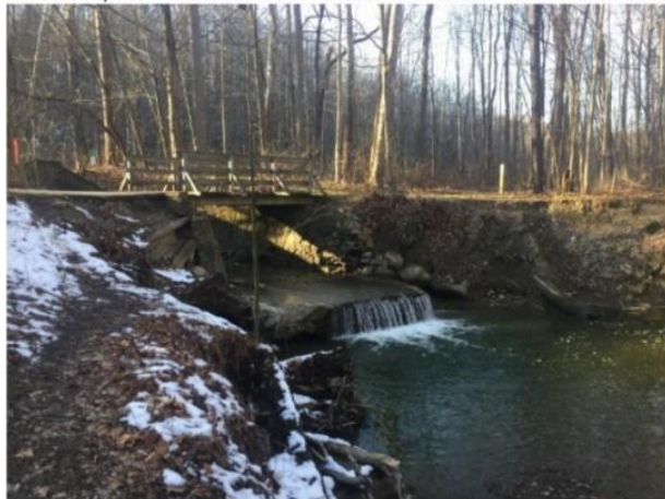
Figure 24: Drop structure acting as fish migration barrier at Beecher's Brook near Wilson Mills trailhead at North Chagrin Reservation
