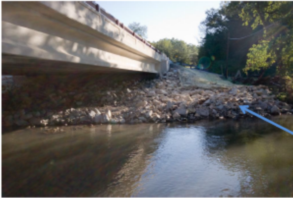
(TH30 Bucksnot Bridge, Fillmore County MN)
