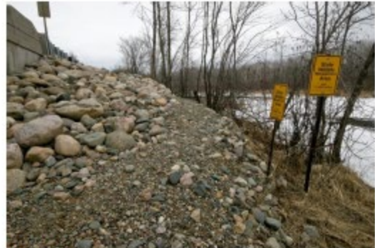
Figure 5. Bench must connect to surrounding topography
