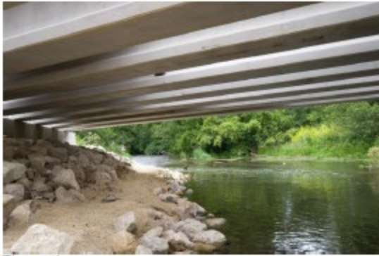
Figure 1. Completed Passage Bench
