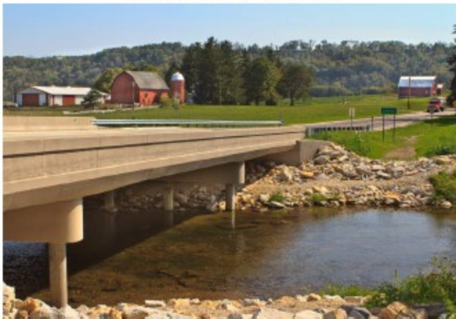
(TH43 Choice Bridge, Fillmore County)
