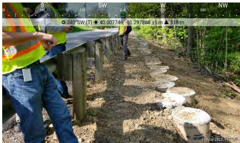
(a) Recent remediation
