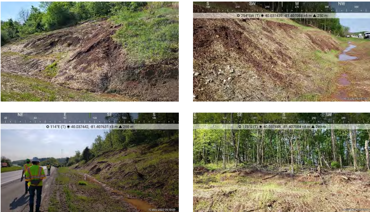
Figure 1 Photos from site visit for site LS00006904 (GUE-70-18.747).
