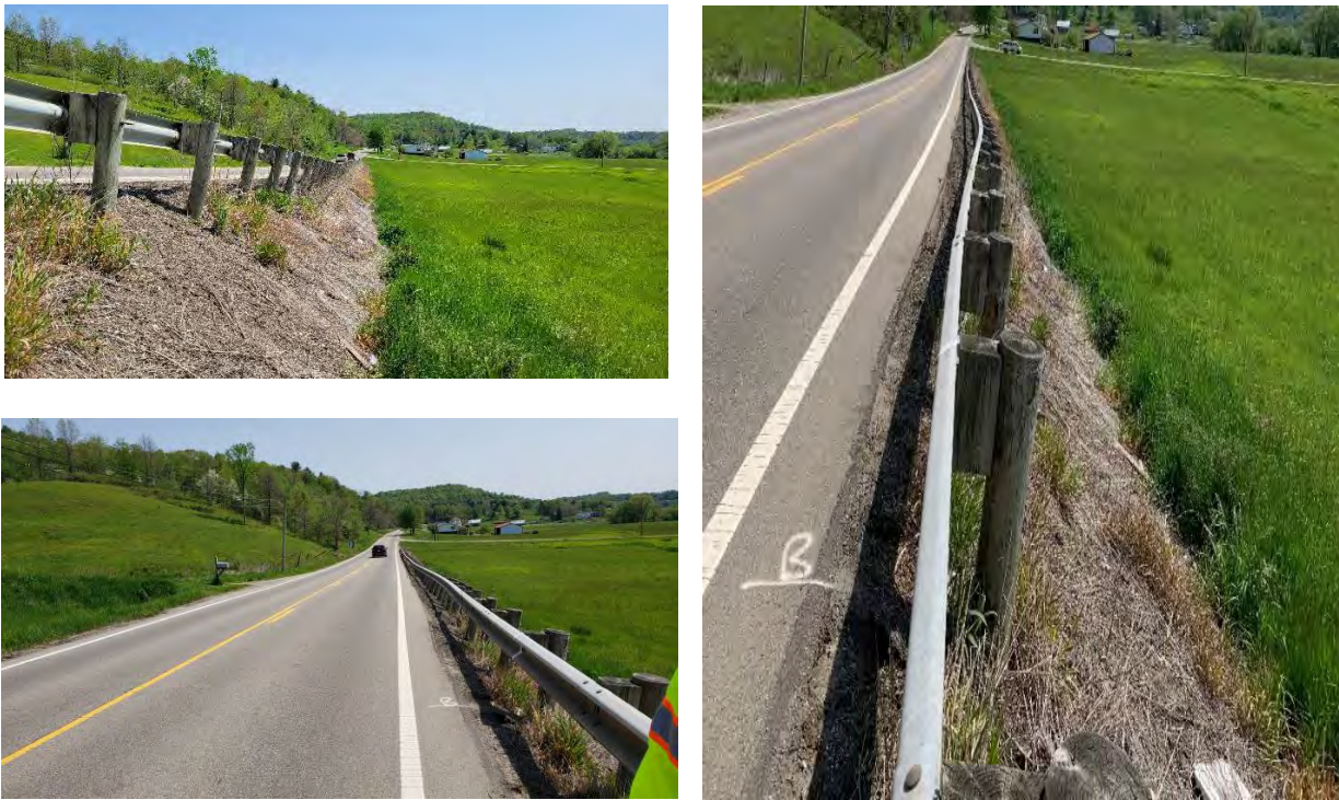
Figure 6 Photos of site visit for site LS00008439 (GUE-265-14.935)
