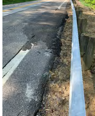
Figure 4 Photos of site visit for site LS00008440 showing bending in guard rails and crack in the pavement.
