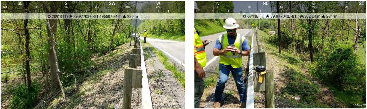
Figure 8 Photos of site visit for LS0000636 (BEL-147-3.434).
