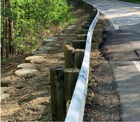
Figure 4 Photos of site visit for site LS00008440 showing bending in guard rails and crack in the pavement.
