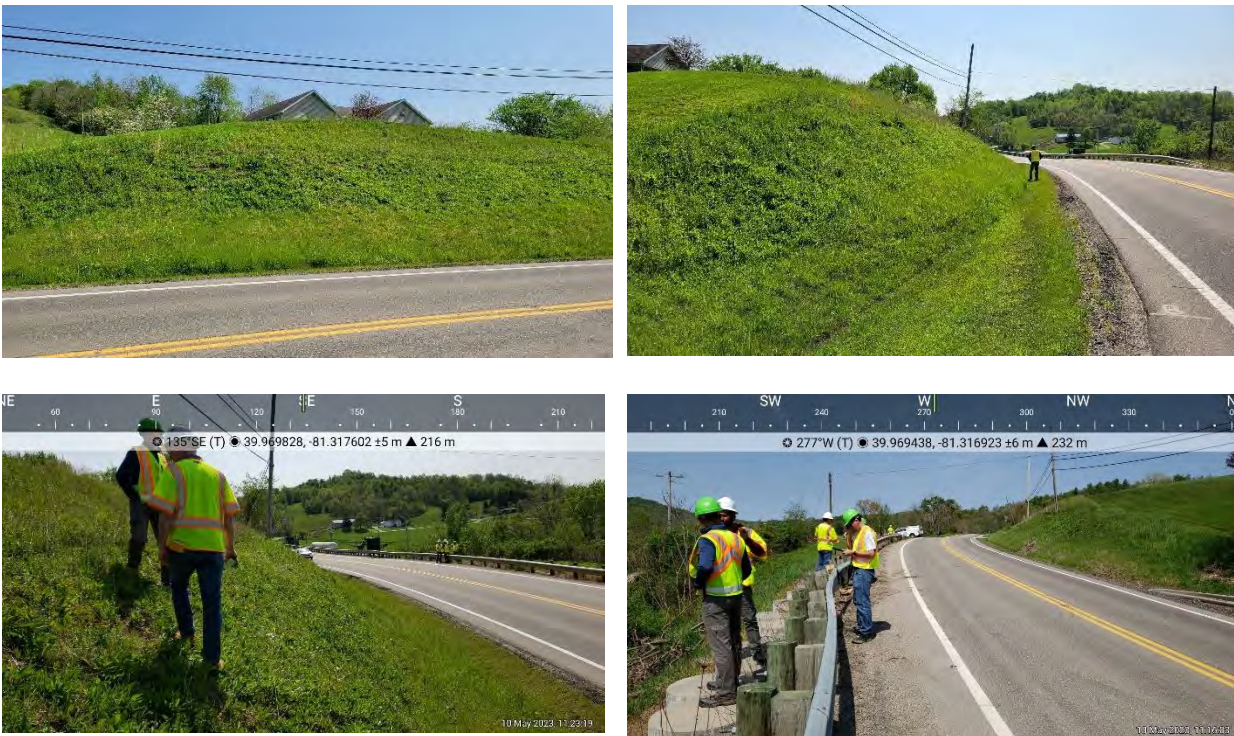
Figure 5 Photos of site visit for site LS00006794 (GUE-265-12.788).
