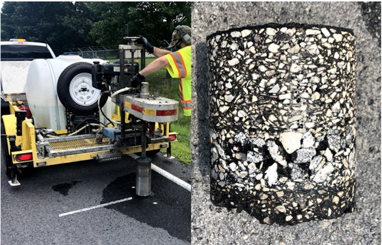
Figure 10. Photo. Coring operation (left); picture of a typical core (right).
