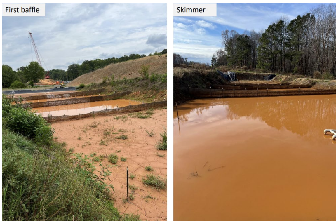
Figure 12. Basin 6 at the end (December 2022) of sample collection. (Left) Looking at the first baffle (first chamber), and (Right) looking at the skimmer (last chamber).
