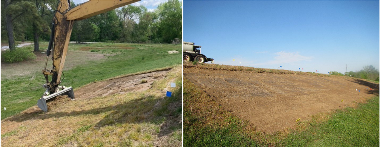
Figure 37. Location of plot in the Kingsboro Industrial Area. The existing vegetation was scraped off before installing the treatments.
