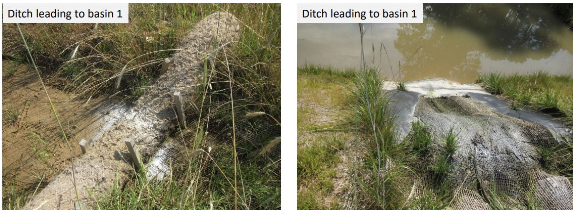
Figure 18. Polyacrylamide (PAM) application on wattles leading to basin 1.
