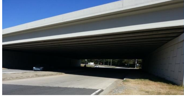
(b) Culvert tunnel
