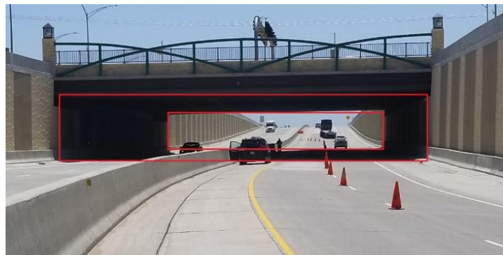
Figure 23. Illustration. Black frame due to the visibility of the exit portal in the approaching drivers' view.
