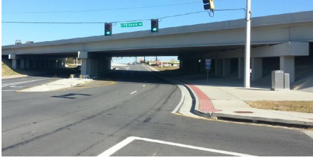
(a) Span tunnel with median piers
