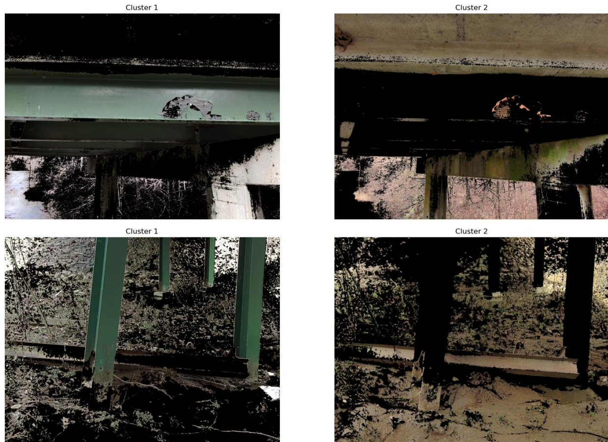
Figure 18. Photographs. Results of color thresholding in the L*ab color space.
