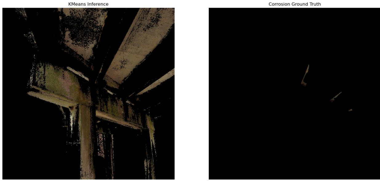
Figure 23. Photographs. K-means segmentation on an image with a small amount of corrosion.
