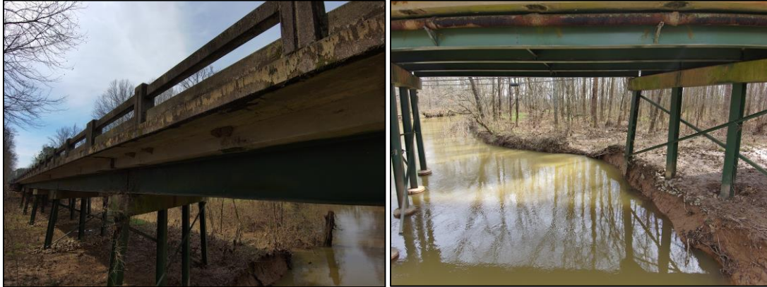
Figure 6. Photographs. Bridge over Salacoa Creek, Calhoun.
