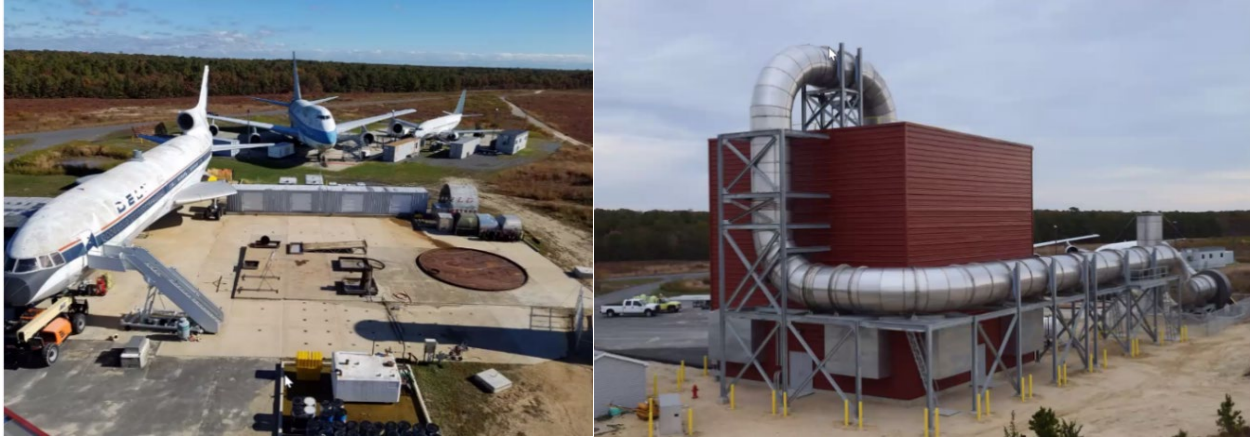
Figure 14. ARFF and Aircraft Safety Test Areas (Left) and ARFF Research Facility (Right)
