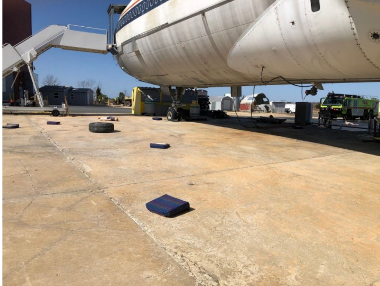
Figure 16. Ground View of ACY Debris
