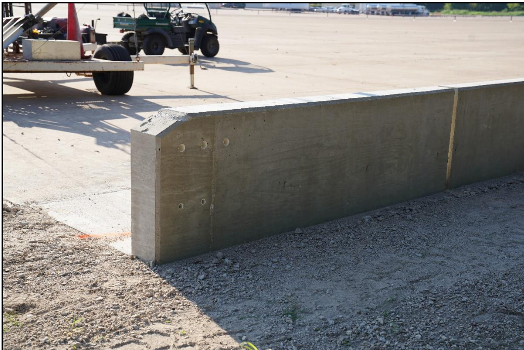
Figure 6.5. Field Side of the Concrete Parapet Shape Transition prior to Testing 611801-03-1&2.
