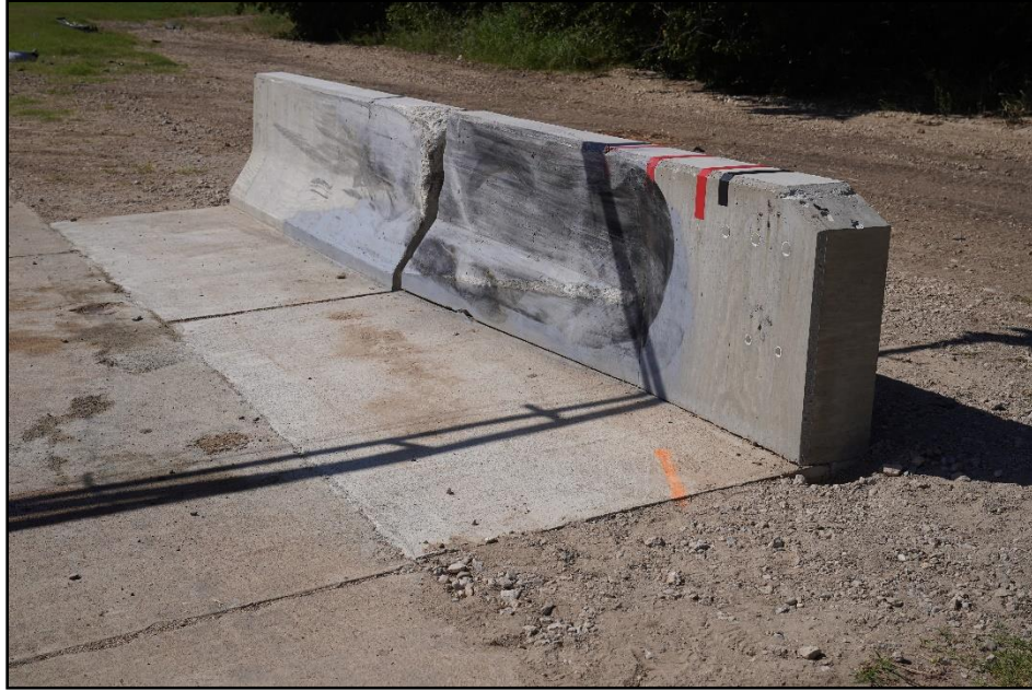
Figure 6.21. Concrete Parapet Shape Transition after Test at Impact Location 611801-03-2.
