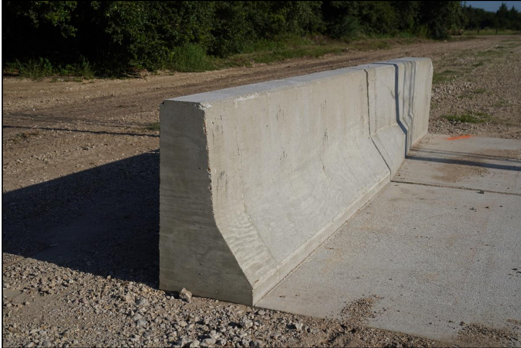
Figure 6.4. End View of the Concrete Parapet Shape Transition Prior to Testing 611801-03-1&2.
