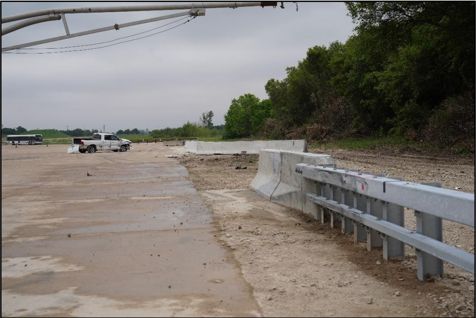
Figure 7.22. Overall View of the Box Beam to Concrete Barrier Transition after Test 611801-04-2.
