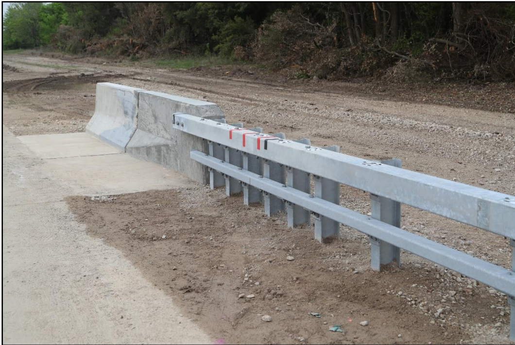
Figure 7.2. Box Beam Guardrail Transition to Concrete Parapet prior to Testing 611801-04-1&2.
