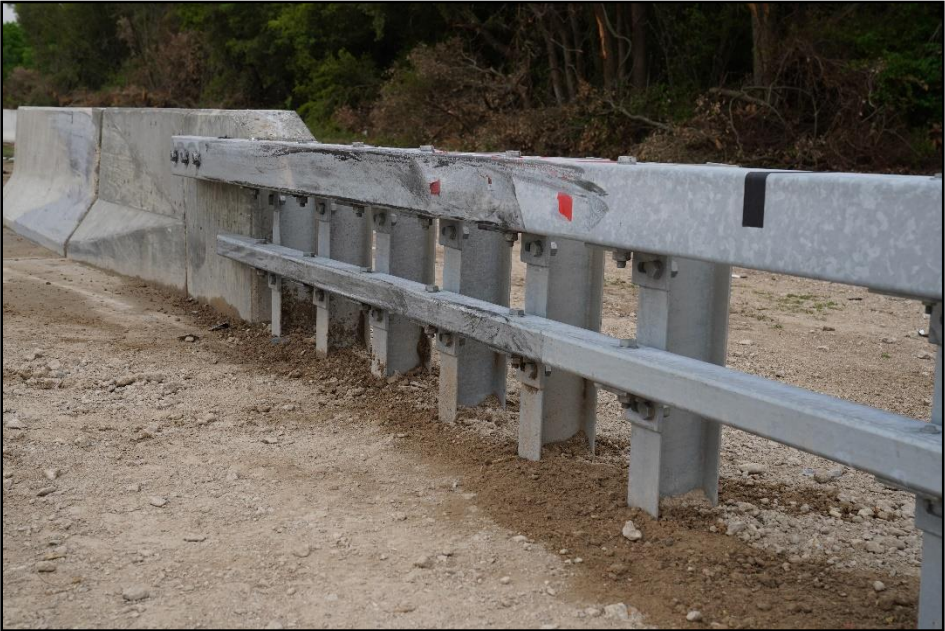
Figure 7.21. Box Beam to Concrete Barrier Transition at Impact Location after Test 611801-04-2.
