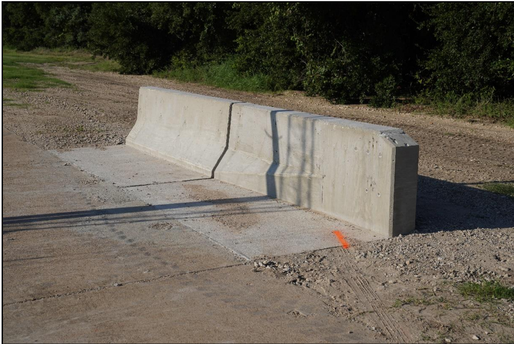
Figure 6.2. Concrete Parapet Shape Transition prior to Testing 611801-03-1&2.
