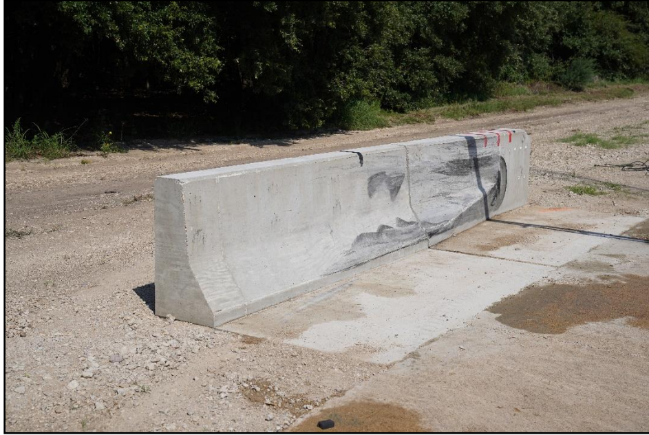
Figure 6.10. Concrete Parapet Shape Transition after Test at Impact Location 611801-03-1.
