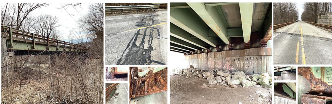
Figure 2.1 Photographs of Case Study #1: steel bridge.
