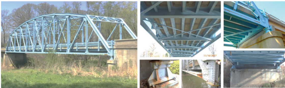
Figure 4.4 Photographs of the alternative bridge for Case Study #1.
