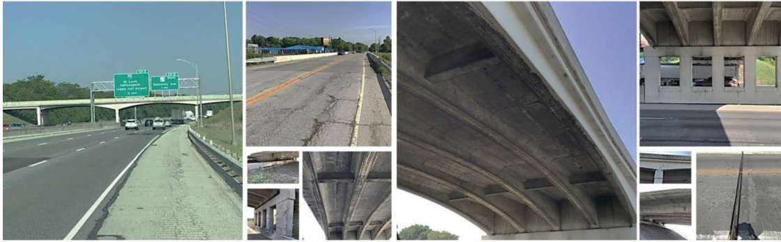
Figure 2.2 Photographs of Case Study #2: concrete bridge.
