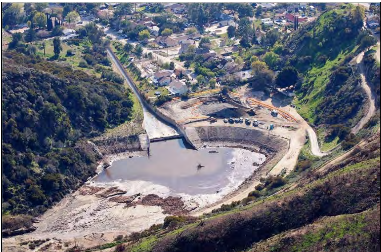
Figure 7.7. Debris basin. Source: Los Angeles County Department of Public Works.
