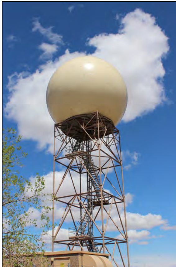
Figure 6.9. Typical NWS NEXRAD radar dome. Source: NWS.
