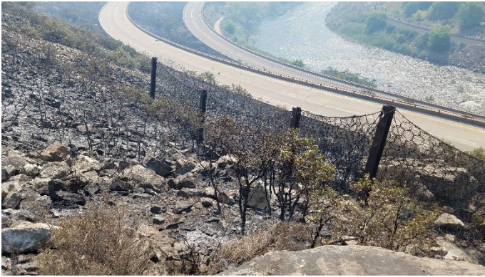
Rockfall fencing. Source: FHWA
