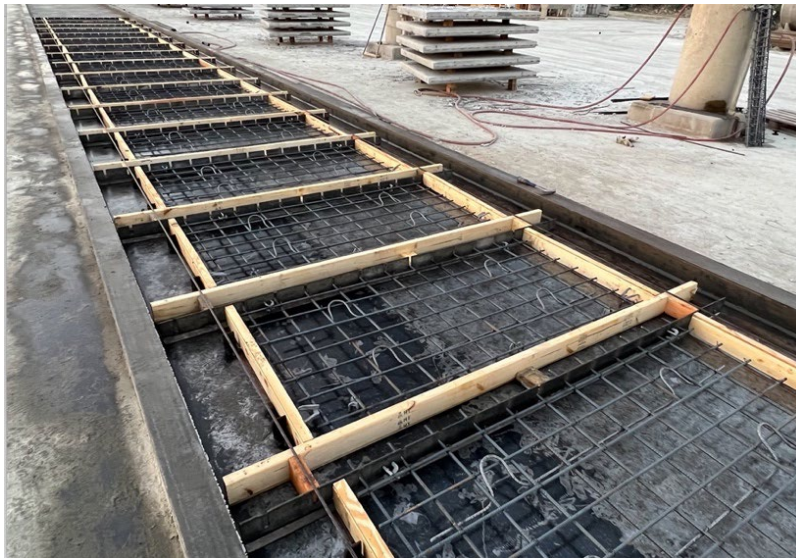
Figure 8.17 – Formwork and Reinforcing for PCPs
