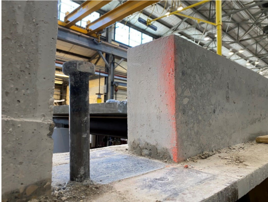
Figure 8.103 – Beam Specimen No. 2 – Section Cut Through Slab Near Shear Stud
