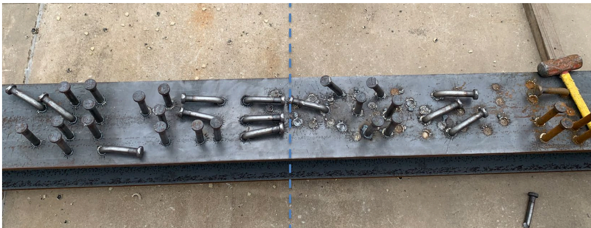
Figure 4.41 - 1-1/8" Studs Welded Using 2150A, 1.4s, S Polarity (right side of photo) and R Polarity (left side of photo) on W14×132 Girder. Some Studs on the Left are Welded Without Cable Looping and Surface Preparation.
