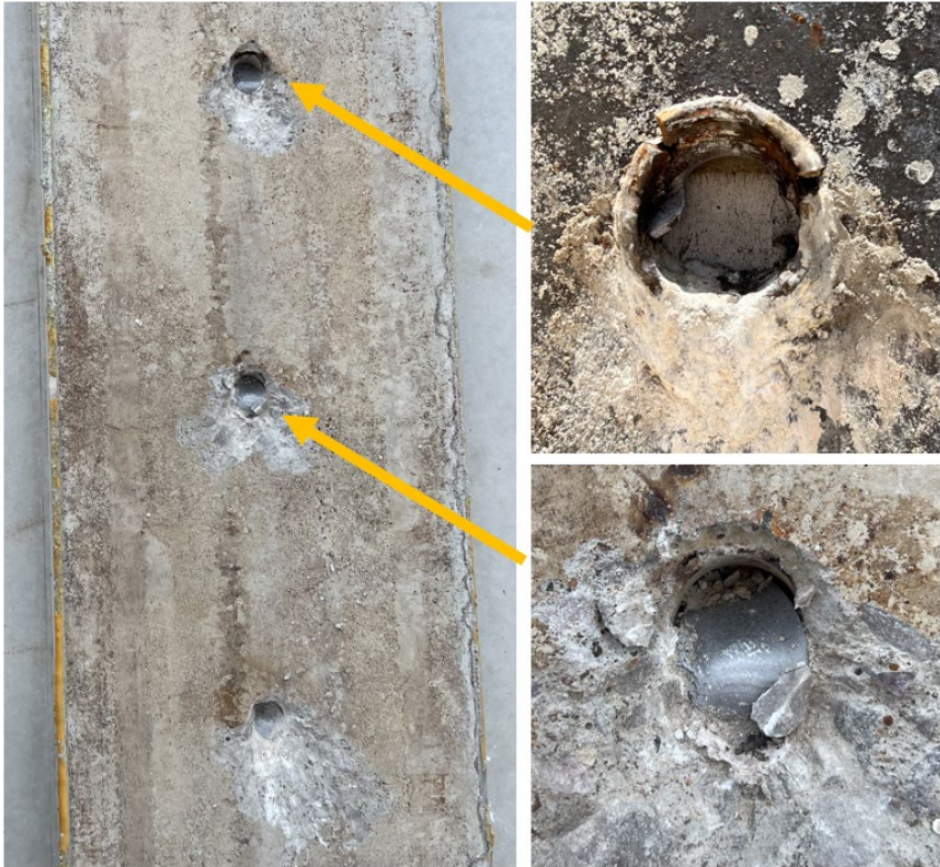
Figure 6.5 - Specimen No.2F: Concrete Deck After Failure with Enlarged Photos of Studs
