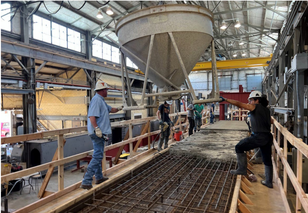
Figure 8.45 – Concrete Placement for Beam Specimen No. 1
