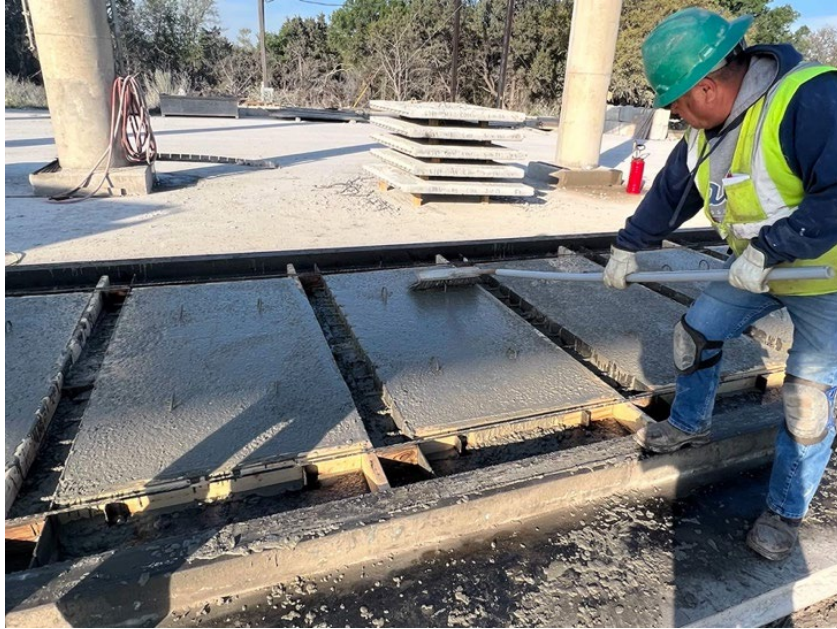
Figure 8.18 – Broom Finishing of Top Surface of PCPs
