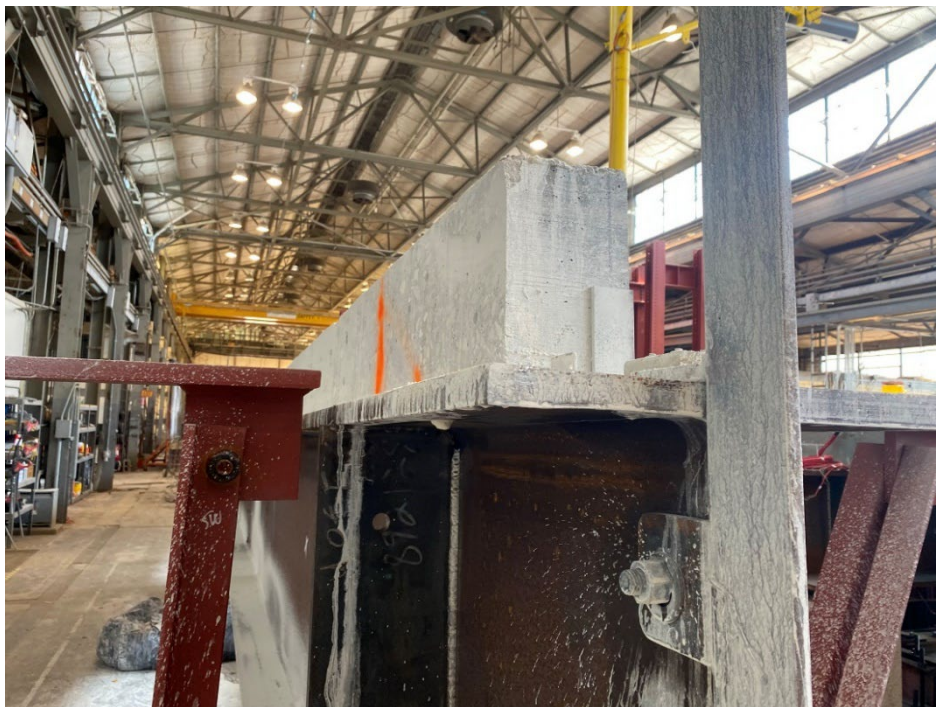
Figure 8.104 – Beam Specimen No. 2 – Section of Slab Cut Near End of Beam
