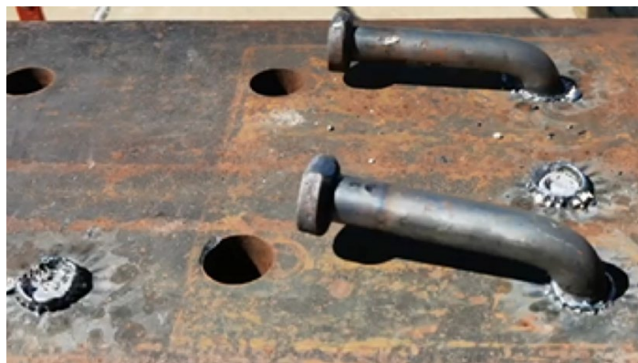
Figure 4.42 - 1-1/8" Studs Welded Using 2150A, 1.4s, R Polarity, No Surface Preparation, No Cable Looping on a W14×500 Girder with 3-1/2" Thick Flange. 90° Bend Test Results
