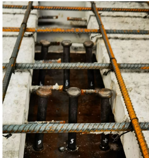
Figure 5.8 - Shear Studs Bent Inward in Specimen No. 2
