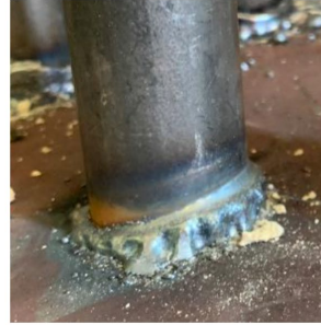
Figure 4.6 - Weld Collar Under Arc Blow Effect (Illustration on the Left: ISO 2017b)
