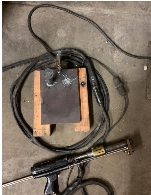
Figure 4.7 - Cable Looping Around the Welding Point
