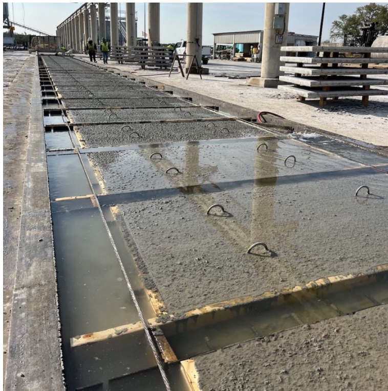
Figure 8.19 – Finished PCP Panels
