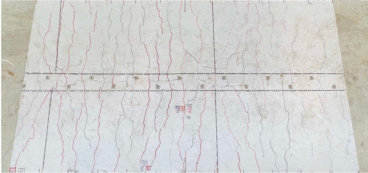
Figure 8.94 - Beam Specimen No. 2 - Crack Distribution After Completion of Two-Span Test and Boundaries of the PCPs
