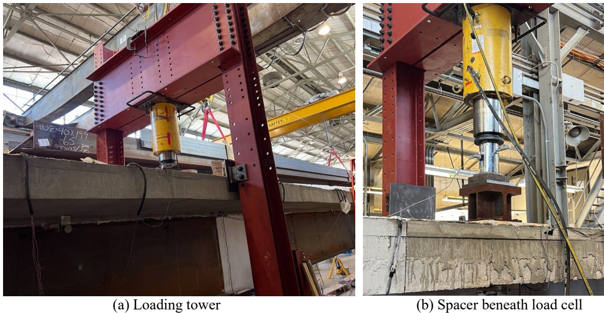
Figure 8.21 – Photos of Loading Tower
