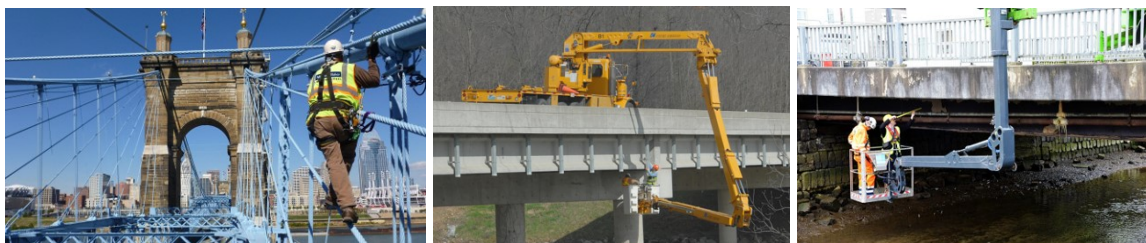
Figure 1. Sample Images of Bridge Inspections Conducted by Specialists (Cho, 2018)
